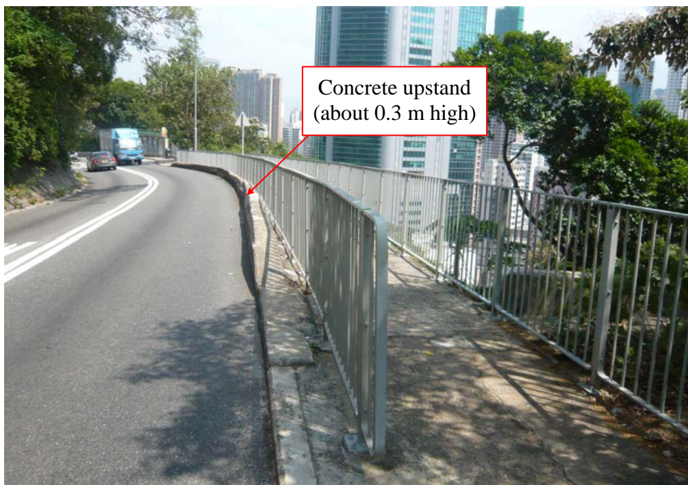
Plate 14 - Concrete Upstand along Stubbs Road above the 7 June 2008 Landslide (Photograph taken on 23 September 2009)
