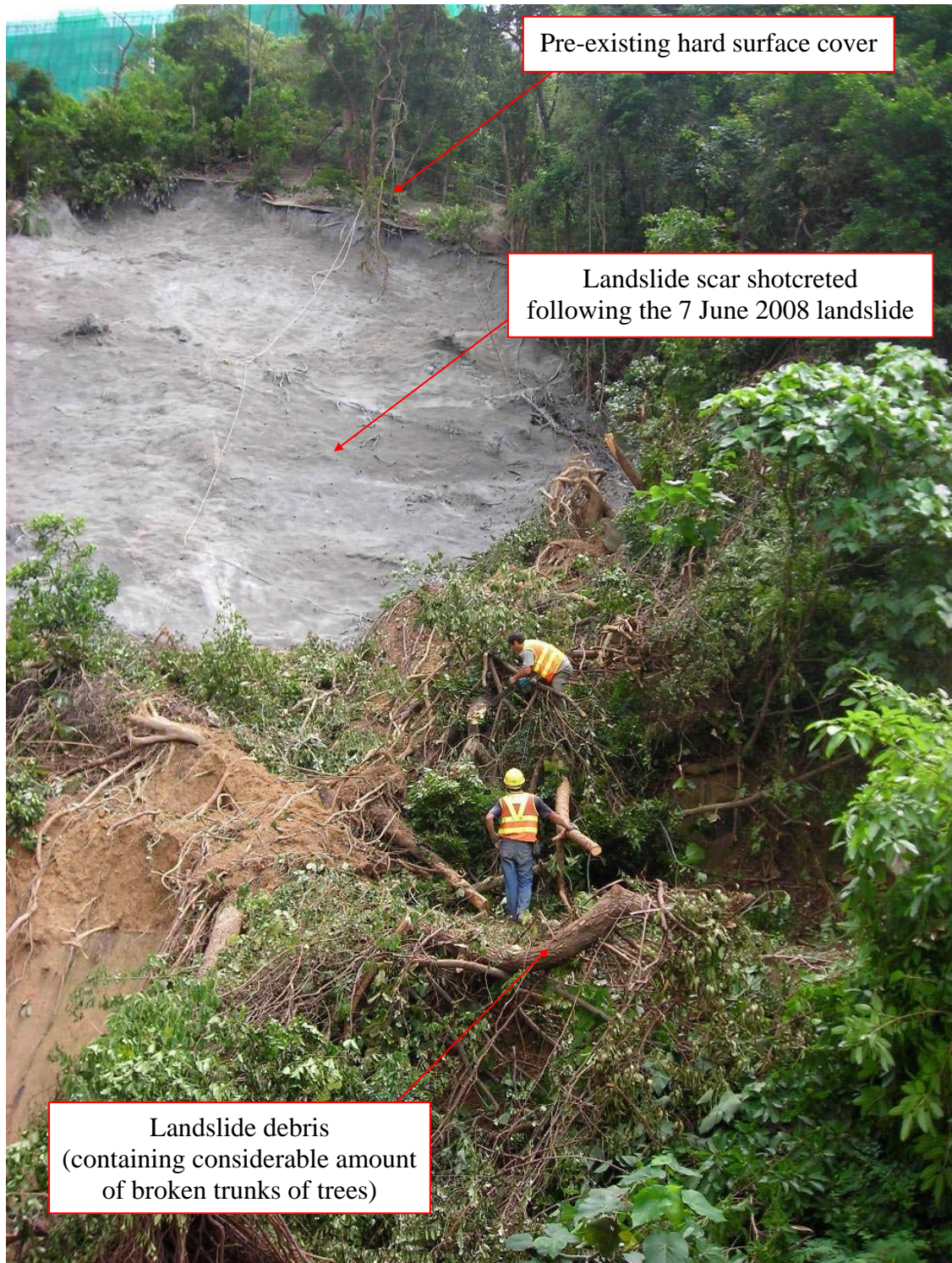
Plate 6 - Landslide Debris Deposited on the Cut Slopes at the Toe of Hillside (Photograph taken on 10 June 2008)
