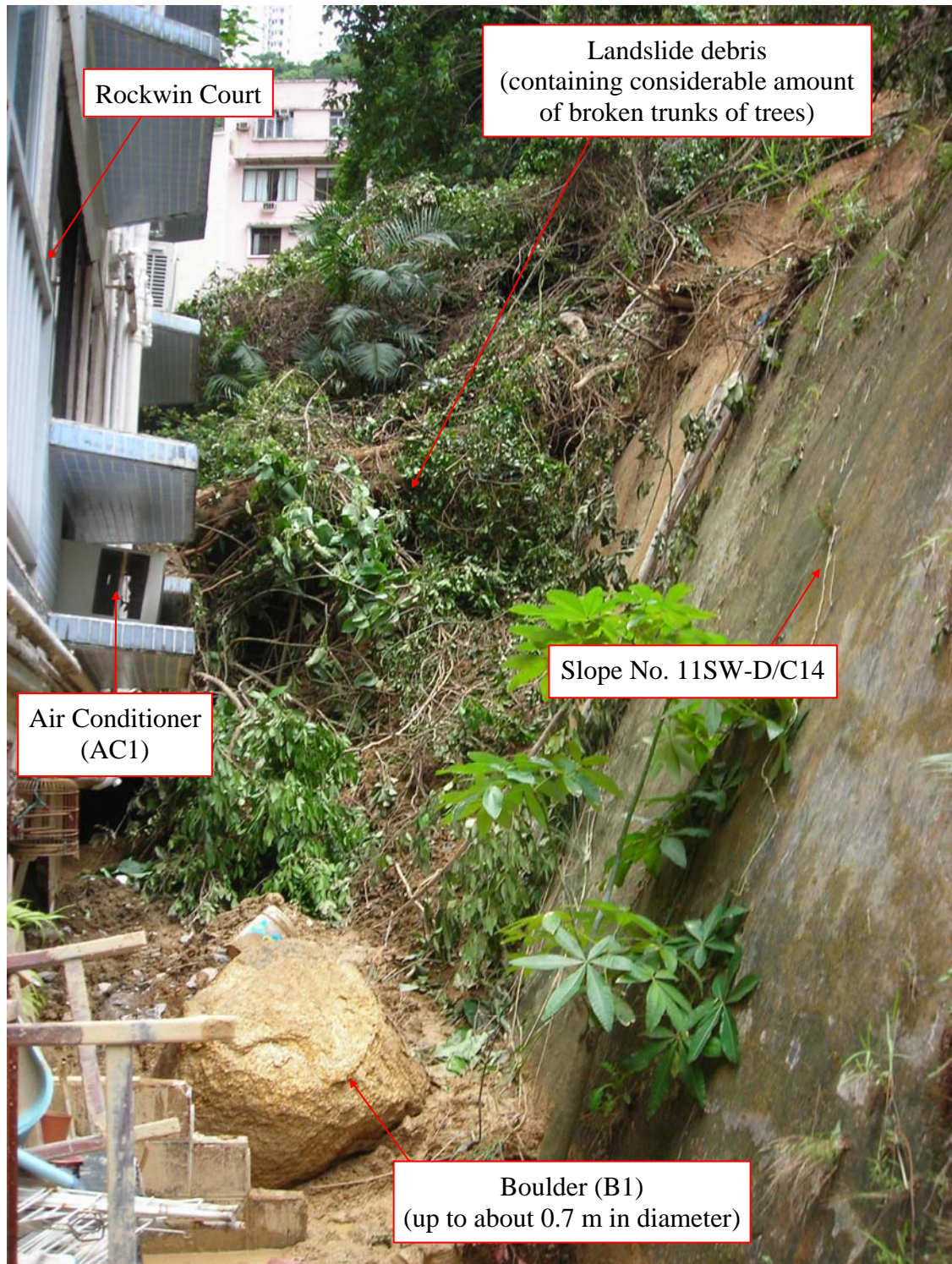
Plate 7 - Landslide Debris Deposited at the Rear of Rockwin Court (Photograph taken on 10 June 2008)
