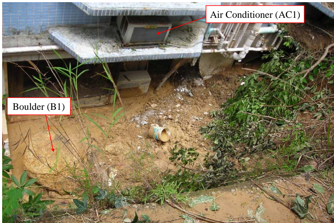
Plate 8 - Landslide Debris Piled against Rockwin Court (Photograph taken on 10 June 2008)
