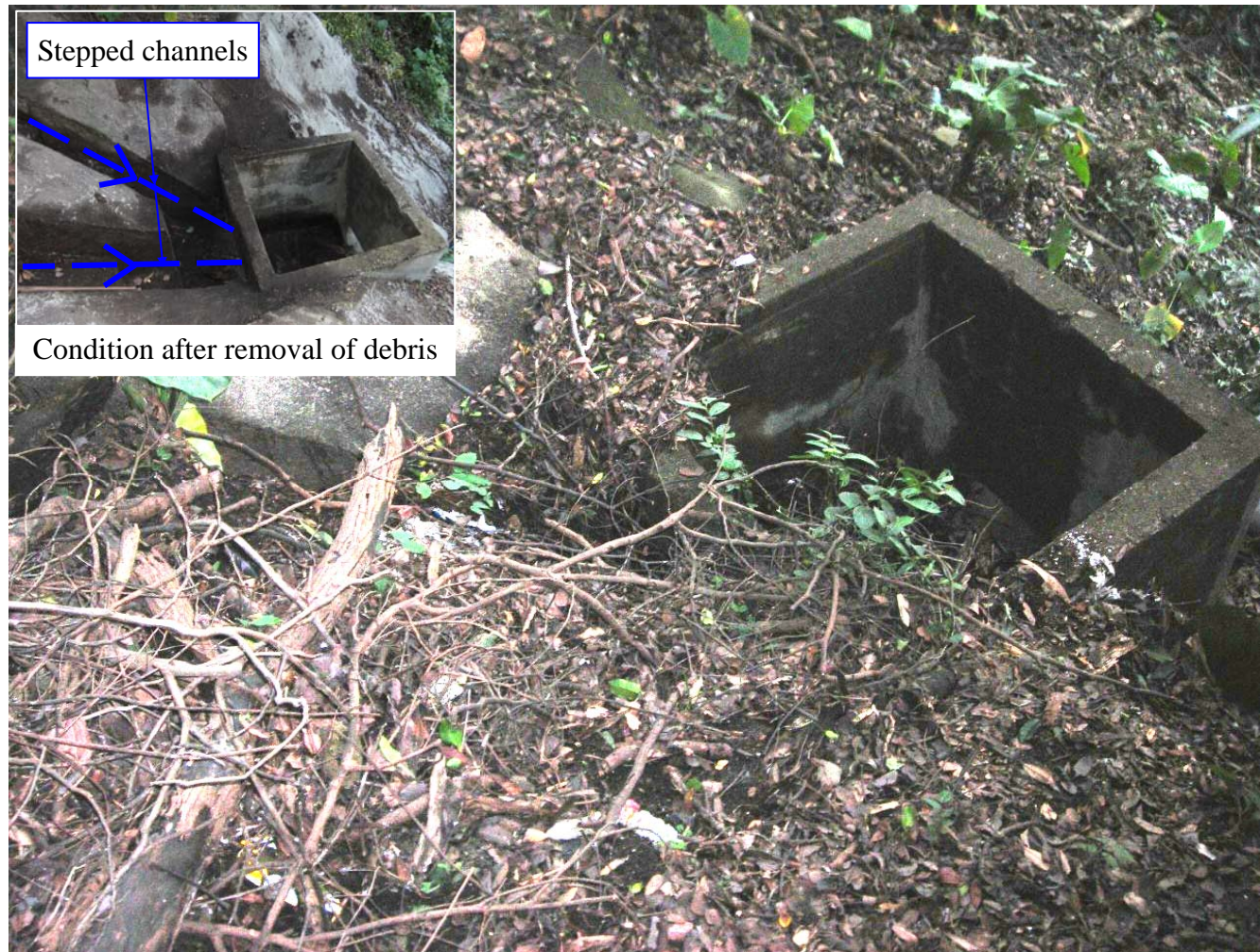
Plate 11 - Blocked Stepped Channels at the Northern Flank of the 7 June 2008 Landslide (Photograph taken on 10 June 2008)
