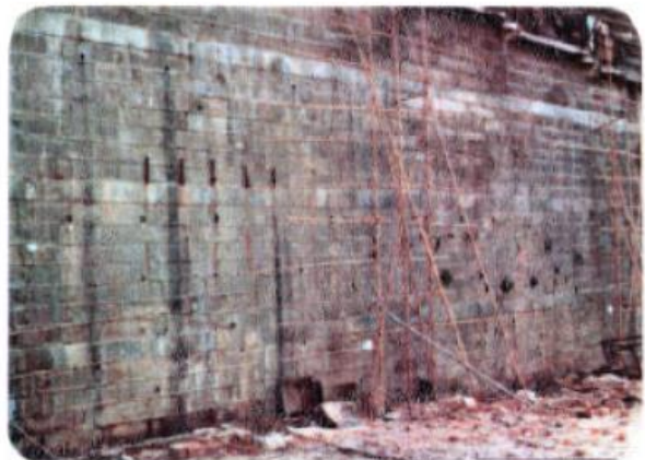
Tied Face Wall with Horizontal Beams (11SW-A/R45)
