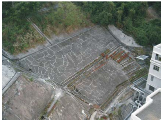
Example F12 Extensive Cracking of Hard Cover
