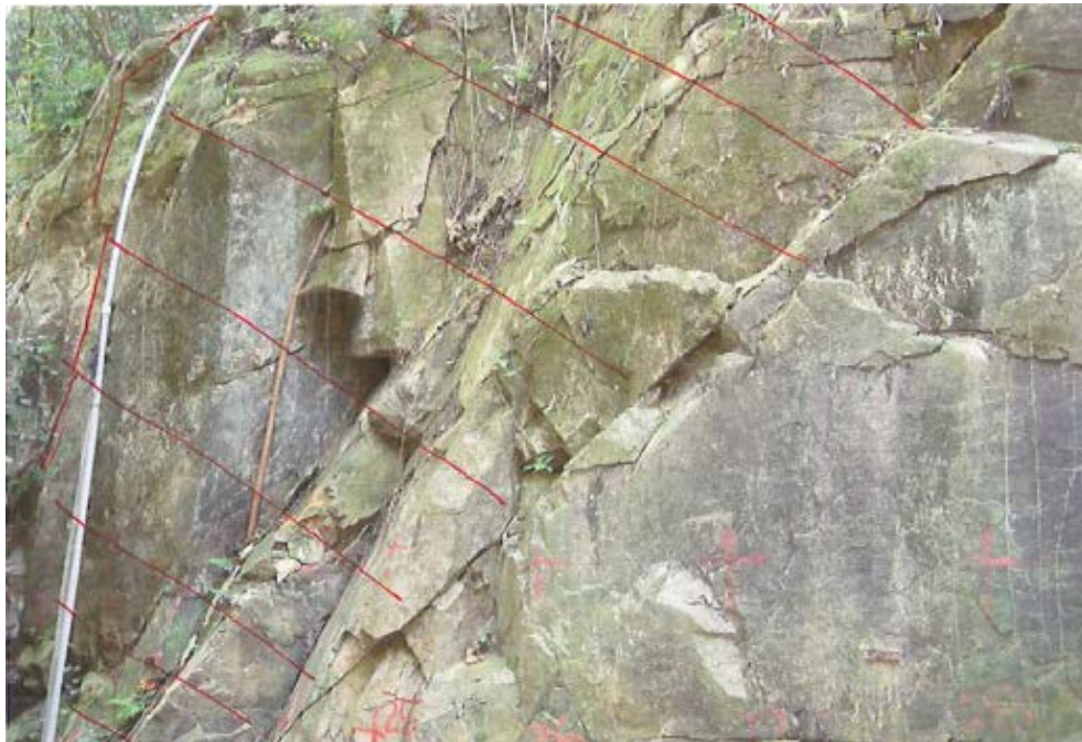
V2 Potential Wedge Failure of the Rock Mass
