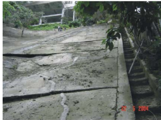
Example F14 Subsidence and Extensive Cracking of Hard Cover
