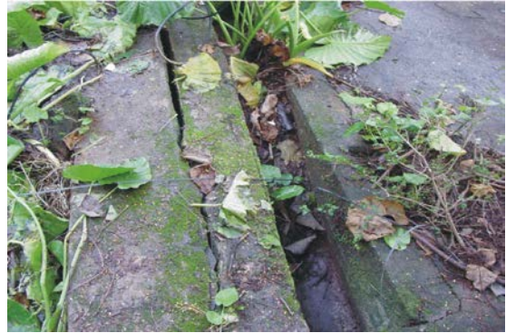
Example F8 Detached Surface Channel
