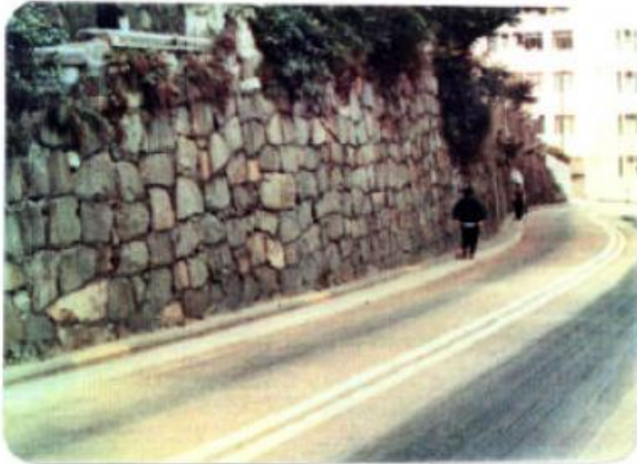
Dry Packed Random Rubble Wall (11SW-A/R389)
