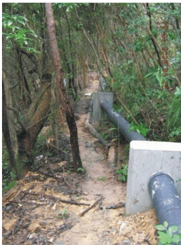
Example F5 Displaced Pipeline
