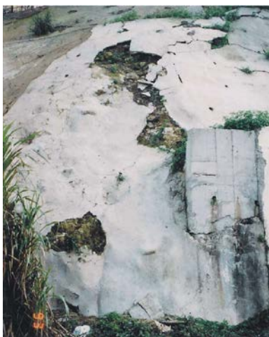
Example F11 Cracking of Hard Cover
