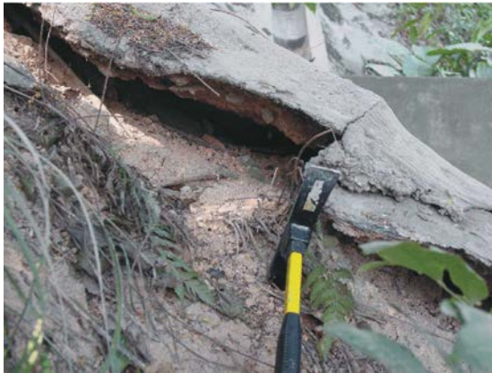
Example F13 Voids Underneath Hard Cover
