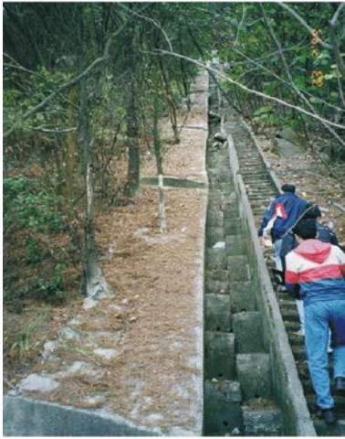
Example F1 Displaced Surface Channel
