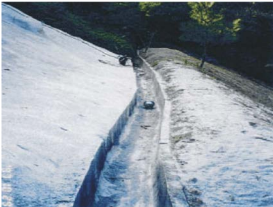
Example F3 Displaced U-channel
