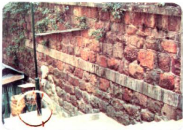
Pointed Squared Rubble Wall with Horizontal Beams (11SW-A/R194)
