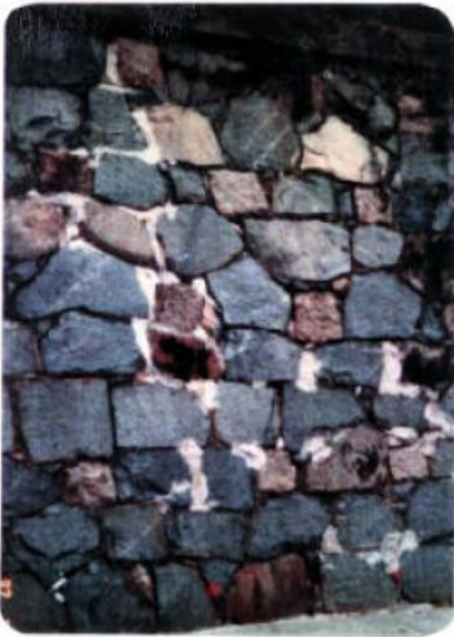
Random Rubble Wall with Stone Ties
