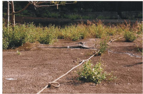
Example F4 Cracking and Bulging of Hard Cover
