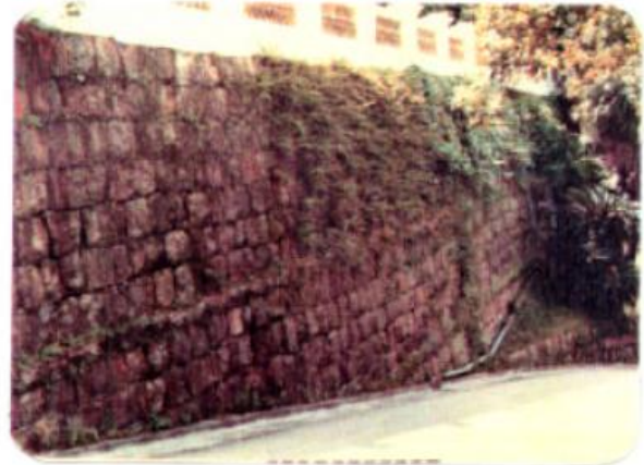
Dry Packed Squared Rubble Wall with Horizontal Beams (11SW-A/R163)
