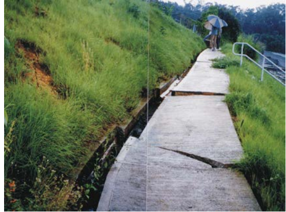
Example F2 Cracking of Berm
