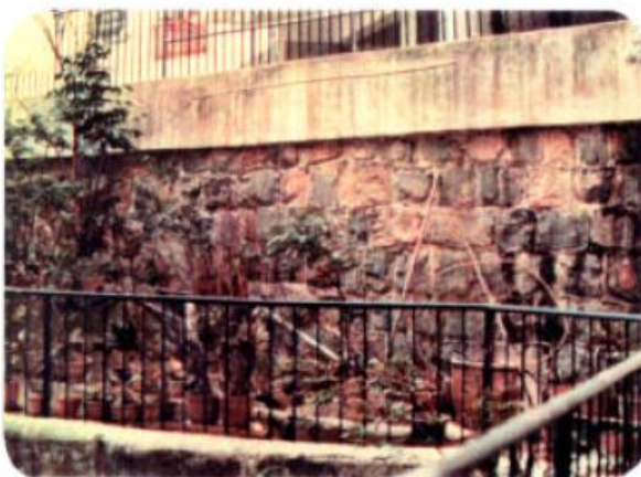
Pointed Squared Rubble Wall (11SW-A/R295)
