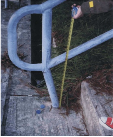
Example F7 Deformed Railings
