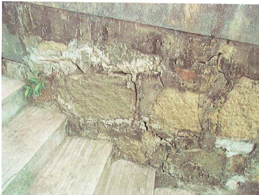
V2 Crack and Missing Pointings
