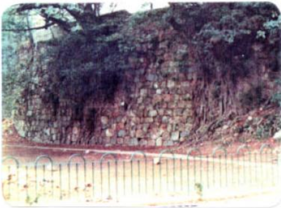
Dry Packed Squared Rubble Wall (11SW-A/R109)
