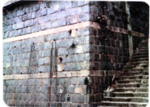
Dressed Block Wall with Horizontal Beams (11SW-A/R423)
