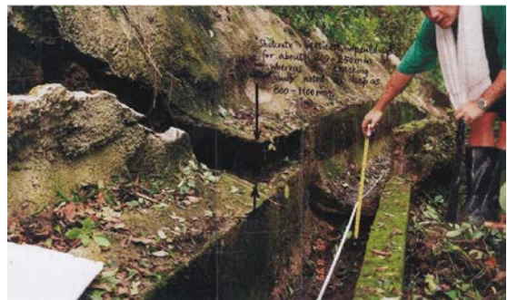
Example F6 Displaced Surface Channel
