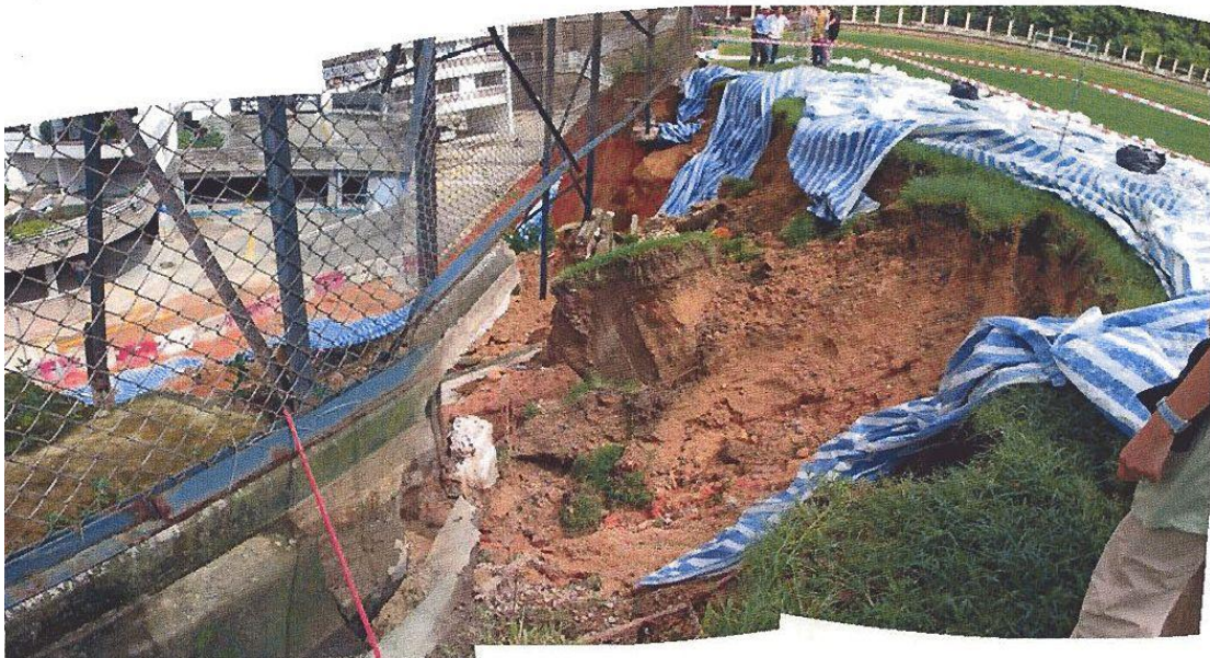
Plate 2 – View of the Landslide Scar Extending into the Grassed Sports Ground above Slope No. 11NW-D/C144 (Photograph taken by GEO on 22 August 2005)
