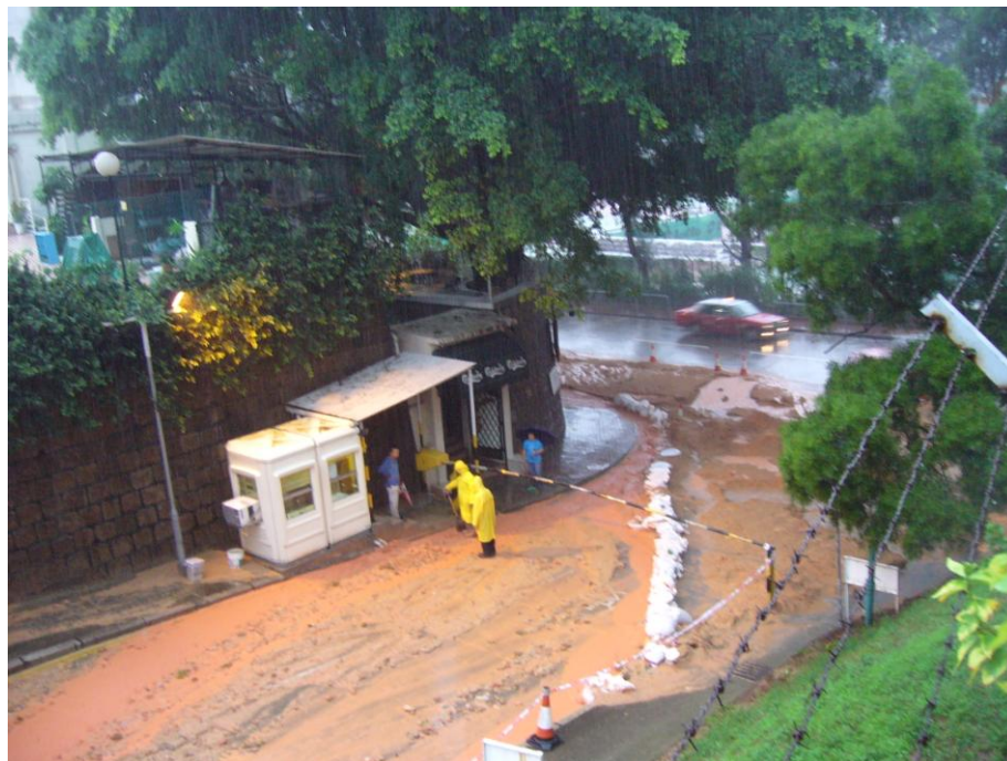
Plate 6 – Landslide Debris Deposited on the Entrance of the Access Road at Wylie Road (Photograph taken by MGSL on 20 August 2005)
