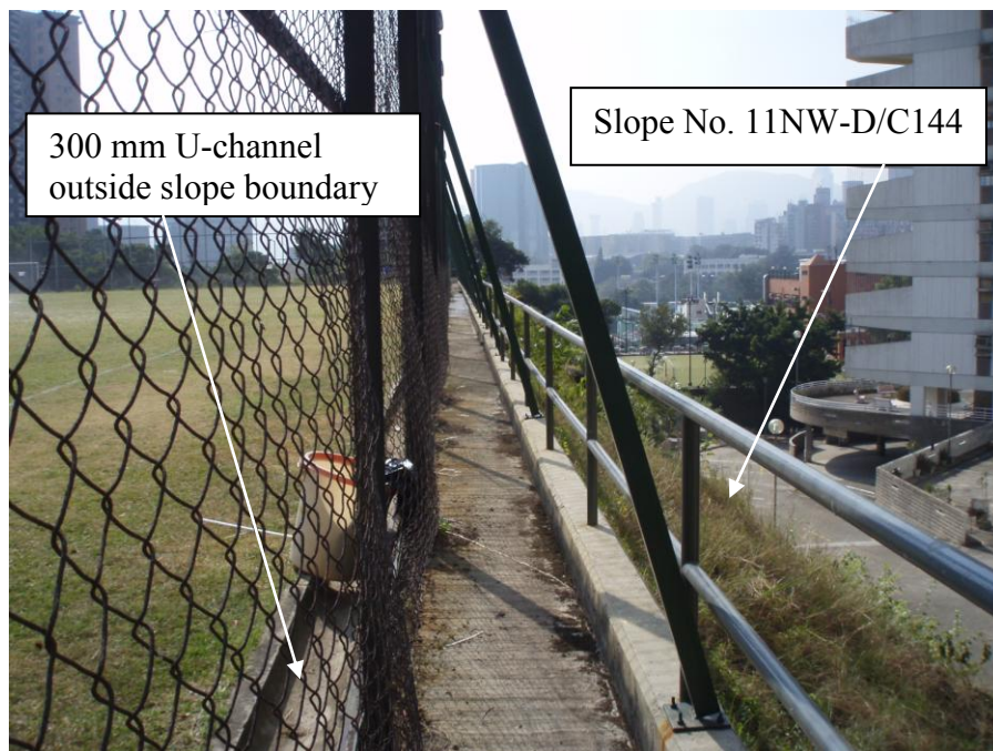
Plate 10 – Crest Condition of Slope No. 11NW-D/C144 after LPM Works (Photograph taken by HCL on 12 November 2007)
