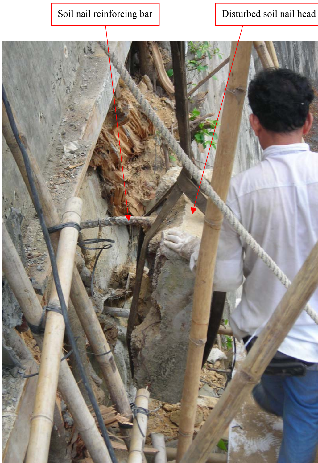
Plate 10 – Close View of Disturbed Soil Nail Head (Photograph taken on 4 September 2006)
