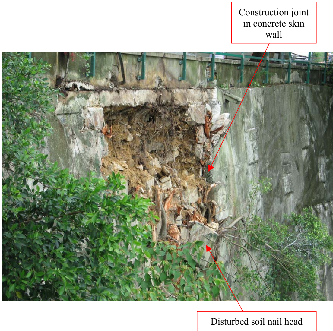
Plate 5 – Close View of Scar Associated with the 3 August 2006 Landslide Incident (Photograph taken by GEO on 4 August 2006)
