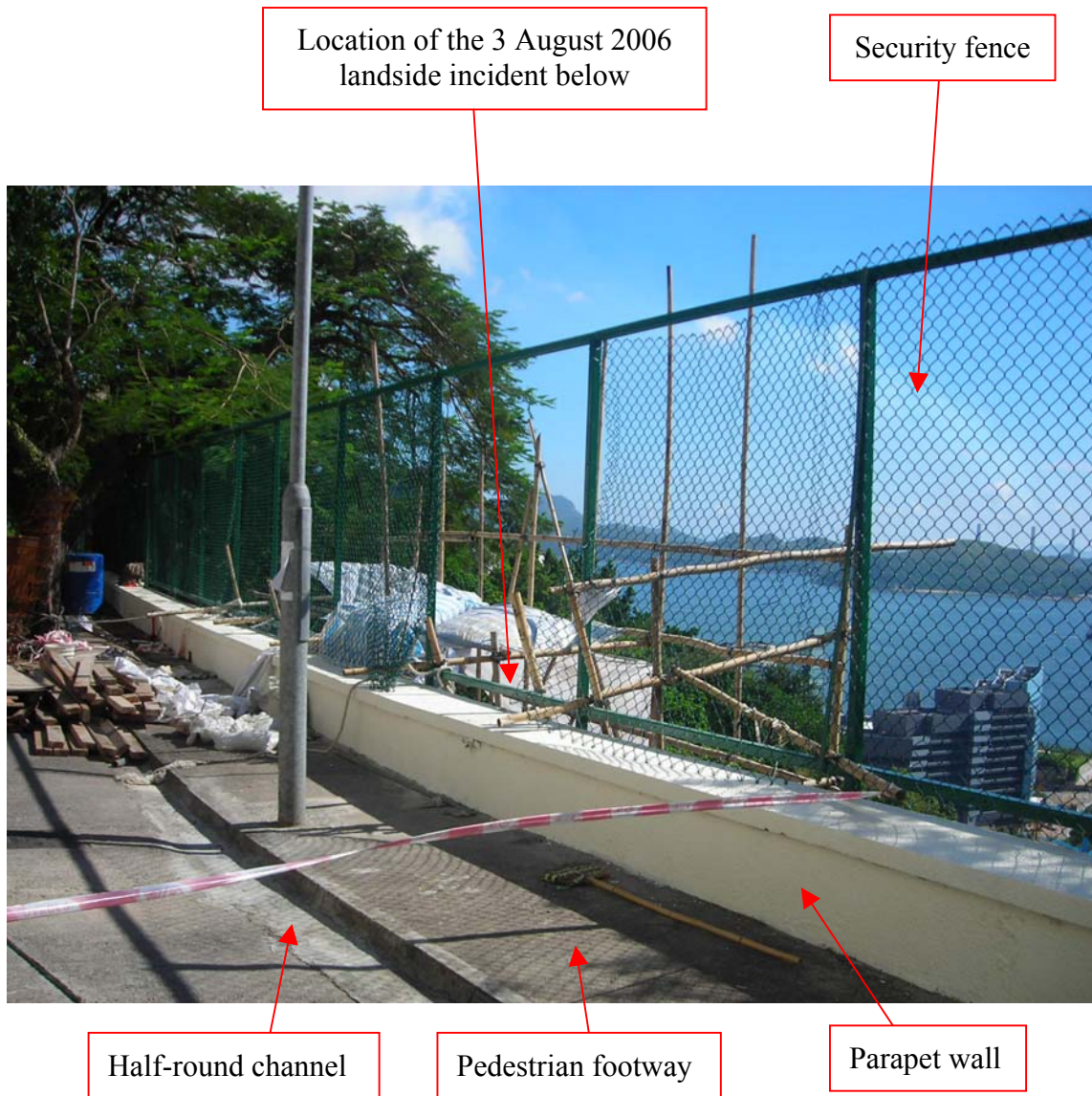
Plate 3 – General View of Crest Area of Slope No. 11SW-C/FR319 above Location of the 3 August 2006 Landslide Incident (Photograph taken on 30 August 2006)
