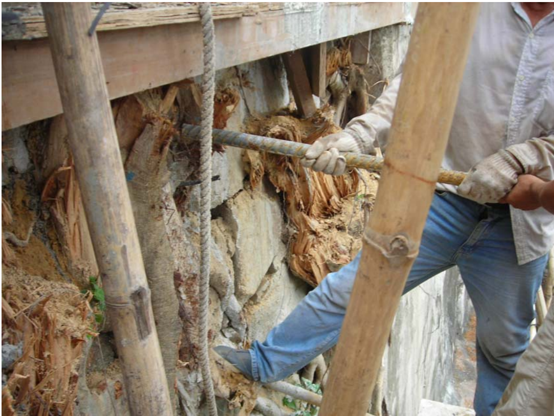
Plate 12 – Manual Removal of Soil Nail Reinforcing Bar (Photograph taken on 4 September 2006)
