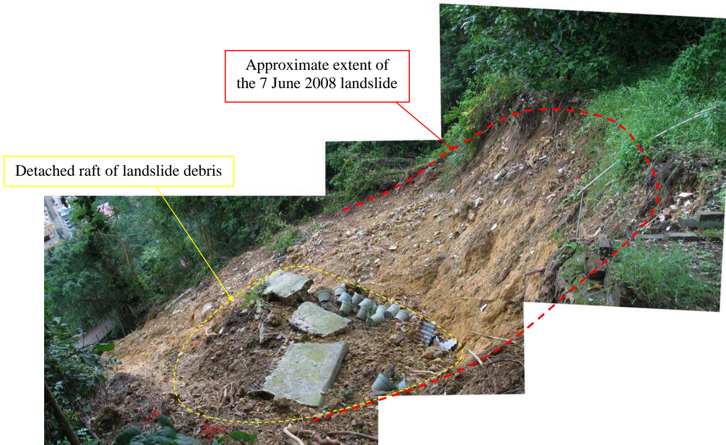
Plate 12 - Source Area of the 7 June 2008 Landslide and the Detached Raft of Landslide Debris at the Western Flank of the Landslide (Photograph taken on 10 June 2008)
