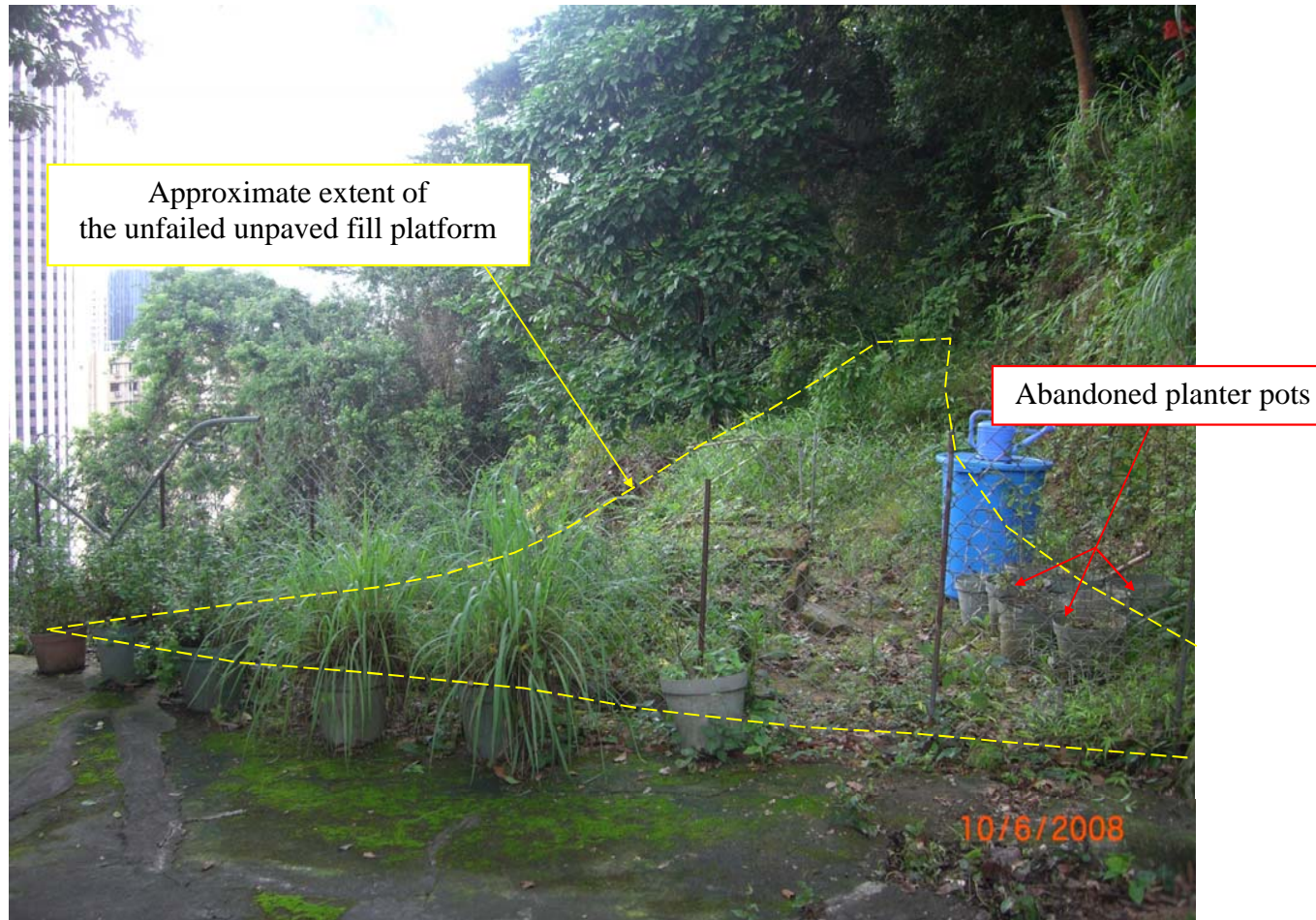
Plate 13 - General View of the Unfailed Unpaved Fill Platform at the Crest of the 7 June 2008 Landslide (Photograph taken on 10 June 2008)
