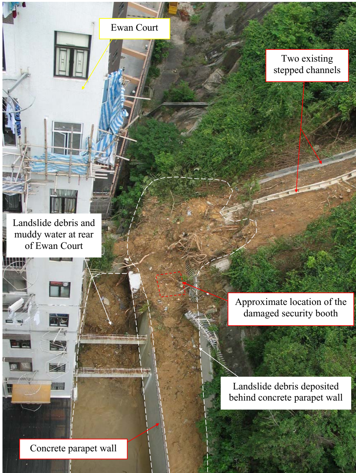
Plate 4 - Landslide Debris Deposited at the Rear of Ewan Court (Photograph taken on 10 June 2008)
