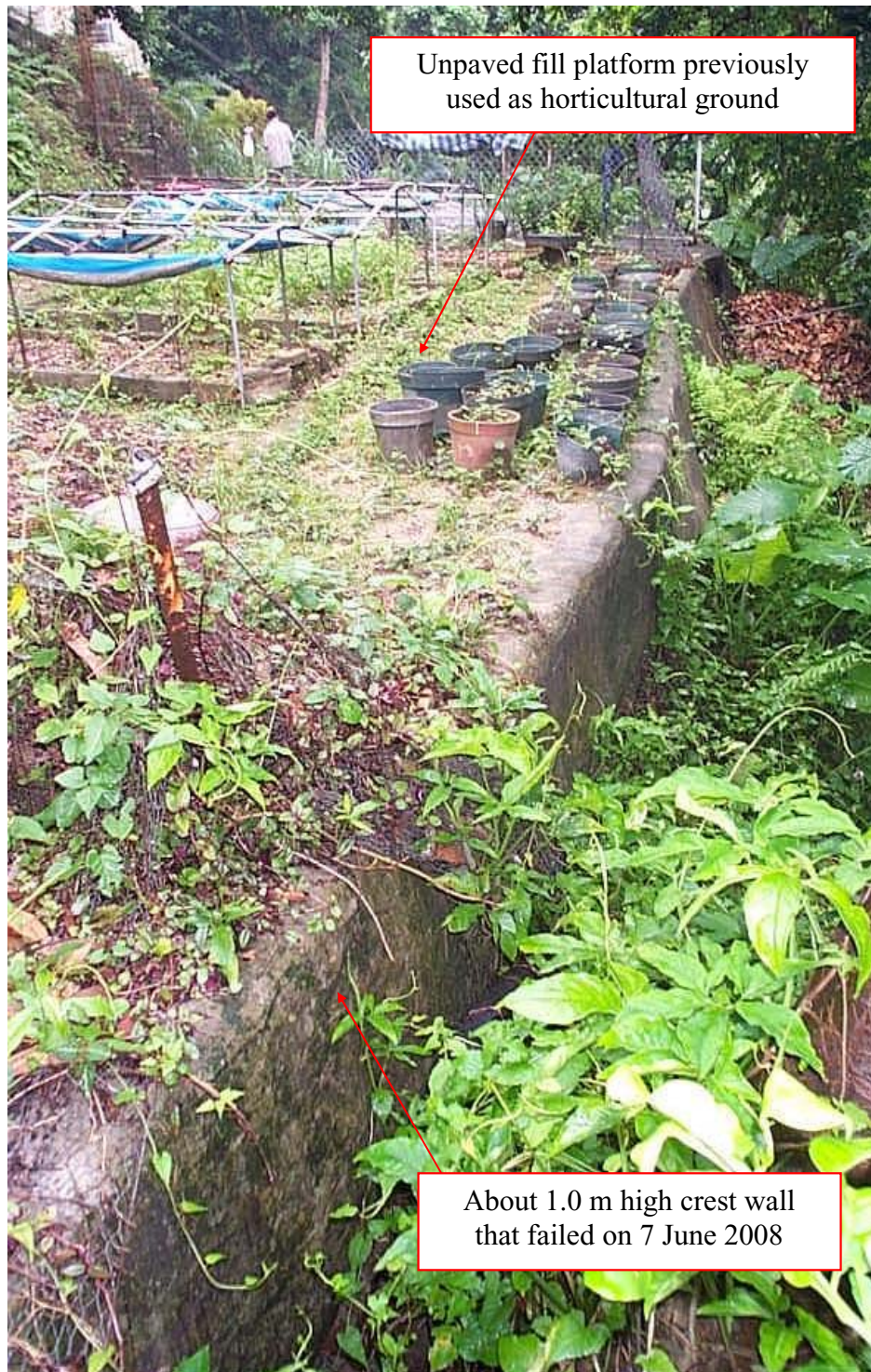
Plate 9 - General View of the Unpaved Fill Platform at the Crest of the 7 June 2008 Landslide (Photograph taken on 24 July 2001)
