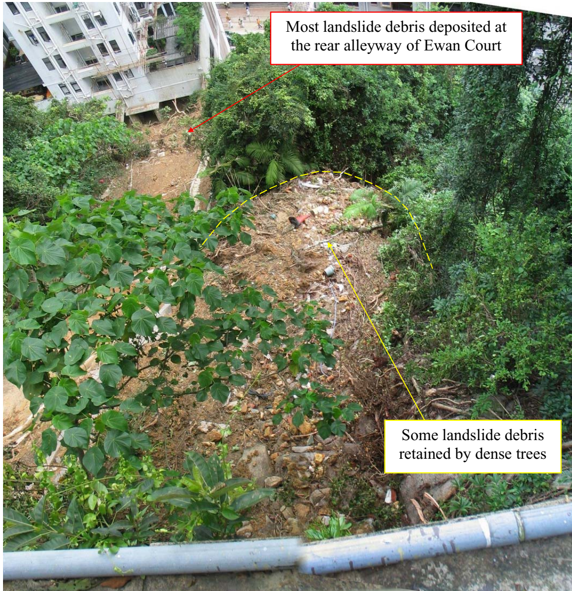
Plate 11 - Landslide Debris Retained by Dense Trees on the Hillside below Bowen Road (Photograph taken on 10 June 2008)
