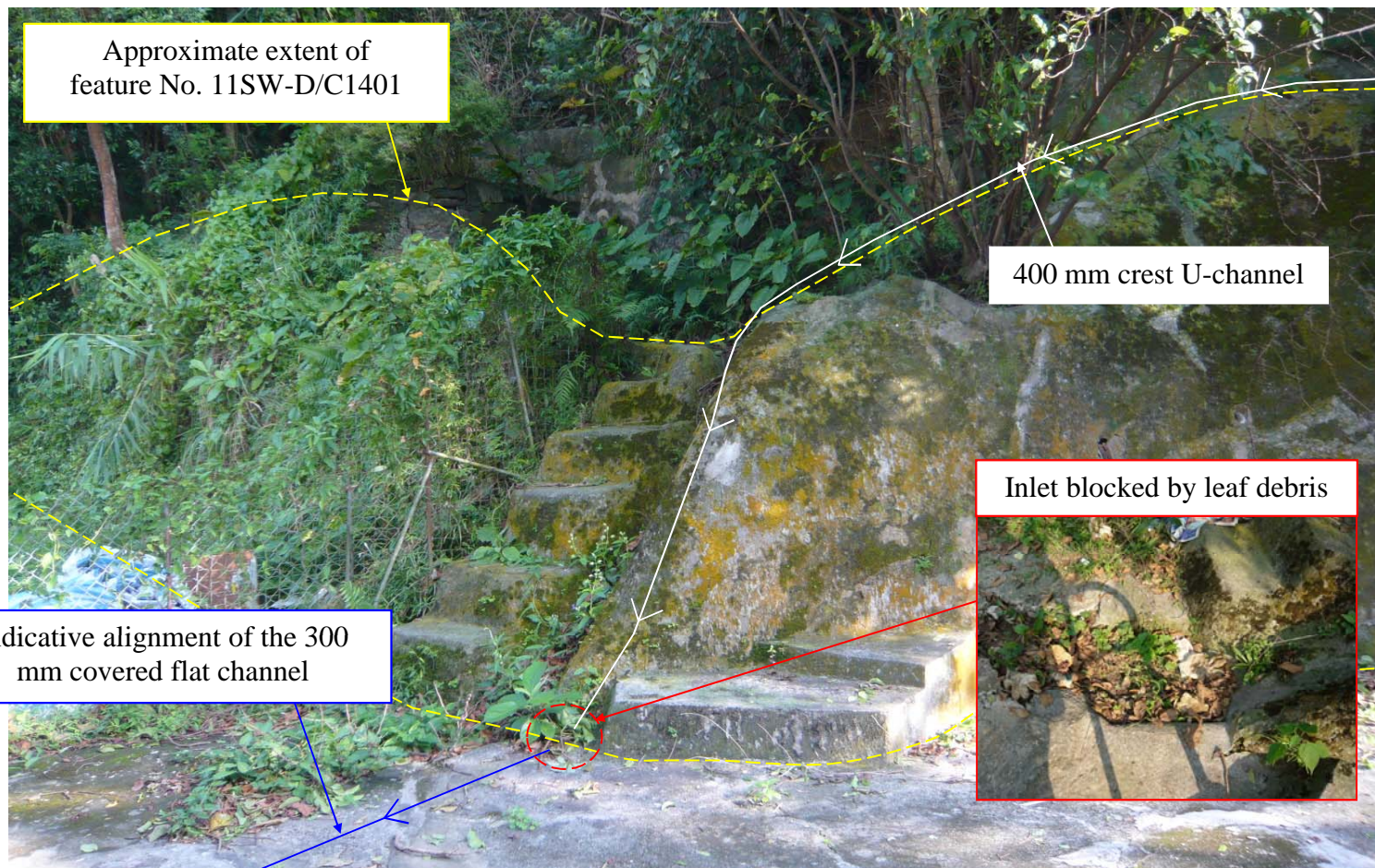
Plate 15 - Blocked Inlet to the 300 mm Covered Flat Channel at the Toe of Feature No. 11SW-D/C1401 (Photograph taken on 26 September 2008)
