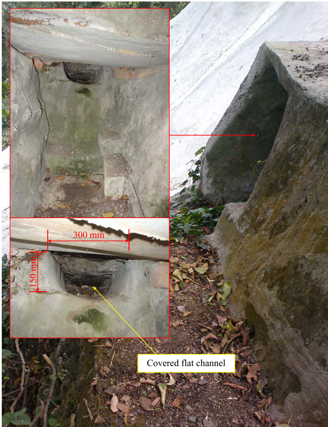
Plate 14 - Condition of the 300 mm Covered Flat Channel (Photograph taken on 23 April 2009)
