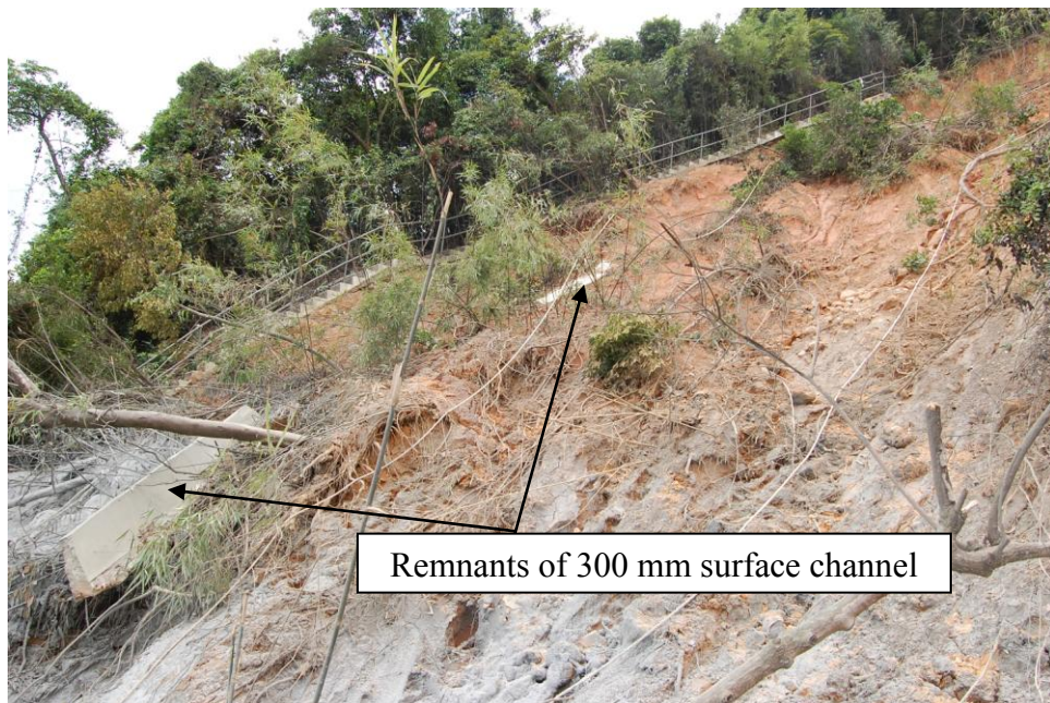
Plate 15 - Remnants of the 300 mm Surface Channel within the Lower Portion of the Primary Source Area (Photograph taken on 24 June 2008)
