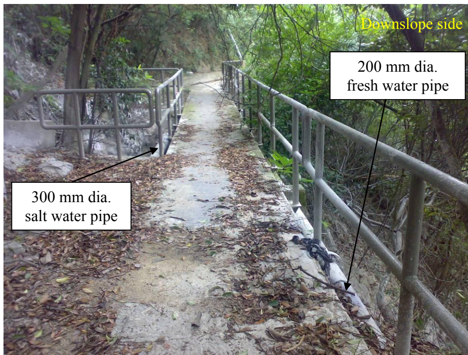
Plate 2 - Water-carrying Services along Pik Shan Path (Photograph taken on 23 September 2008)
