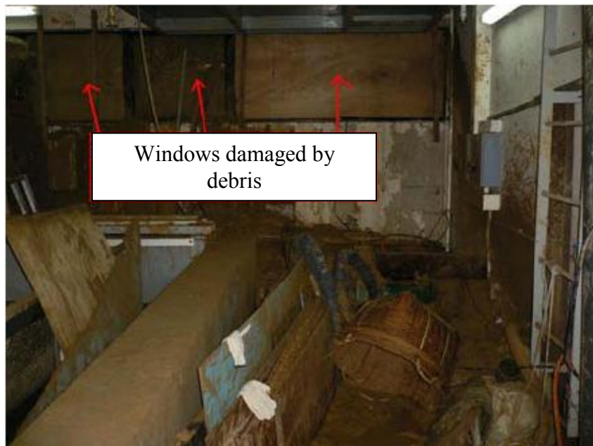
Plate 12 - Debris Flowed into LG3 of a Hydraulics Laboratory in CYC Building (Photograph taken on 8 June 2008 by HKU Estates Officer)
