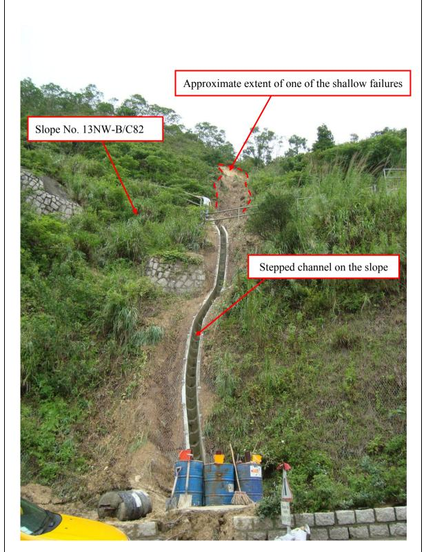
Plate 17 - The 7 June 2008 Landslide Incident (Landslide KS1) on Natural Hillside above Slope No. 13NW-B/C82, Keung Shan Road, Lantau Island (Incident No. 2008/06/0132)
