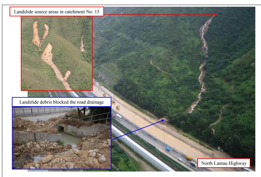
Plate 8 - The 7 June 2008 Landslide Incident on Natural Hillside in Catchment No. 15 above North Lantau Highway, Tung Chung (Incident No. 2008/06/0346)
