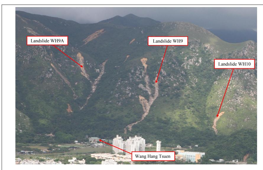
Plate 14 - The 7 June 2008 Landslide Incidents on Natural Hillside above Wang Hang Tsuen, Tai O (Incident Nos. 2008/06/0382, 2008/06/0396 and 2008/06/0479)
