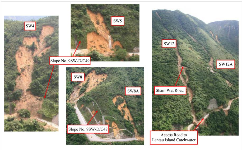
Plate 21 - The June 2008 Landslide Incidents above Sham Wat Road (Incident Nos. 2008/06/0435, 2008/06/0439, 2008/06/0440, 2008/06/0441, 2008/06/0555 and LI/2008/06/2013)
