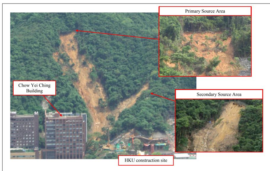
Plate 2 - The 7 June 2008 Landslide Incident on Natural Hillside behind Chow Yei Ching Building at the University of Hong Kong, Pok Fu Lam (Incident No. 2008/06/0193)
