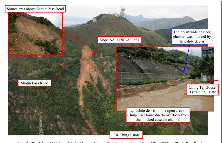
Plate 7 - The 7 June 2008 Landslide Incident on Natural Hillside above Slope No. 11NE-A/C351 at Shatin Pass Road (Incident No. 2008/06/0170)
