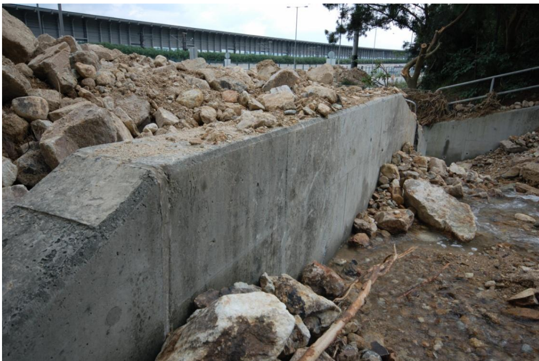
Plate 29 - No Impact Marks on the Concrete Head Wall Connected to the Drainage Inlet in Catchment No. 15 (Photograph taken on 8 June 2008)
