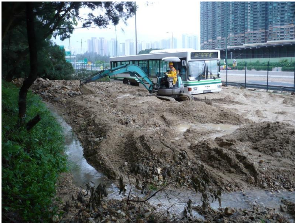
Plate 6 - Up to 0.5 m thick Sandy/Gravelly Deposit on Cheung Tung Road below Catchment No. 16 (Photograph taken at 2 pm on 7 June 2008)
