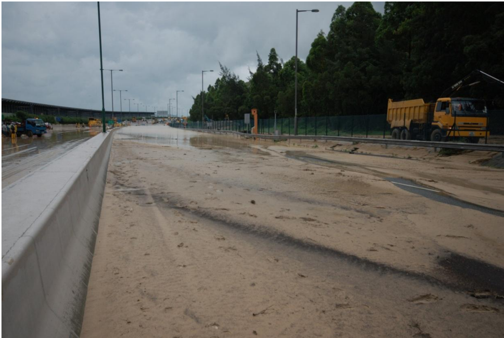
Plate 4 - Fines Observed on North Lantau Highway (Photograph taken at 2 pm on 7 June 2008)
