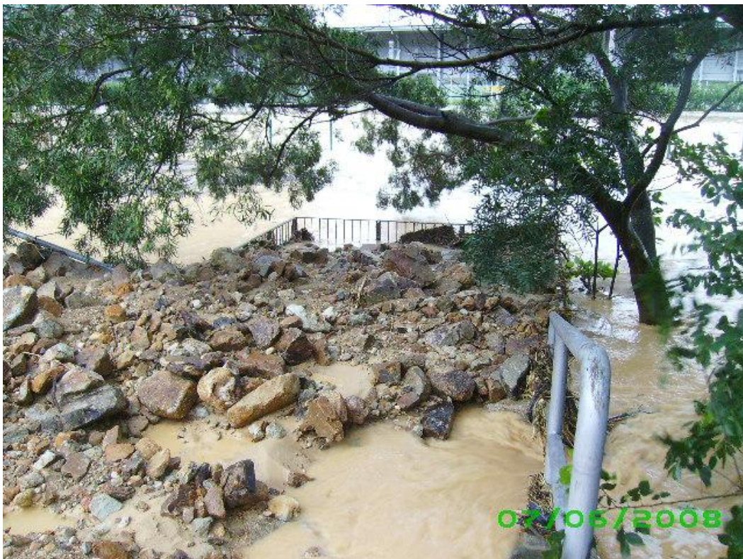
Plate 27 - Drainage Inlet Blocked with Clast-Supported Bouldery Debris at CH850 (Photograph taken at 11:30 am on 7 June 2008)
