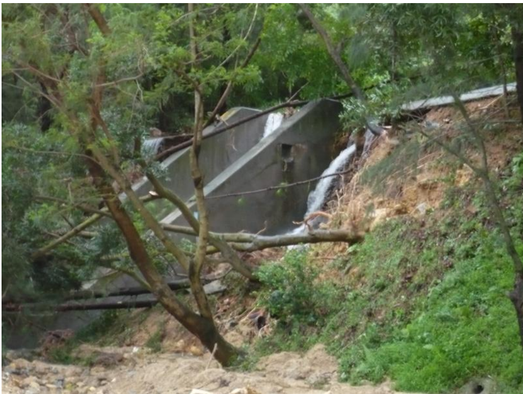
Plate 5 - Erosion at the Side of Drainage Channel at the Toe of Catchment No. 16 (Photograph taken at 2-3 pm on 7 June 2008)
