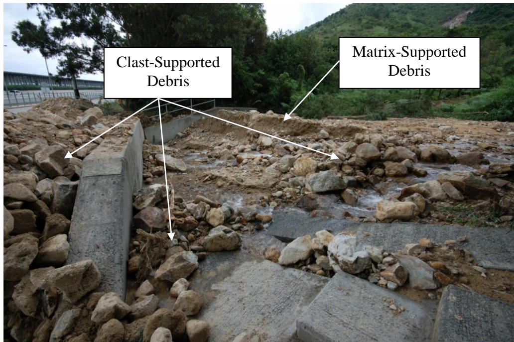
Plate 26 - View of Debris Beyond CH735 in Catchment No. 15 (Photograph taken on 8 June 2008)
