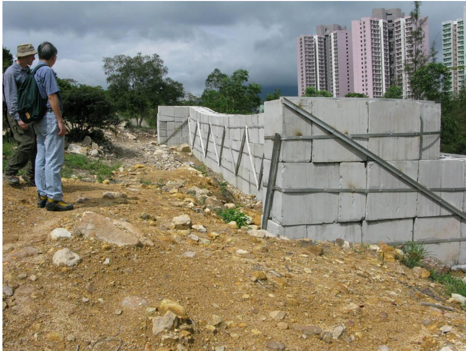
Plate 42 – Temporary Barrier above Slope No. 9SE-B/C52 in Catchment No. 24 (Photograph taken on 15 June 2009)
