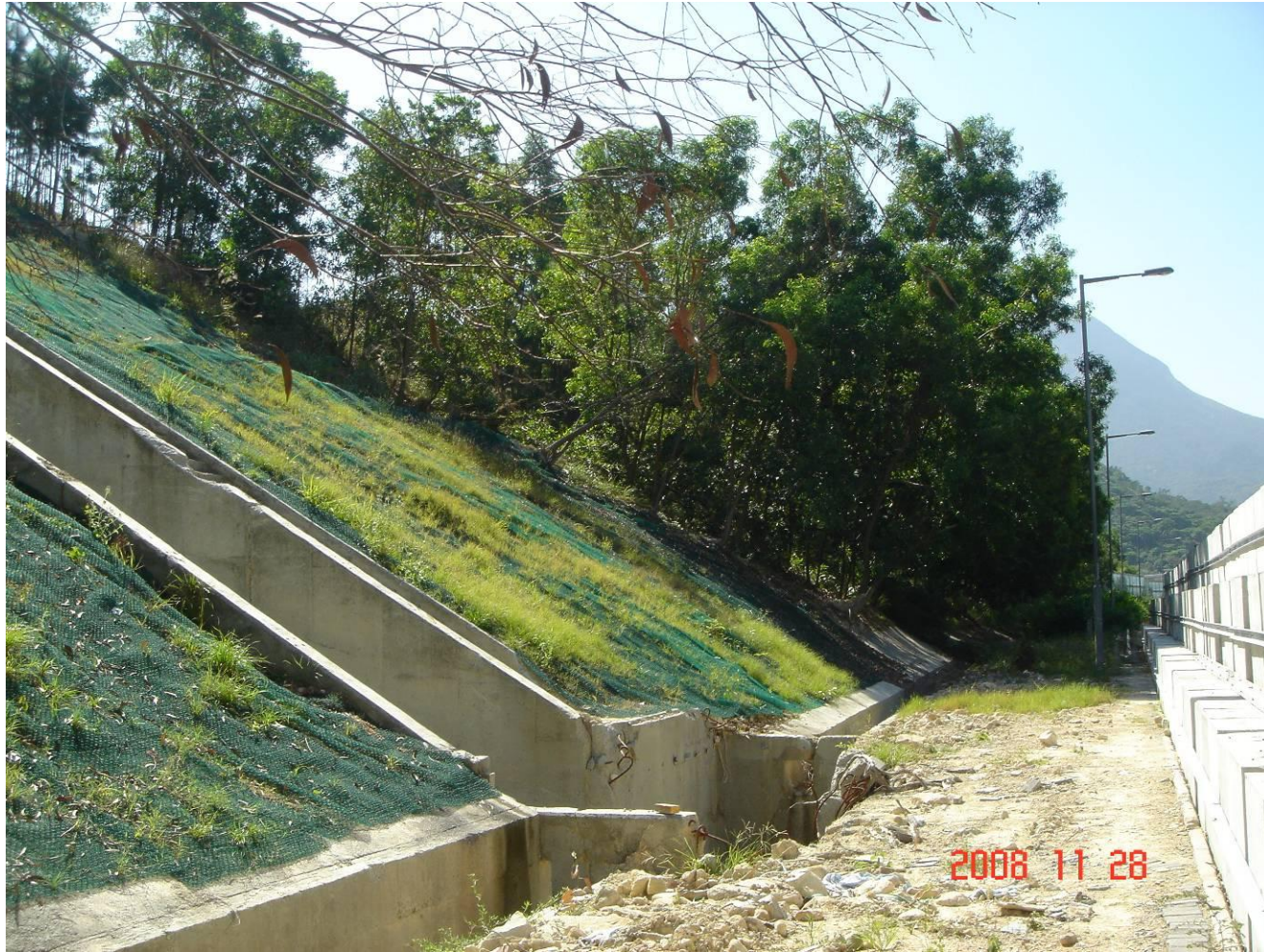
Plate 41 – Damage to Concrete Channel at Toe of Slope No. 9SE-B/C27 in Catchment No. 30 (Photograph taken on 11 November 2008)
