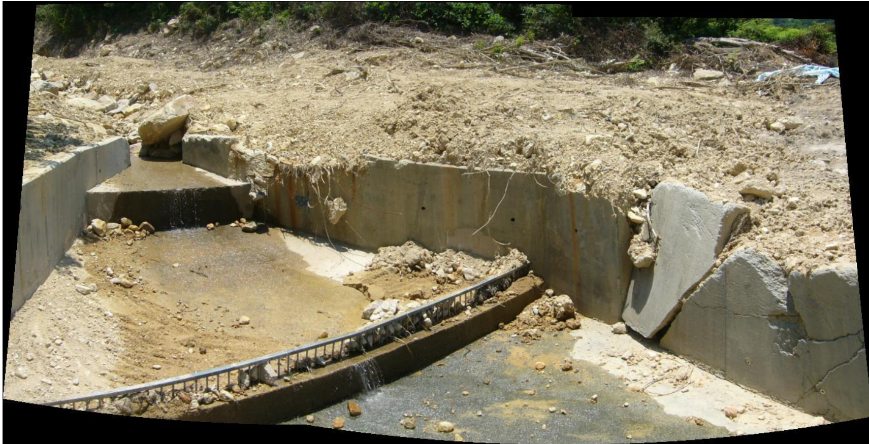
Plate 40 – Damage to Concrete Drainage Channel at West of Slope No. 9SE-B/C27 in Catchment No. 30 (Photograph taken on 25 July 2008)
