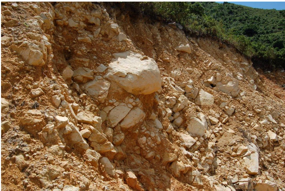
Plate 30 – Close-up of Talluvium in Backscarp of Landslide No. L25 in Catchment No. 30 (Photograph taken on 21 July 2008)
