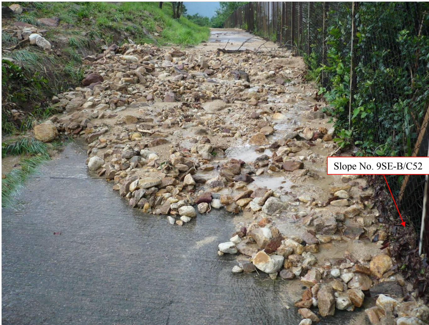
Plate 23 – Small Volume of Outwash from Landslide No. L2 in Catchment No. 25 Deposited on Concrete Path above Crest of Slope No. 9SE-B/C52 (Photograph taken on 7 June 2008)
