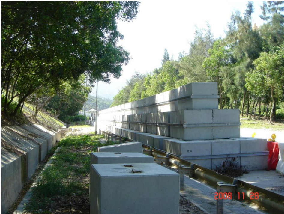
Plate 43 – Temporary Barrier along Yu Tung Road below Catchment No. 30 (Photograph taken on 28 November 2008)
