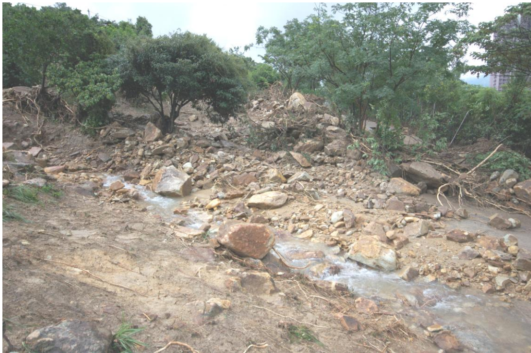
Plate 13 – Debris Deposited along the Southern Side of the Drainage Line between CH547 and CH605 in Catchment No. 24 (Photograph taken on 7 June 2008)
