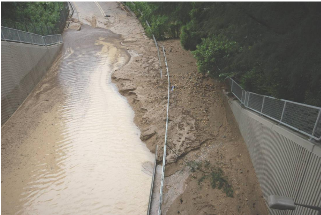
Plate 3 - Outwash from Landslide No. L3 in Catchment No. 24 and Flooding of Cheung Tung Road (Photograph taken on 7 June 2008)
