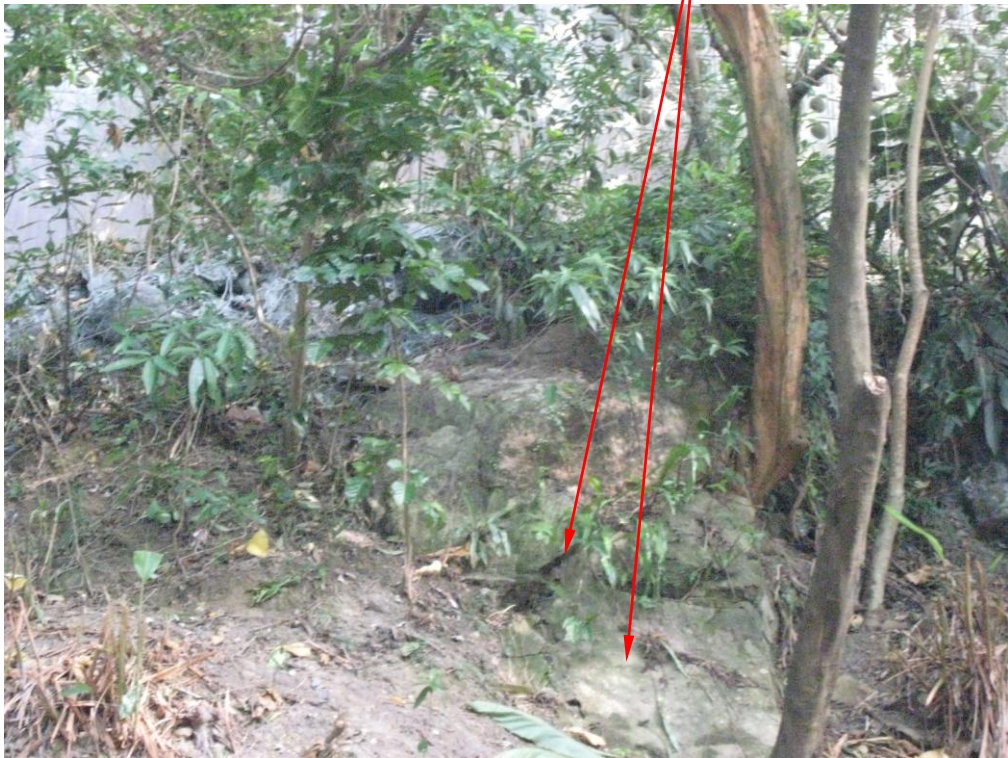
Plate 26 - Rock Outcrops/Corestones Exposed on Ground Surface above Crest of Retaining Wall No. 11SW-A/R677 (Photograph taken on 25 July 2007)
