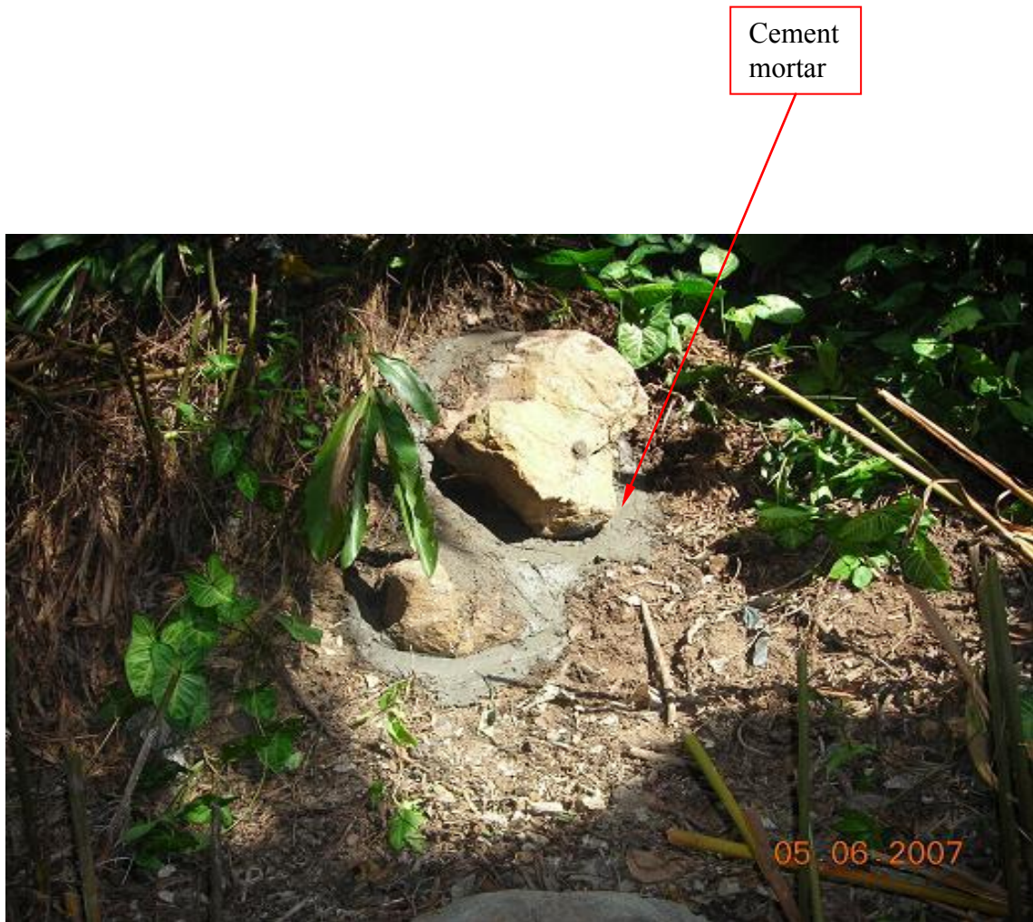
Plate 21 – Boulder Stabilisation Works Completed by HyD following the 27 May 2007 Boulder Fall (Photograph taken on 5 June 2007)
