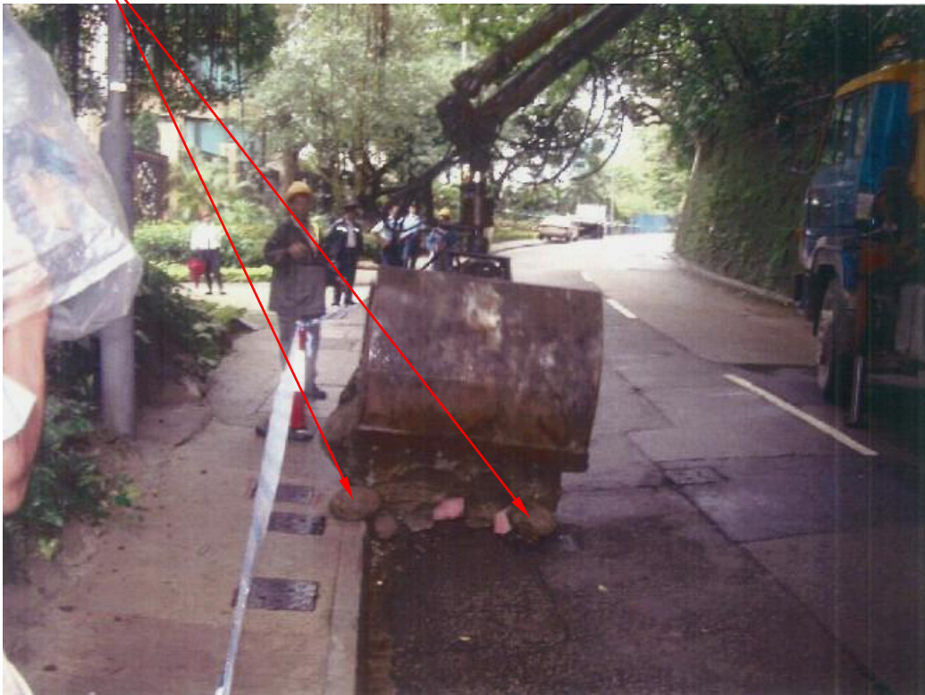
Plate 7 - Cobble-sized Rock Fragments Brought down with the Main Boulder (Photograph taken by HyD on 27 May 2007)
