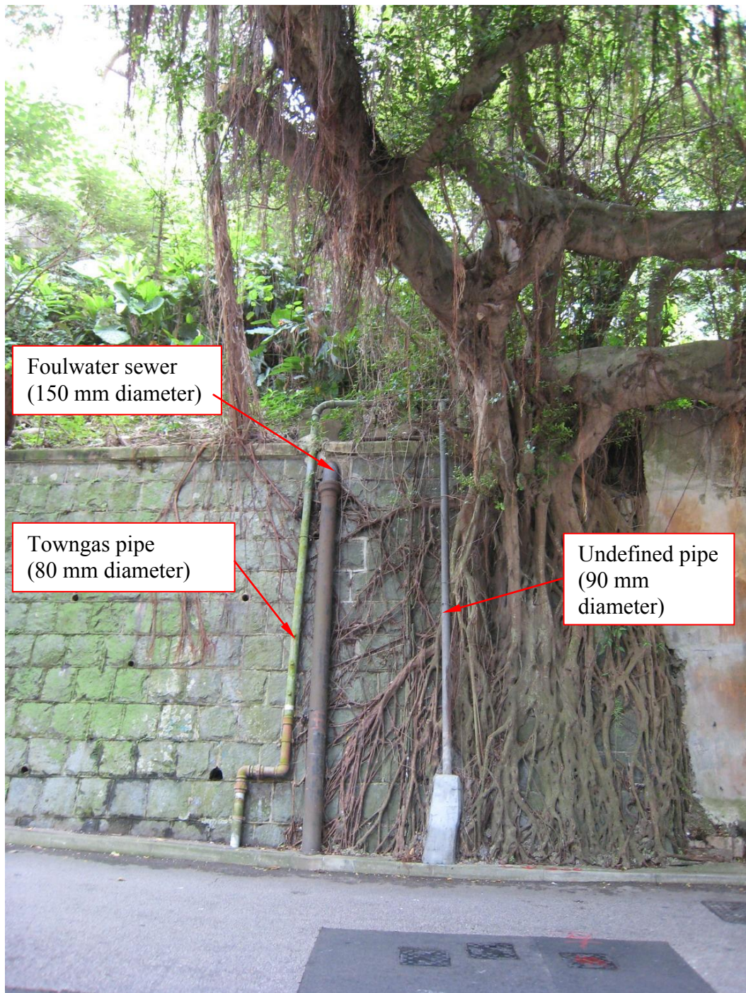
Plate 6 – Exposed Pipelines and Large Tree at Western End of Retaining Wall No. 11SW-A/R677 (Photograph taken on 5 September 2007)
