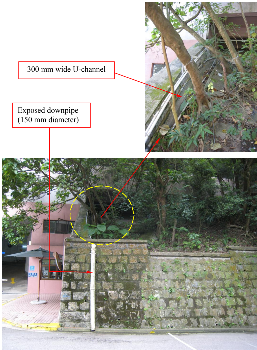
Plate 5 – Exposed Downpipe and U-channel at the Eastern End of Retaining Wall No. 11SW-A/F677 (Photograph taken on 5 September 2007)
