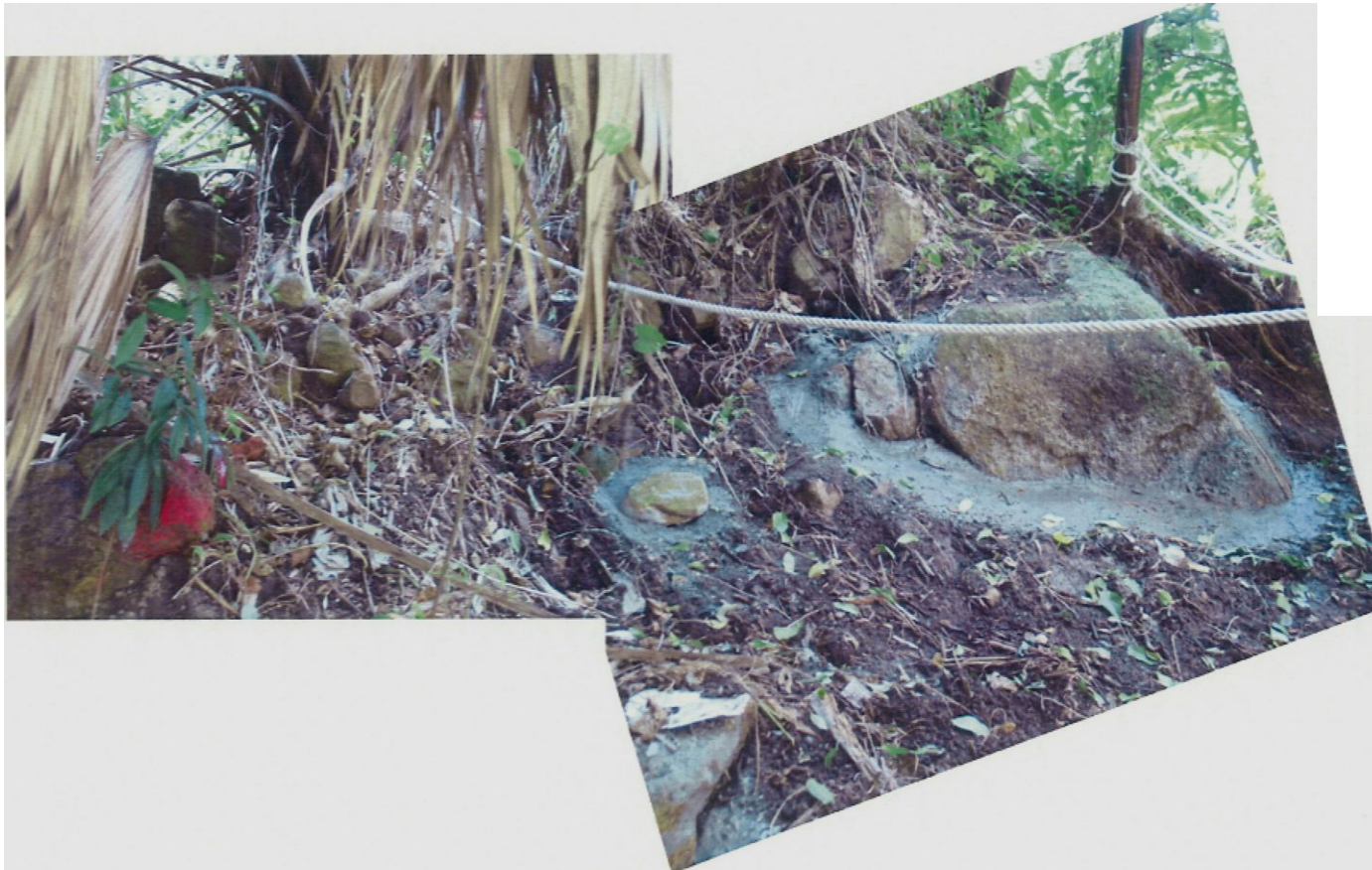
Plate 9 - Boulder Stabilisation Works Completed by HyD following the 27 May 2007 Boulder Fall (Photograph taken by GEO on 4 June 2007)
