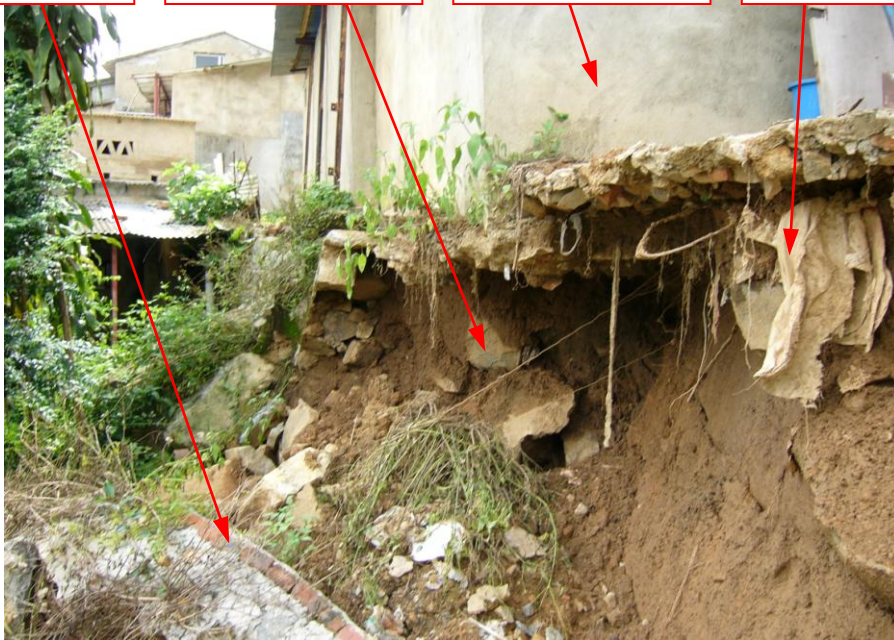
Plate 10 - Undermined Flimsy Squatter Structure (Photograph taken on 29 June 2005 by MGSL)
