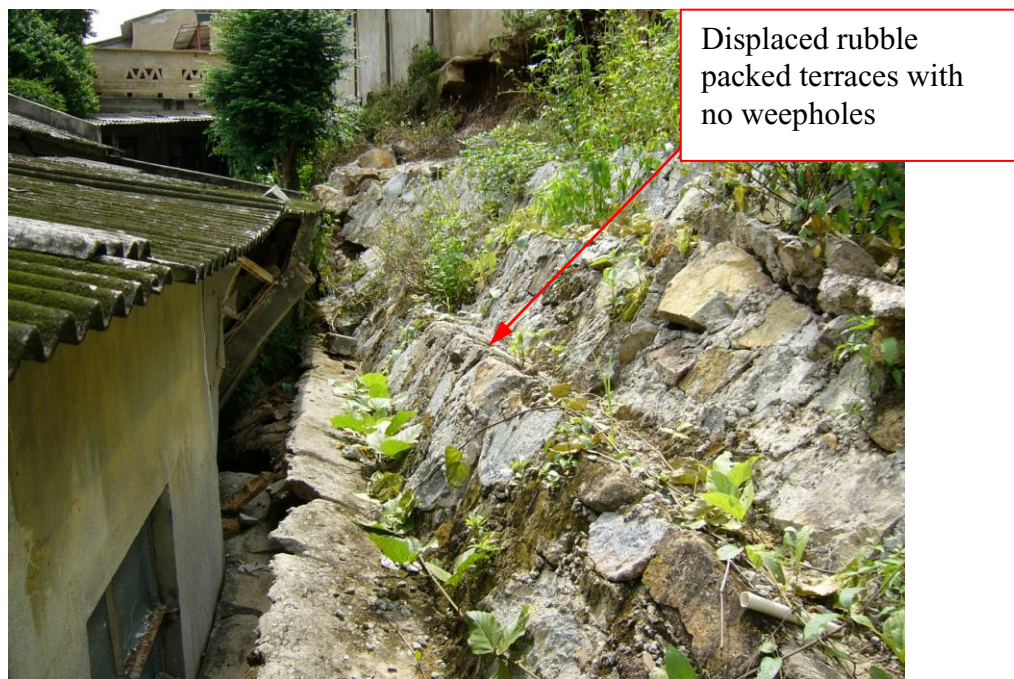
Plate 8 - Displaced Rubble Packed Terraces above Failed Toe Wall (Photograph taken on 29 June 2005 by MGSL)
