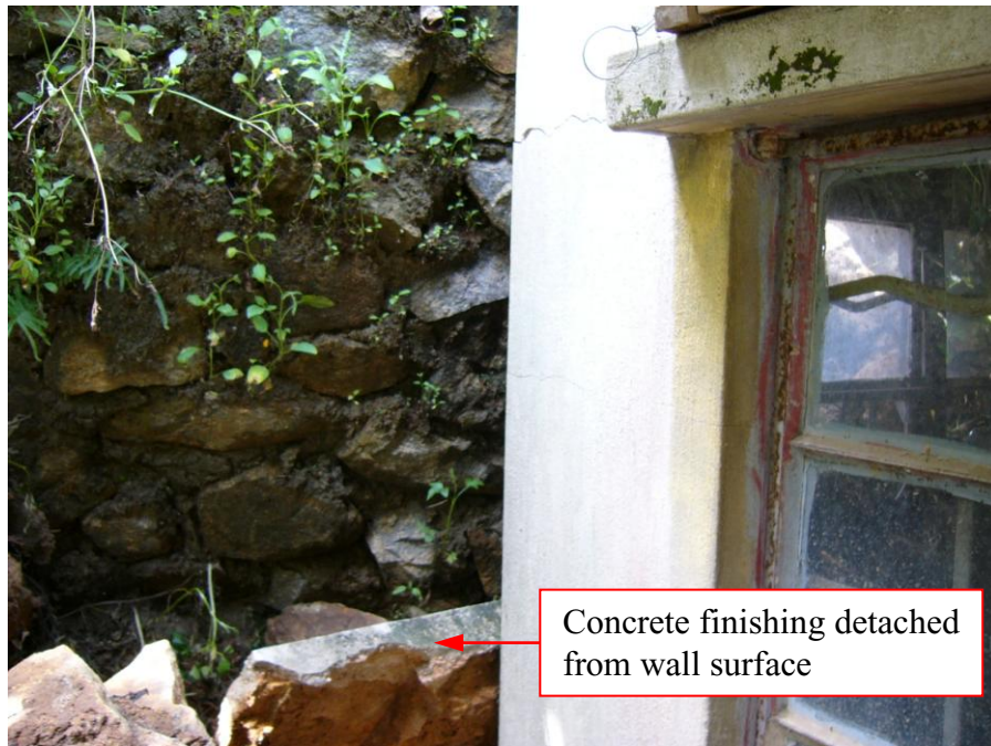
Plate 7 - Concrete Finishing of Toe Wall (Photograph taken on 29 June 2005 by MGSL)
