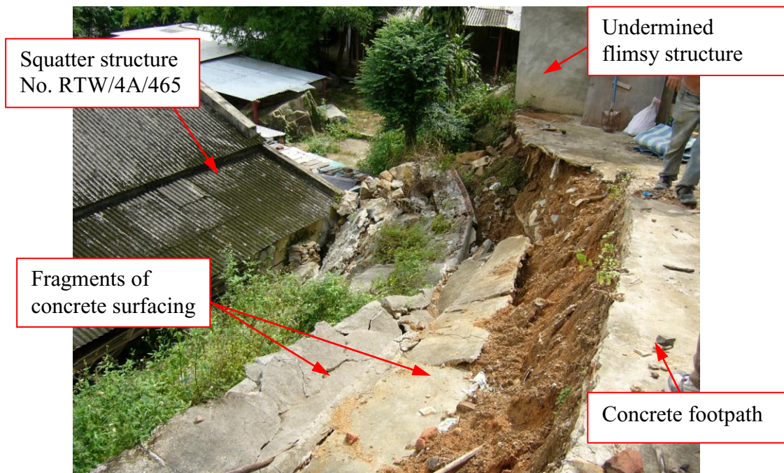
Plate 4 - General View of the Landslide from Slope Crest (Photograph taken on 29 June 2005 by MGSL)
