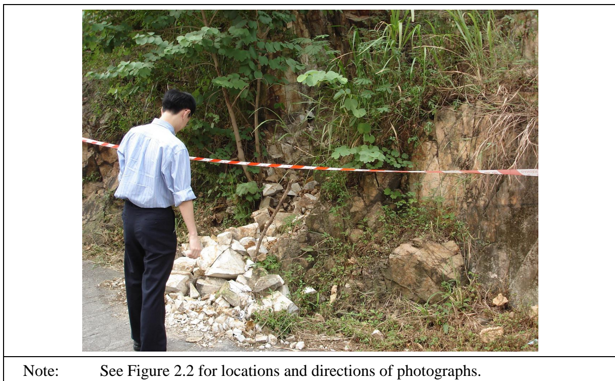
Figure 5.3 View of the Detached Rock Blocks from the 12 September 2007 Rockfall (Photograph Taken by ArchSD on 17 September 2007)
