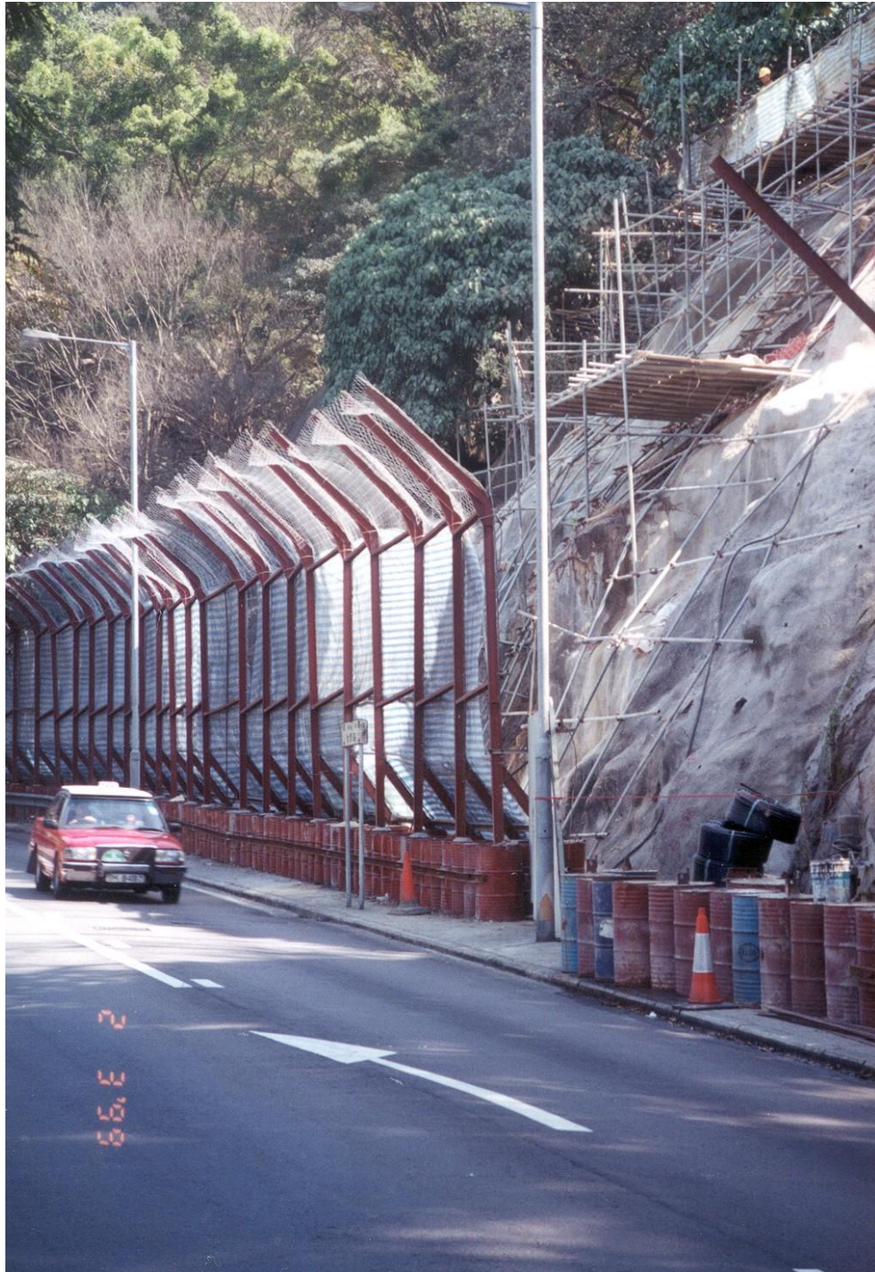
Plate 6.2 - Example of a CED Standard Temporary Fence (Type B)
