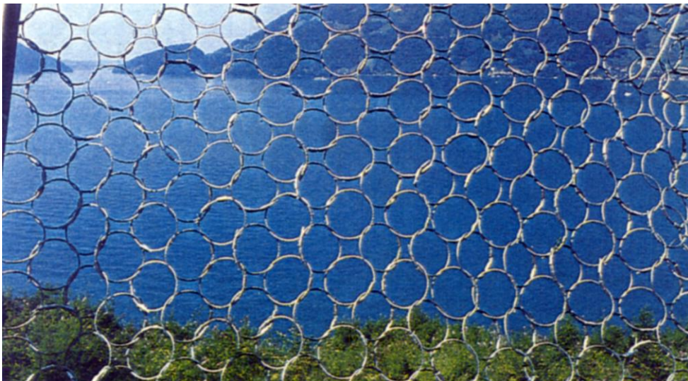
Plate 6.9 - Example of Specialised Rockfall Fences (from Tubosider)
