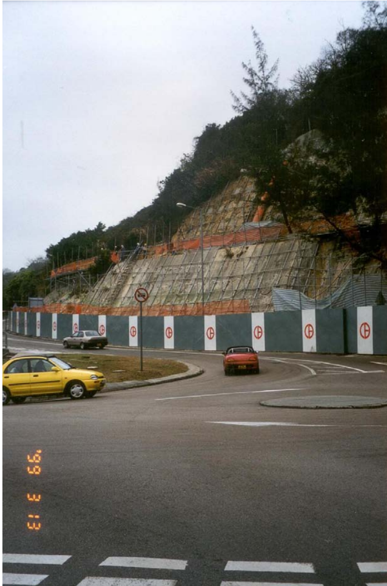
Plate 6.3 - Example of a Typical Hoarding Type II
