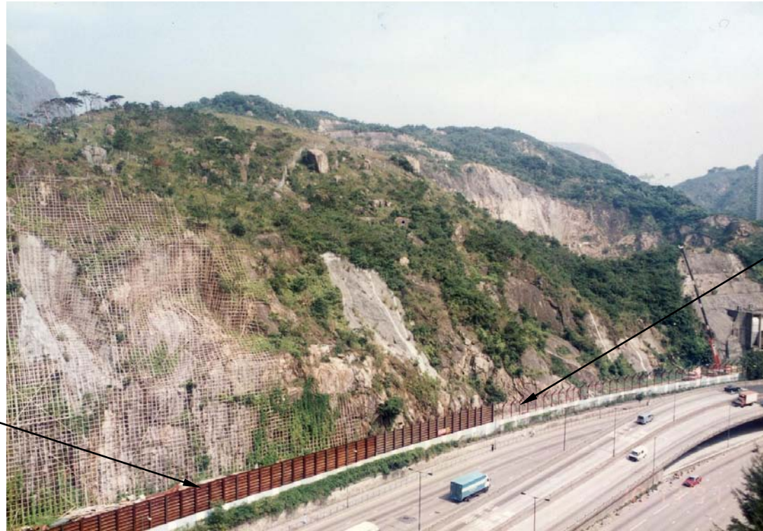
Plate 6.5 - Example of Upgraded Type A CED Standard Temporary Fence Used at Kwun Tong Road
