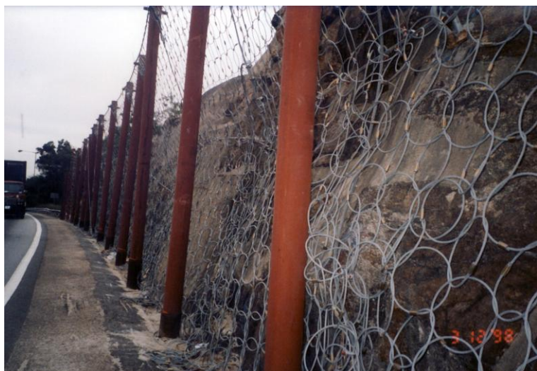
Plate 6.6 - Example of Specialised Rockfall Fences (from Geobrugg)
