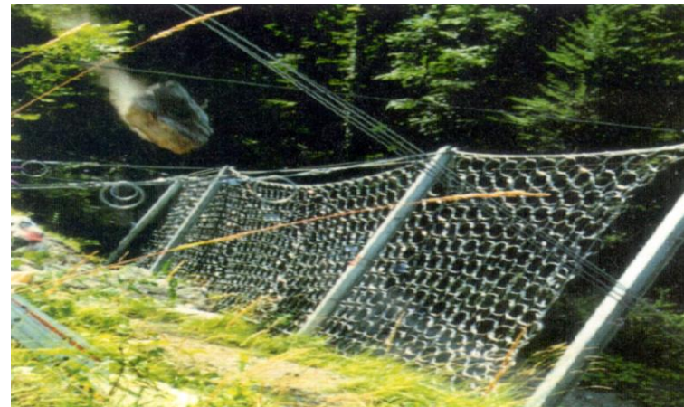
A typical Rockfall Barrier, installed by Geobrugg
