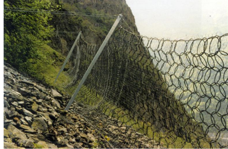
A typical Rockfall Barrier, installed by EI Montagne
