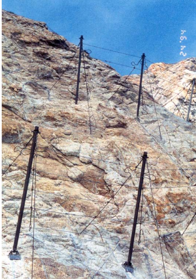
A typical Rockfall Barrier, installed in Italy in 1994 by Cento Laboratorio Industriale Osservazioni Scientifiche (C.L.I.O.S.)
