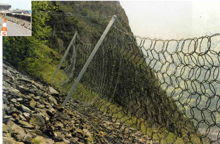
Plate 6.7 - Example of Specialised Rockfall Fences (from EI Montagne)
