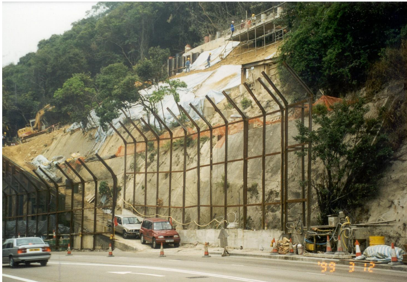
Plate 6.1 - Example of a CED Standard Temporary Fence (Type A)
