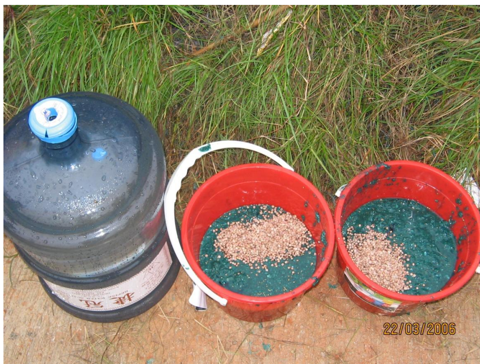
(b) View of seeds mixing with hydroseeding mix
