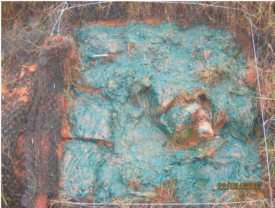
(d) View of the planting plot following application of hydroseeding
