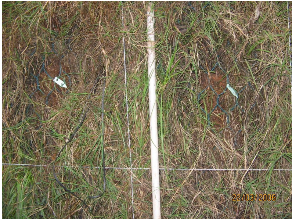
(b) View of the planting area following spot-sowing (Note: Each label tag indicates location of each seed planted underneath the slope surface.)
