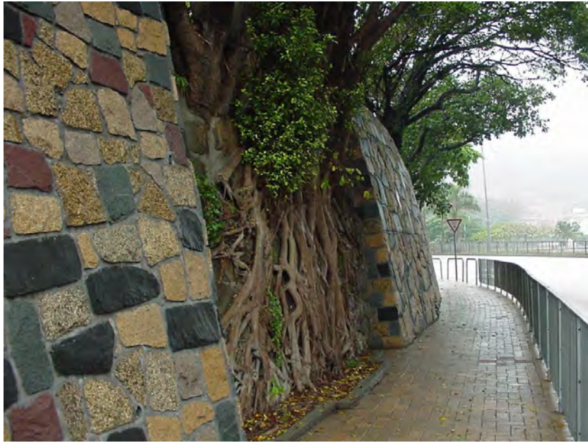
Figure 17 - Feature No. 11SW-C/R38 Upgraded Using Mass Concrete Wall and Finished with the Old Granite Blocks
