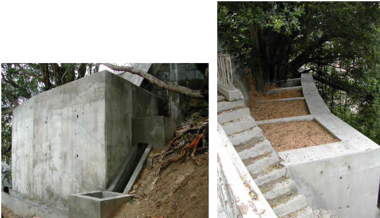
Figure 16 - Feature No. 11SW-C/R476 Upgraded Using Soil Nails, L-shaped Wall and Planter
