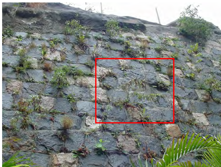
Figure 6 - Joints between Masonry Blocks at the Location of Fallen Tree were Repaired
