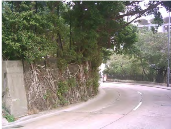
Figure 3 - The Surface Roots of Chinese Banyan Form a Dense Network Covering the Stone Façade at Hospital Road
