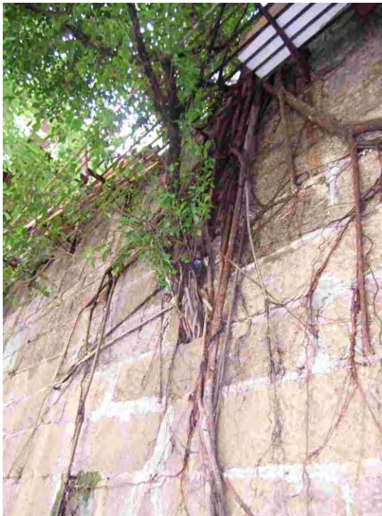
Figure 12 - Wall Tree with Weak Anchorage between Roots and Wall
