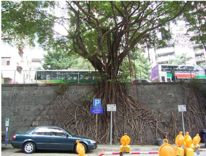
Figure 1 - A Chinese Banyan Growing Spontaneously on a Masonry Wall at High Street
