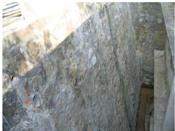
Figure 15 - Feature No. 11SW-A/R1086 before and after Upgrading Works Using Soil Nails
