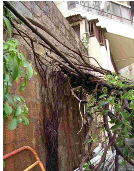
Figure 11 - Tree failure on Feature No. 11SW-B/R735
