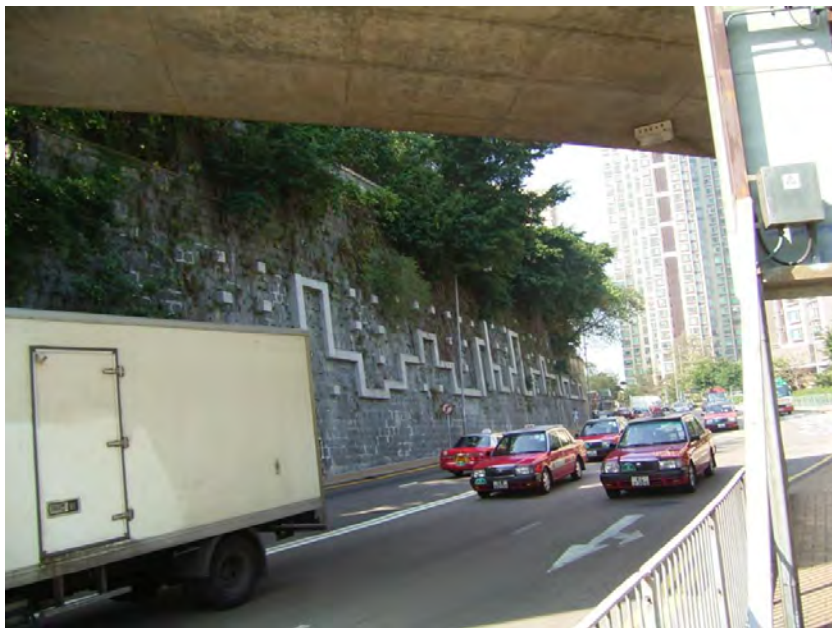
Figure 18 - Feature No. 11SW-A/R346 Upgraded Using Soil Nails
