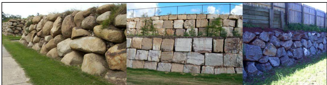
Figure 6.2.5 - Example of Rubble Wall Pattern
