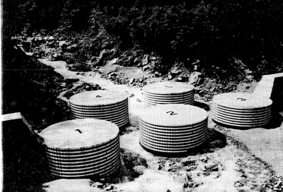
Photo 3 Yotagiri River steel cell dam
