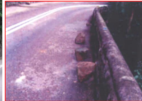
Close-up view of the fallen masonry blocks
