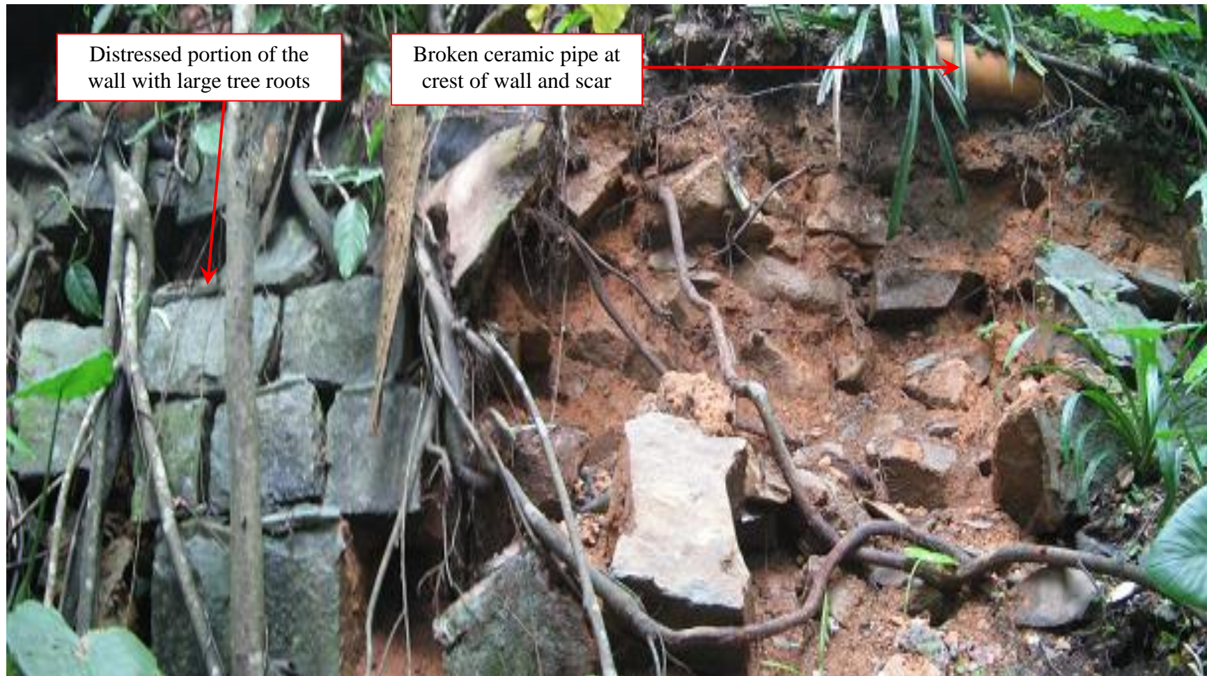
Plate 8 - Failure Scar on the Squared Masonry Retaining Wall (Photograph taken on 11 June 2007)
