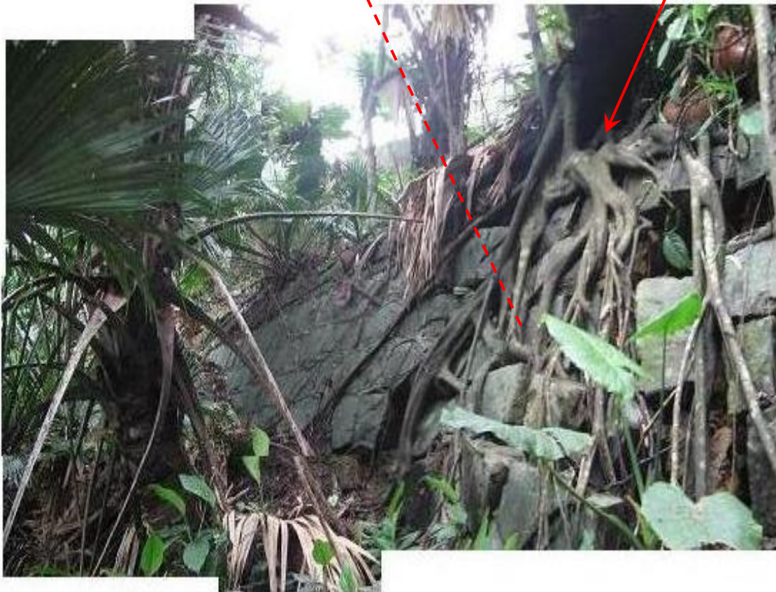
Plate 10 - Portion of the Masonry Retaining Wall in an Advanced State of Distress (Photograph taken on 13 June 2007)
