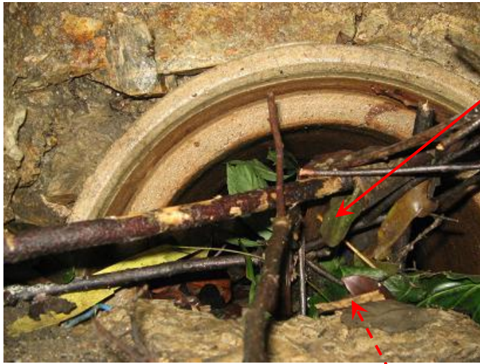
Blocked 150 mm diameter cross-road drain (viewed from inside the open catch pit)
