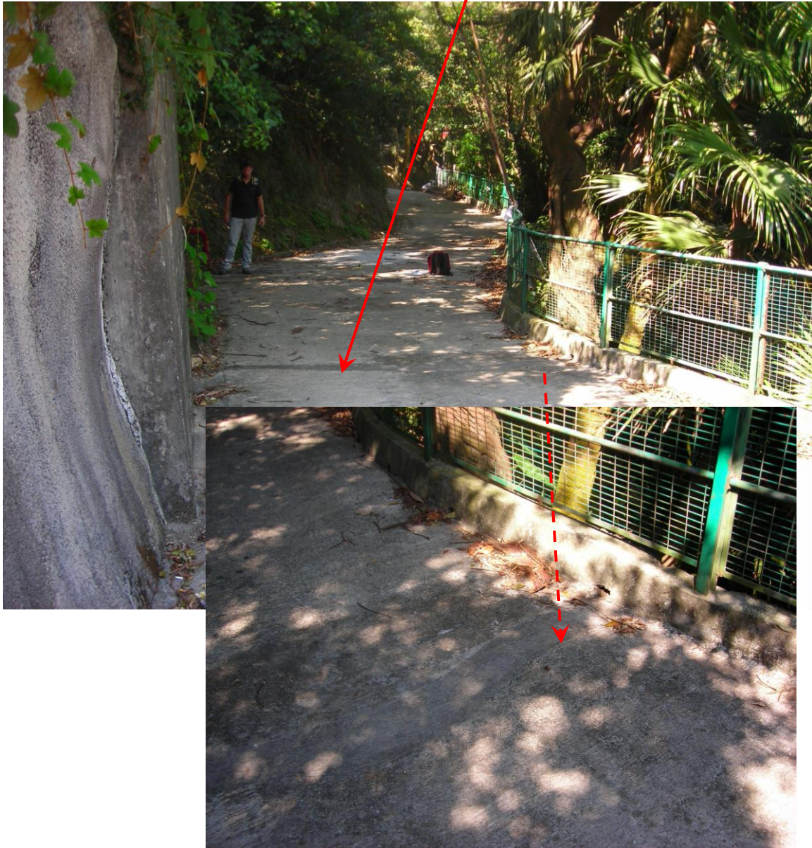
Plate 13 - Crack on the Access Road to the South of the Failure (Photograph taken on 7 November 2007)
