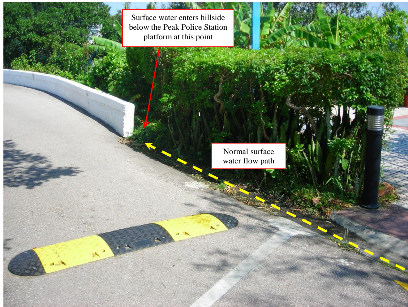
Plate 7 - Peak Police Station Access Road Surface Drainage Discharge Point (Photograph taken on 7 November 2007)
