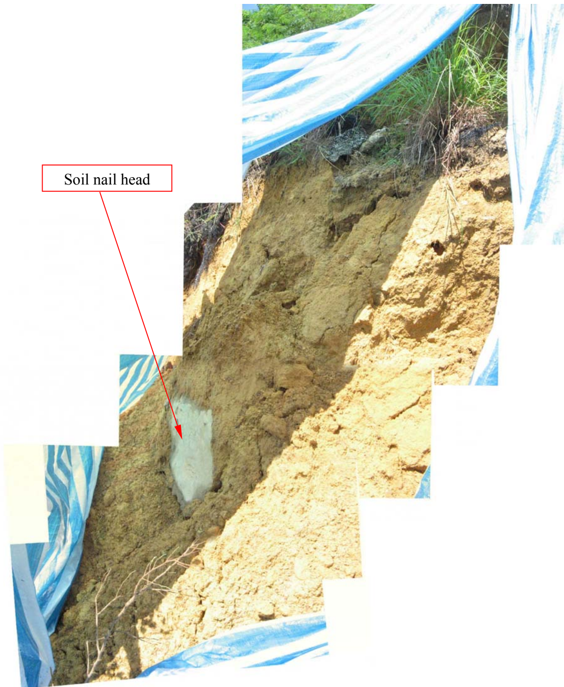
Plate 13 – Close View of Soil Nail No. 2 (Photograph taken on 30 August 2005)
