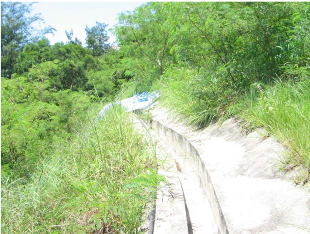
Plate 16 – Surface Channel above Landslide Scar (Photograph taken on 30 August 2005)
