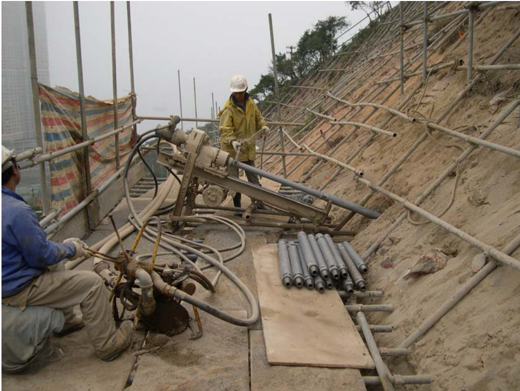
Plate 1 - Common Practice of Drilling of a Soil Nail using a Pneumatic Percussive Rig
