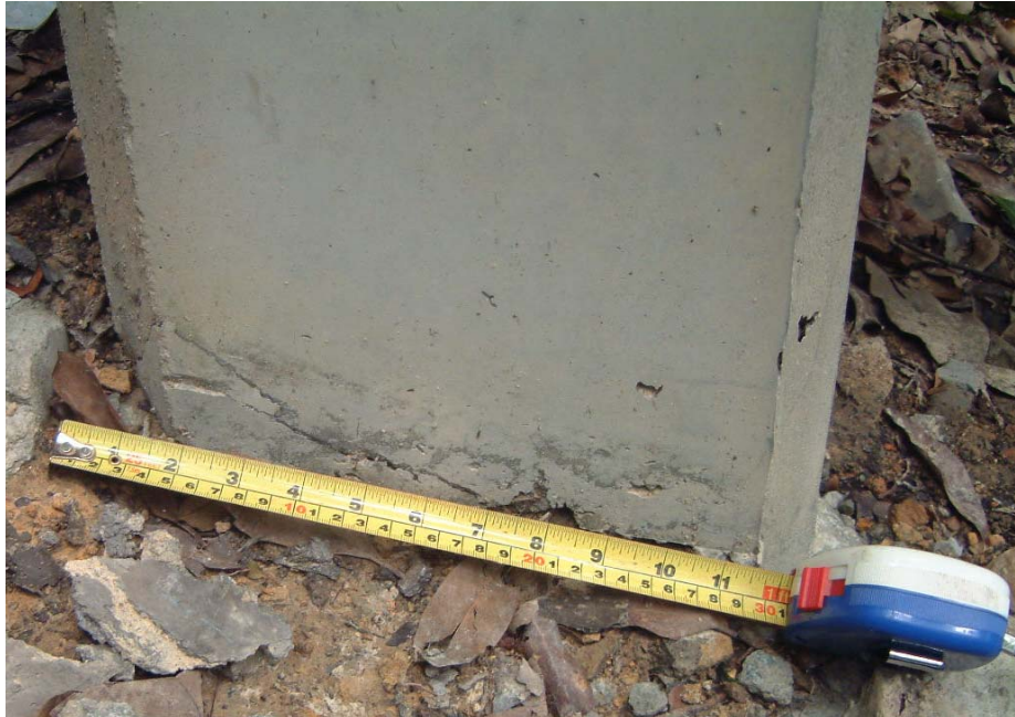
Plate 12 – View of Hairline Crack at the Base of Concrete Plinth Support to the Replacement Ductile Iron Pipeline (Photograph taken by FSW on 12 September 2005)
