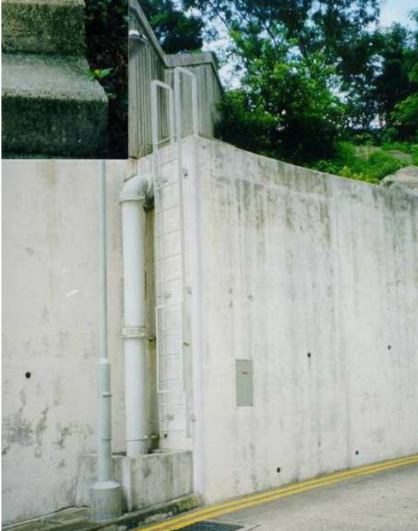
(1) Exposed Down Pipe on Retaining Wall
