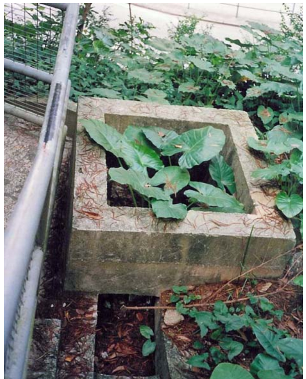
(4) Catchpit at Crest of Slope
