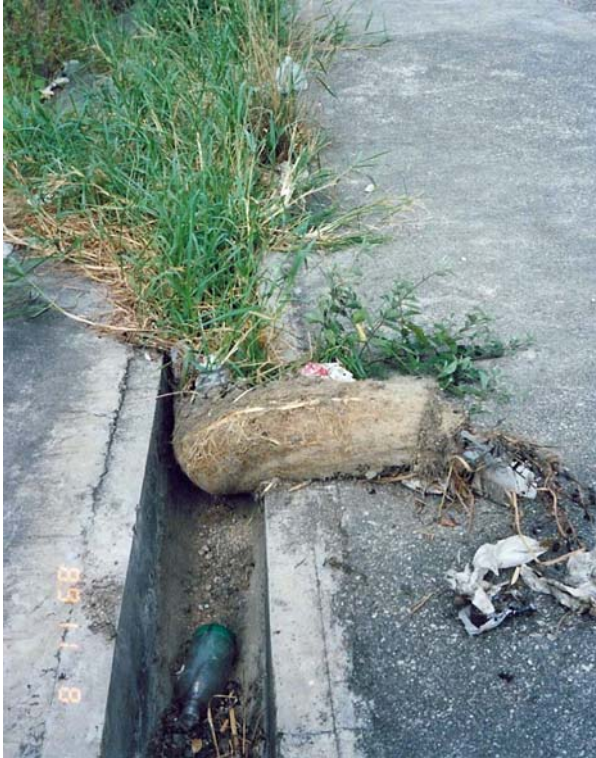
(1) U-channel along Crest of Slope
