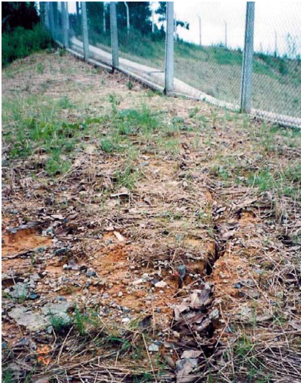
(1) Tension Crack on Slope
