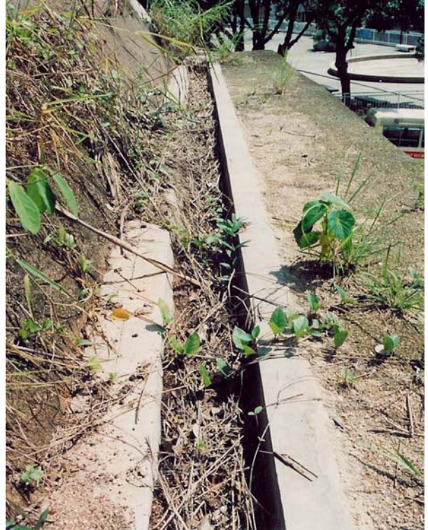
(2) U-channel along Berm of Slope
