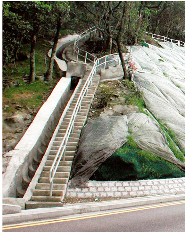
(4) Combined Stepped Channel and Stairway
