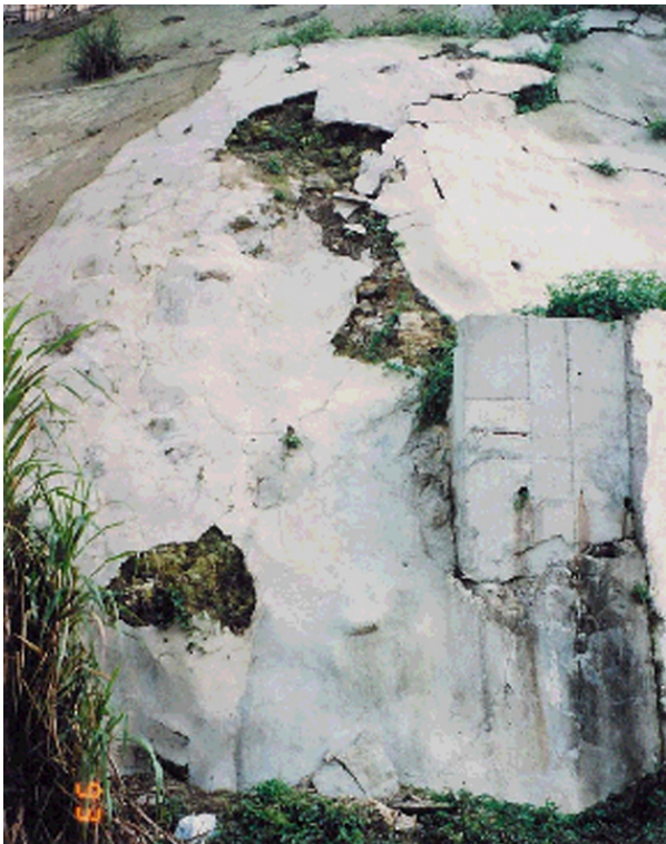
(3) Cracked Chunam Surface
