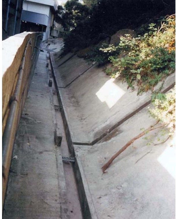
(2) U-channel along Toe of Slope
