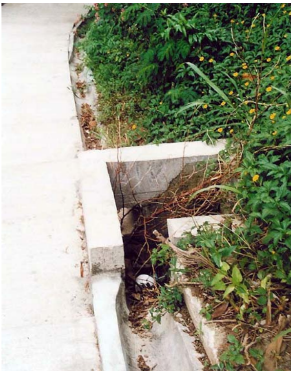
(3) Catchpit at Toe of Slope
