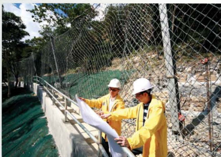
Geotechnical engineers inspecting a flexible barrier under LPMiP
