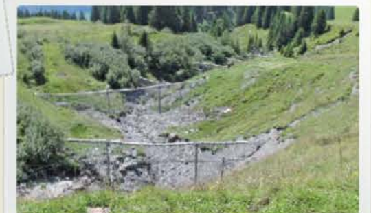
Multiple flexible barriers in Switzerland - Photo courtesy of Geobrugg*
