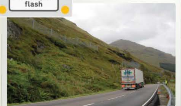
Use of flexible barriers for mitigation of landslides in Scotland
