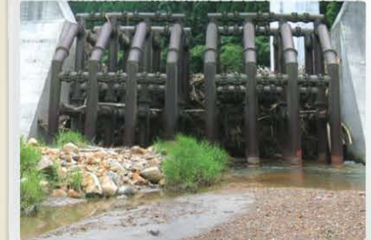
Debris-straining structure (grid structure) in Japan - Photo courtesy of Kobe Steel Limited
