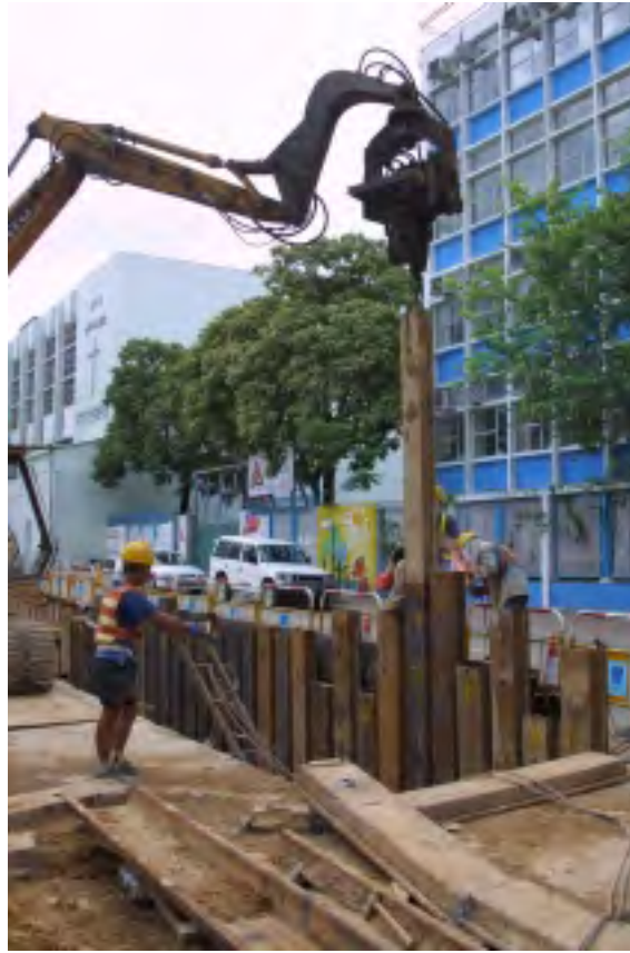
Plate A9 – Installation of support from outside the trench
