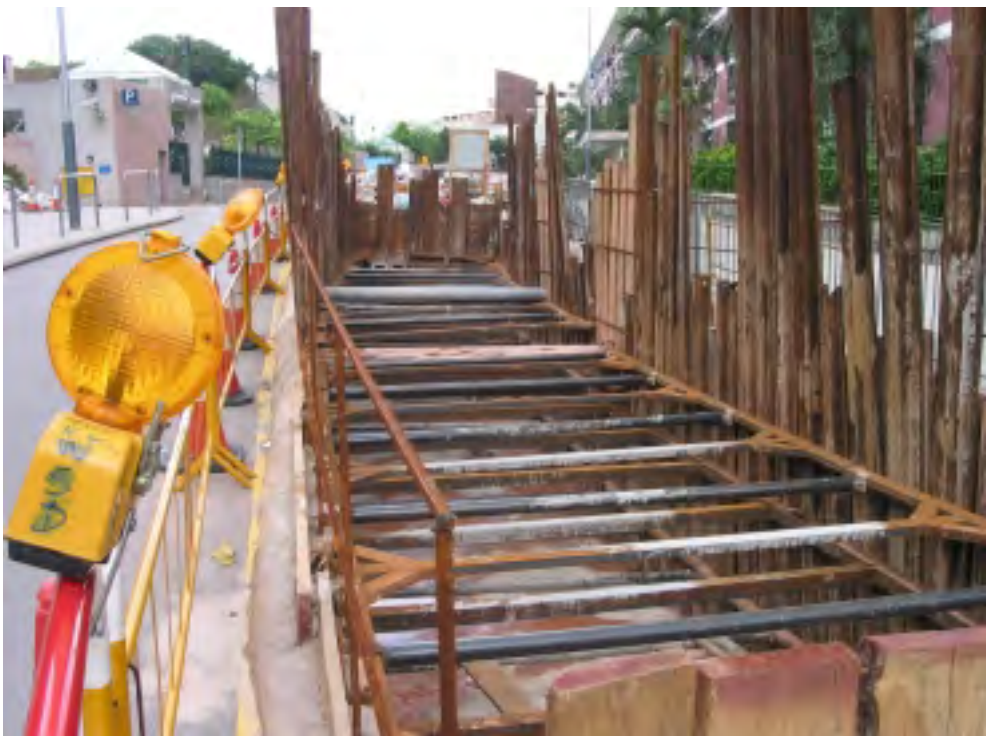
Plate A4 – Steel sheet pile support
