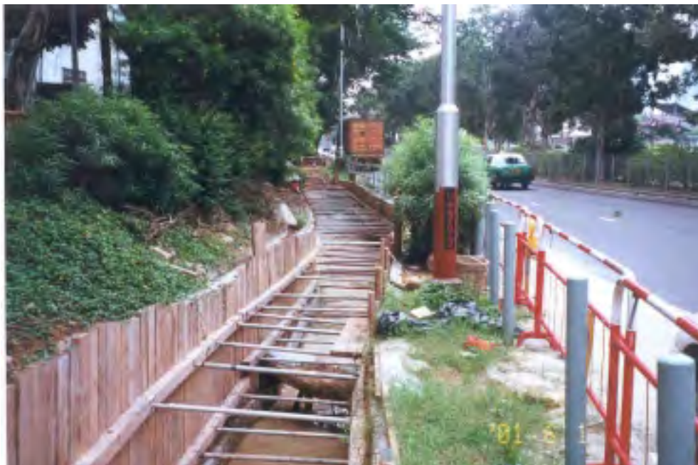
Plate A2 – Timber support with two layers of struts
