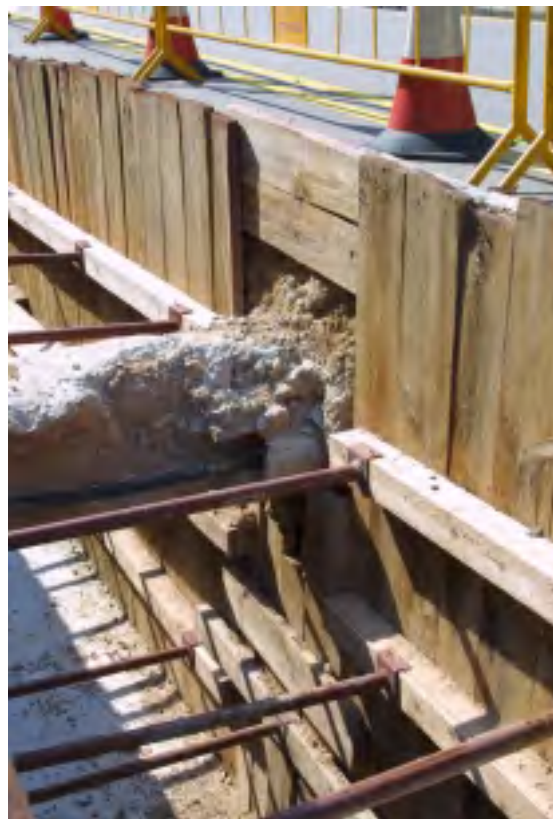
Plate A8 – Timber support provided in areas surrounding existing crossing services
