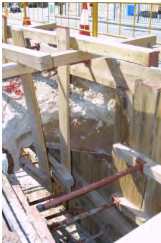
Plate A6 – Timber support provided in areas surrounding existing crossing services
