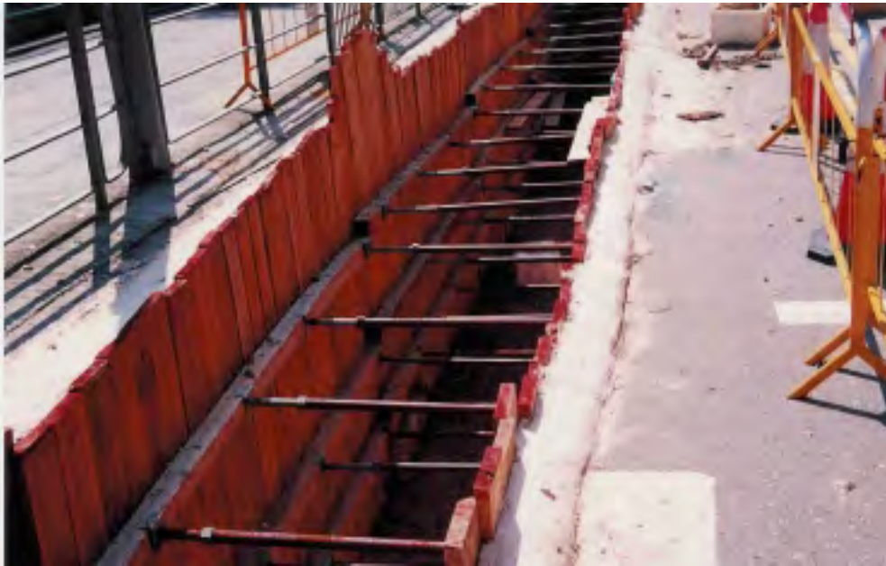
Plate B5 – Timber support protruding above ground with cement mortar wedge applied to prevent surface runoff
