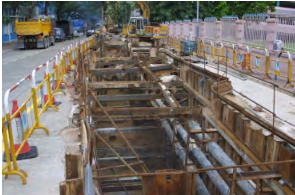
Plate A5 – Steel sheet pile support
