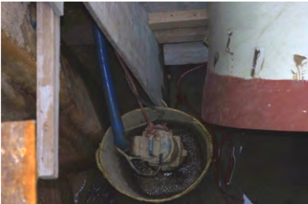
Plate B6 – Pumping provided
