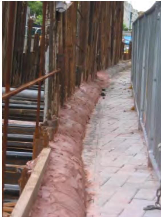
Plate B4 – Sheet piles protruding above ground with cement mortar wedge applied to prevent surface runoff
