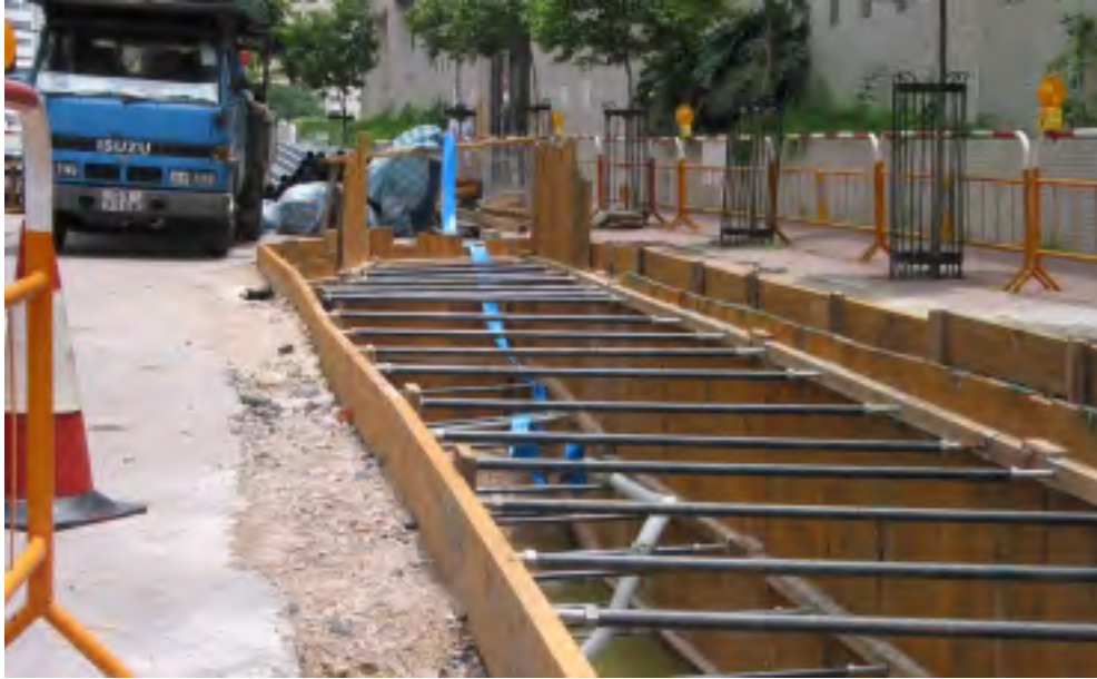
Plate A3 – Timber support for deeper excavation
