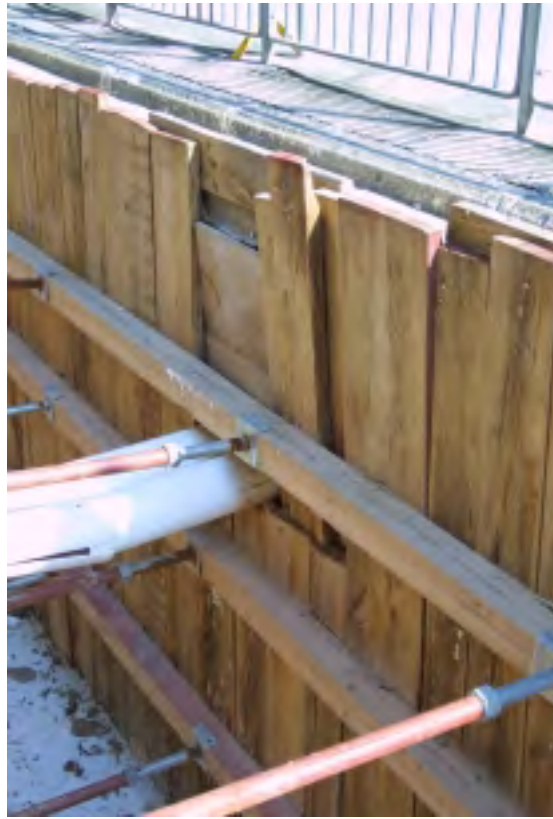
Plate A7 – Timber support provided in areas surrounding existing crossing services
