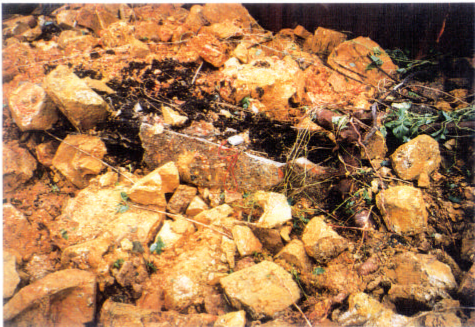
Plate 5 - Blocked Surface Drainage Channel in the Landslide Debris (Photograph Taken on 13 August 1995. See Figure 21 for Location)
