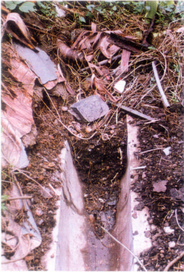
Plate 4 - Blocked Surface Drainage Channel on the Unfailed Section of the Cut Slope (Photograph Taken on 10 October 1995. See Figure 21 for Location)
