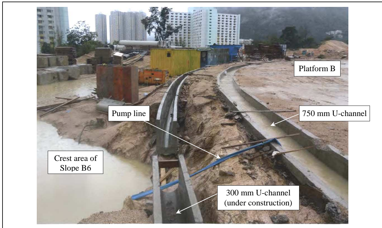
Plate 19 Standby Pump Provided at the Crest Area of Slope B6 (Photograph taken on 22 May 2013)
