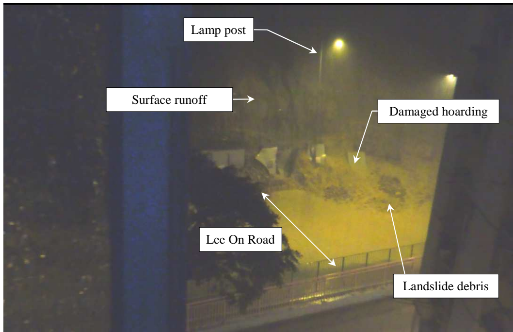
(a) Initial Stage of Failure (Exact Time Unknown)
