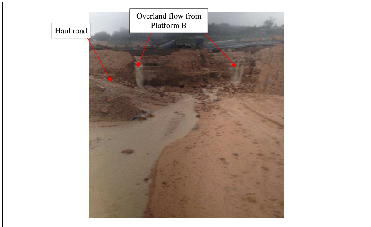
Plate 17 Significant Overland Flow from Platform B between Sand Traps ST15 and ST16 (Photograph taken around 9:00 a.m. on 22 May 2013)
