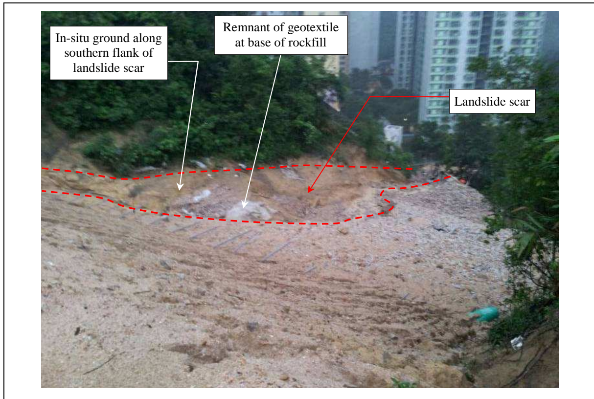
Plate 9 Landslide Scar at Slope B6 (Photograph taken on 22 May 2013)
