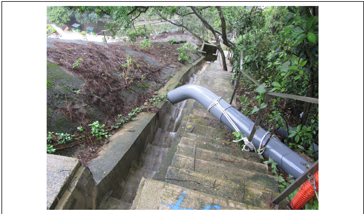
Plate 18 Discharge of 225 mm Diameter UPVC Pipe to Surface Drainage System of Slope 11NE-D/C30 (Photograph taken on 25 May 2013)
