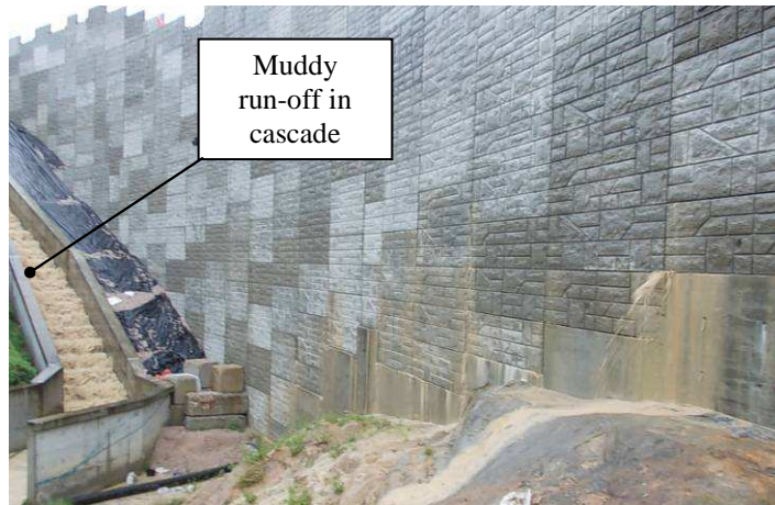
(a) Muddy Seepage at Bottom of Dummy Panels at Bay 3 (Photograph taken on 18 May 2012)
