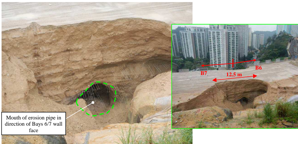
(c) Condition of Sinkhole (Photographs taken on 22 May 2013)
