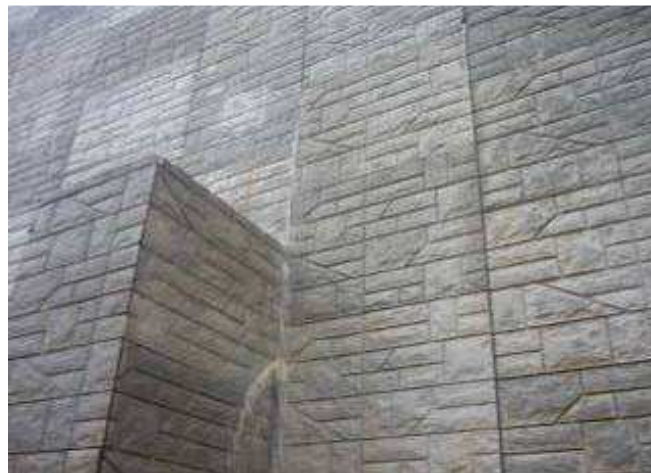
(c) Seepage at Bay 4 prior to July 2012 Incident (Photograph taken on 23 July 2012)
