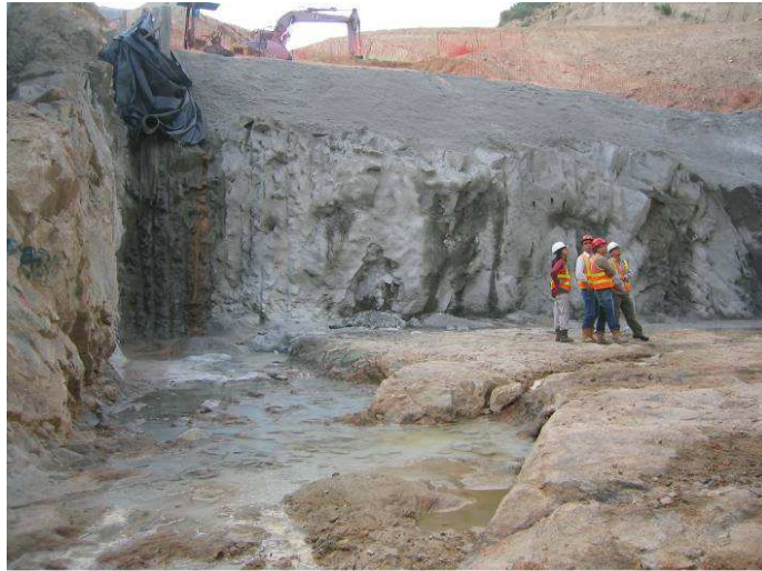
(a) Seepage Flow Rate of 0.84 \ell/s Recorded at Bay 1 in April 2010
