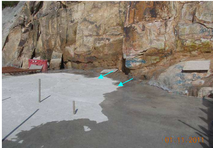
(b) Seepage from Weak Seam at Temporary Cut at Bay 3 and Bay 4 (Photograph taken on 1 November 2011)
