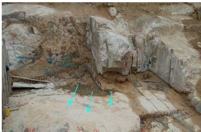
(c) Seepage from Weak Seam at Bay 7 (Photograph taken on 1 December 2011)
