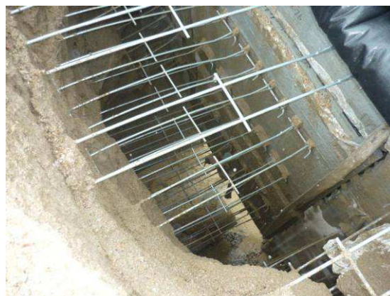
(c) Soil Loss behind Panels
