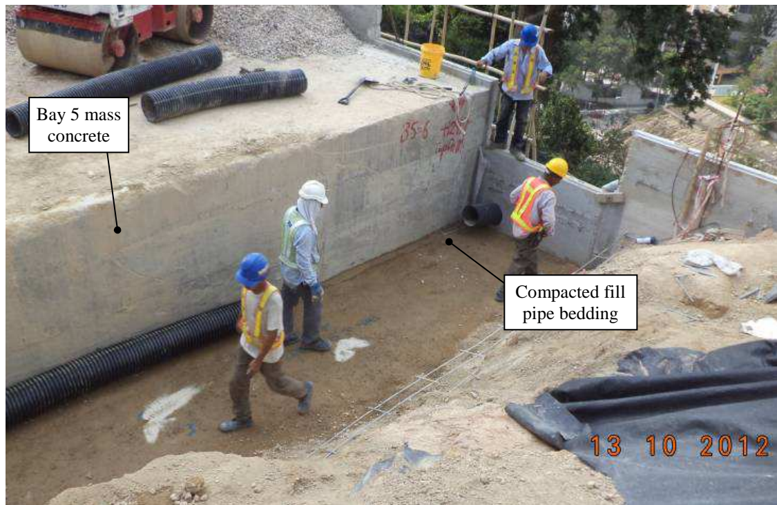
(a) Installation of Subsoil Drain Pipe at Bay 4 (Photograph taken on 13 October 2012)
