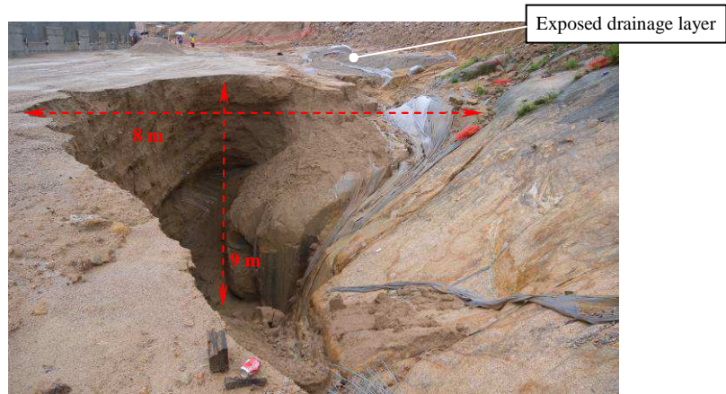
(b) Formation of Sinkhole in Backyard of Bays 6/7 (Photograph taken on 22 May 2013)
