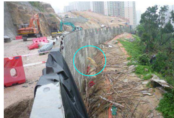
(d) Muddy Outflow from Subsoil Drain Pipe at Bay 9 (Photograph taken on 25 July 2012)
