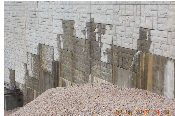
(b) Seepage at Bottom of Dummy Panels at Bay 3 (Photograph taken on 6 May 2013)
