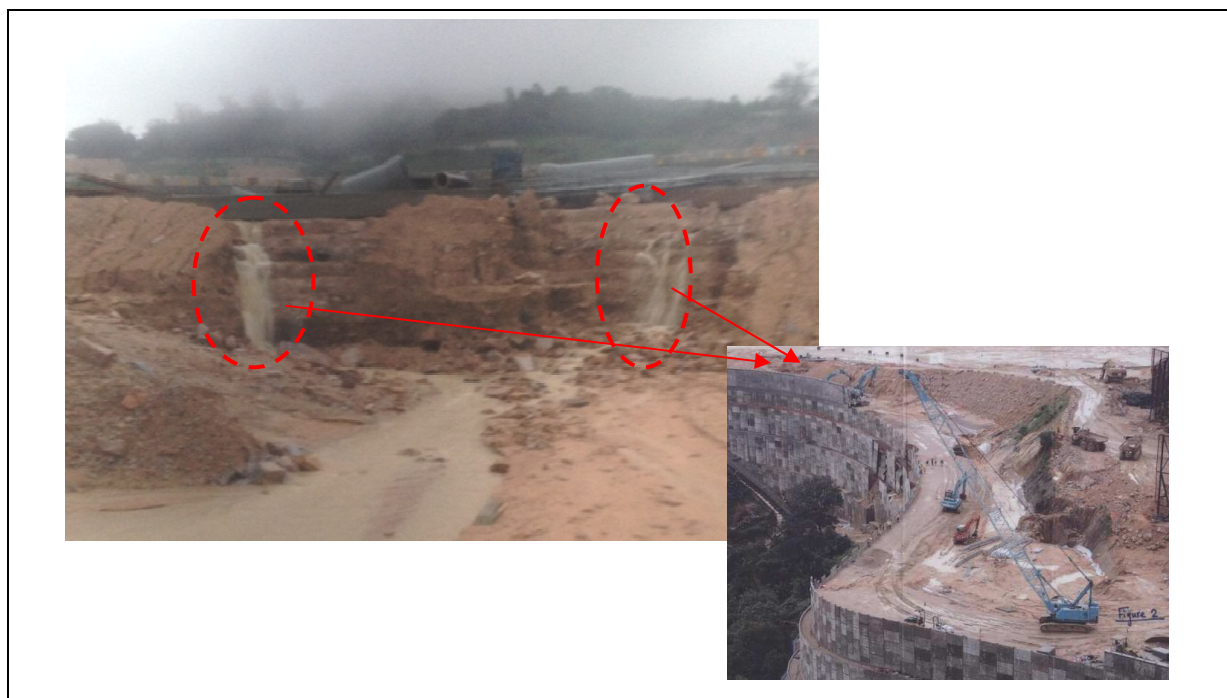
Plate 12 Significant Overland Flow from Platform B between Sand Traps ST15 and ST16 towards the Back of Wall R22 (Photographs taken around 9:00 a.m. on 22 May 2013)
