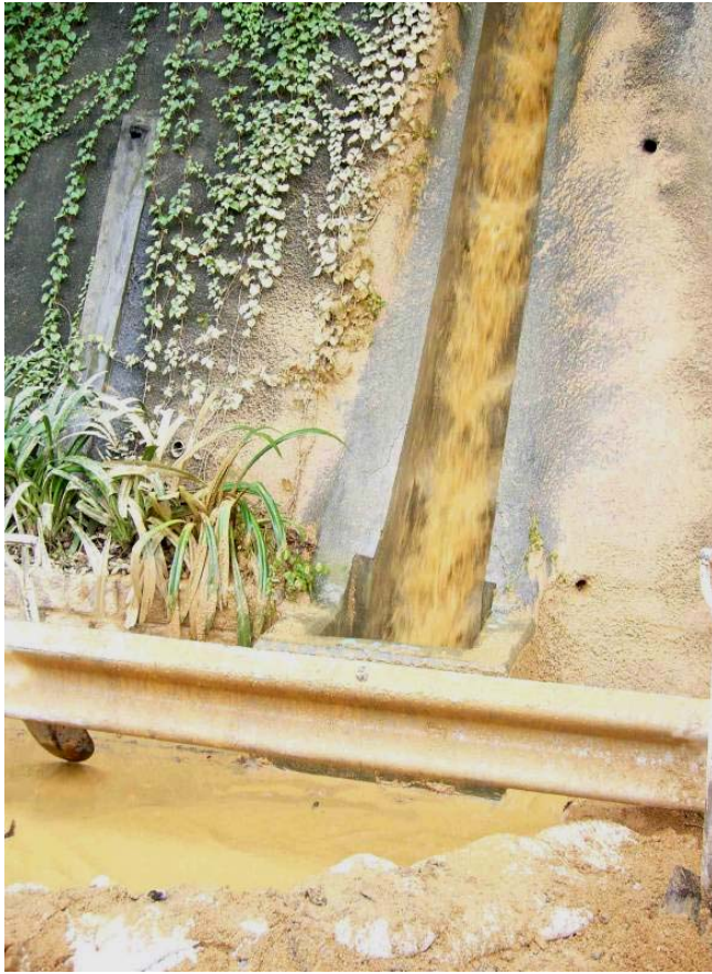
Plate 3 - Muddy Water Flow from Stepped Channel of Slope No. 7SW-D/C2 (Photograph taken on 23 August 2005)
