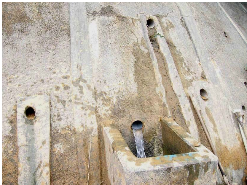
Plate 4 - Water Flow from Raking Drains of Slope No. 7SW-D/C2 (Photograph taken on 23 August 2005)
