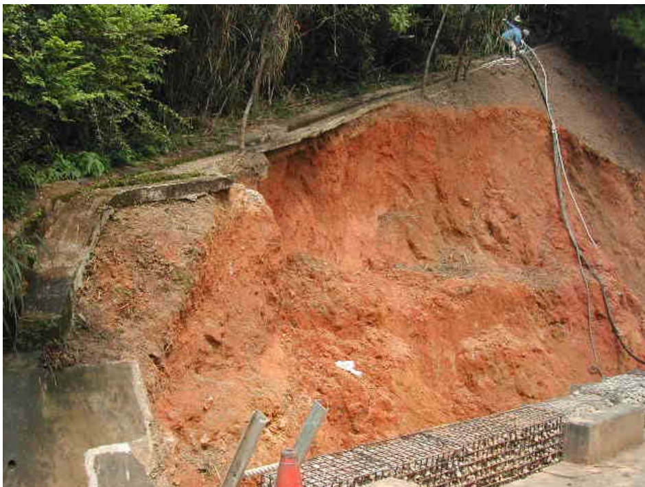
Plate 12 - General View of the Landslide on Slope No. 6SE-B/CR249 (Photograph taken by WSD on 31 August 2005)
