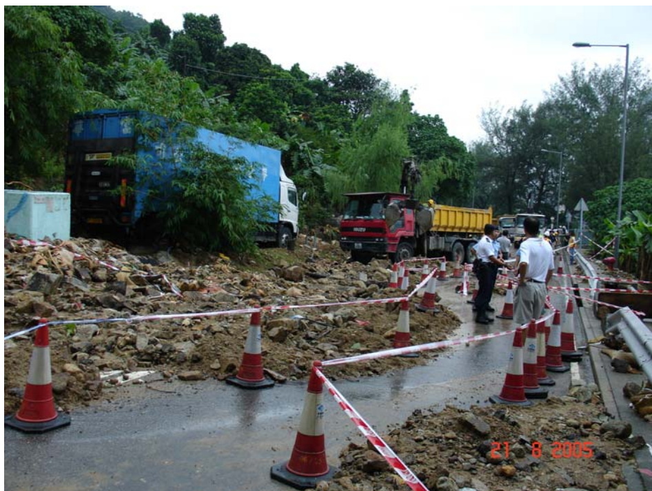
Plate 2 - Debris Deposited on Route Twisk Looking Southeast (Photograph taken by HyD on 21 August 2005)
