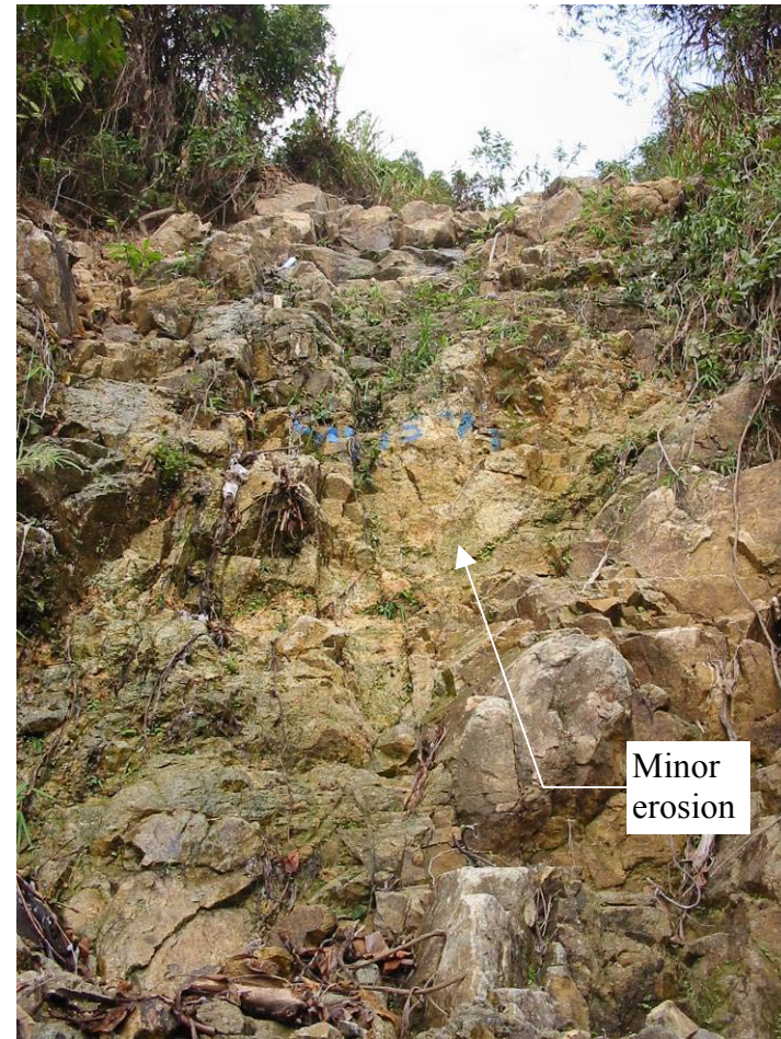
Plate 16 - View of the Steeper Section of the Debris Flood Trail between CH 49 and CH 57 (Photograph taken on 22 February 2006)
