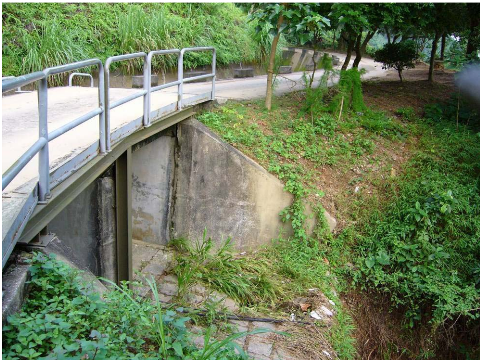
Plate 6 - View of Overflow Weir SMOF-28 (Photograph taken on 26 August 2005)
