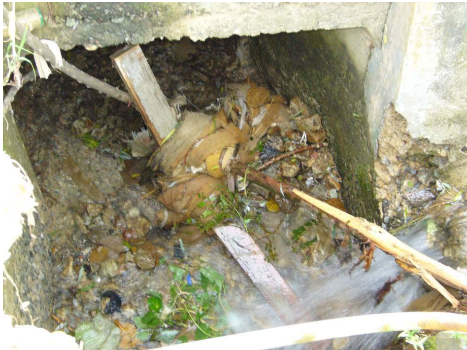
Plate 8 - Inlet of 1.4 m x 1.4 m Cross-road Culvert (Photograph taken on 26 August 2005)
