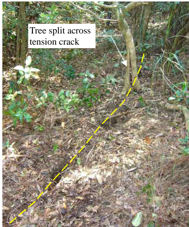
Plate 25 - One of a Series of Stepped Tension Cracks on the Western Flank of the Distressed Hillside (Photograph taken on 10 March 2006)
