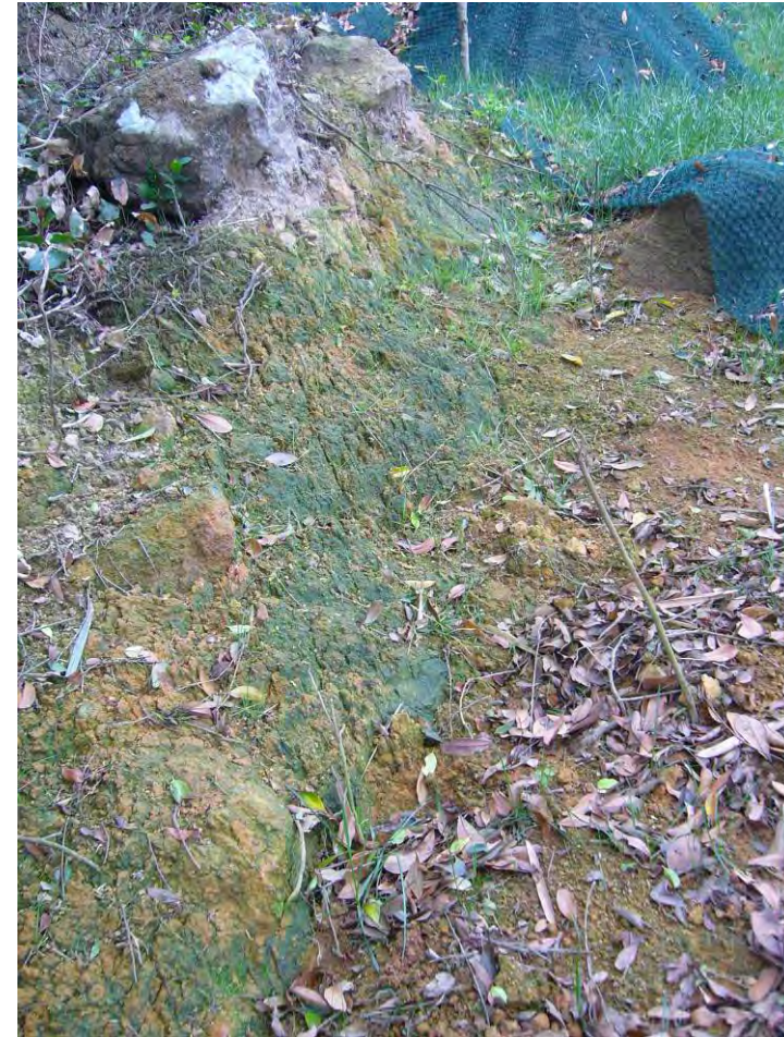
Plate 10 - Upslope Extension of the Lateral Tension Crack Immediately West of the August 2005 Landslide above the Main Scarp (Photograph taken on 10 March 2006)
