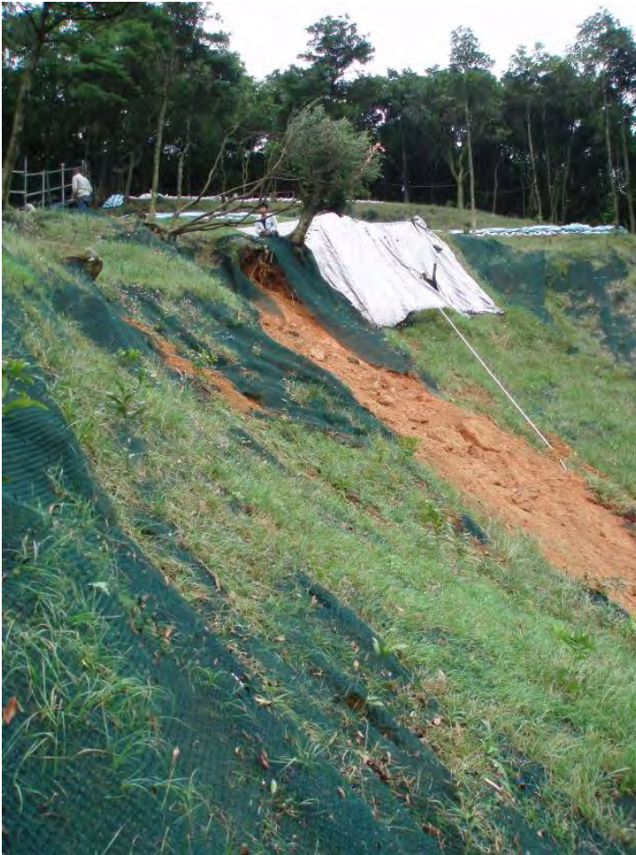
Plate 7 - Displaced Mass below Stepped Tension Cracks on Eastern Flank of the August 2005 Landslide Source (Photograph taken on 5 June 2006)
