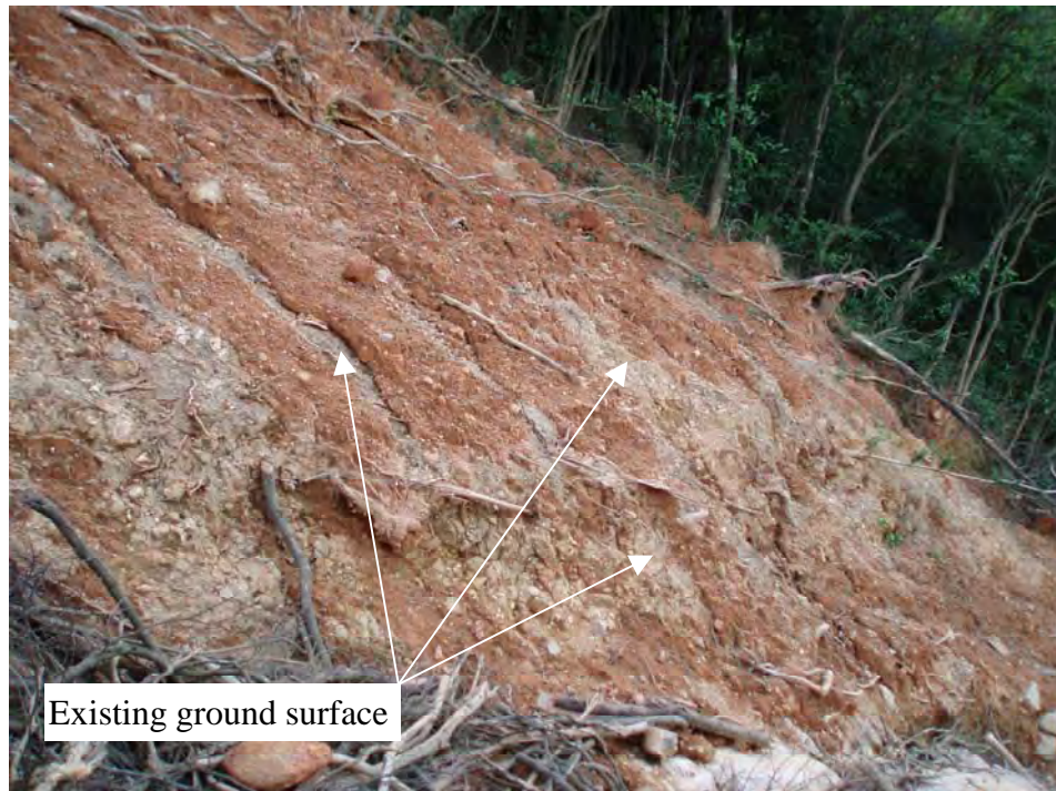
Plate 15 - Existing Ground Surface Exposed in the Base of the Debris Trail (Photograph taken on 25 May 2005)
