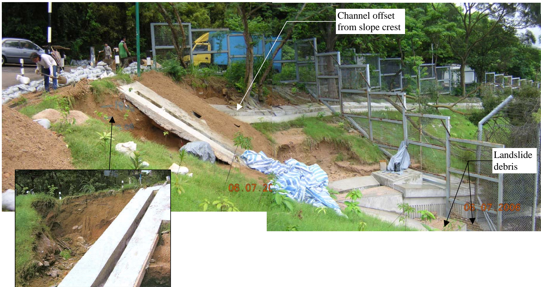
Plate 1 - General View of the 9 June 2006 Washout Incident on Slope No. 11NW-B/FR60 (Photograph taken by Arch SD on 6 July 2006)
