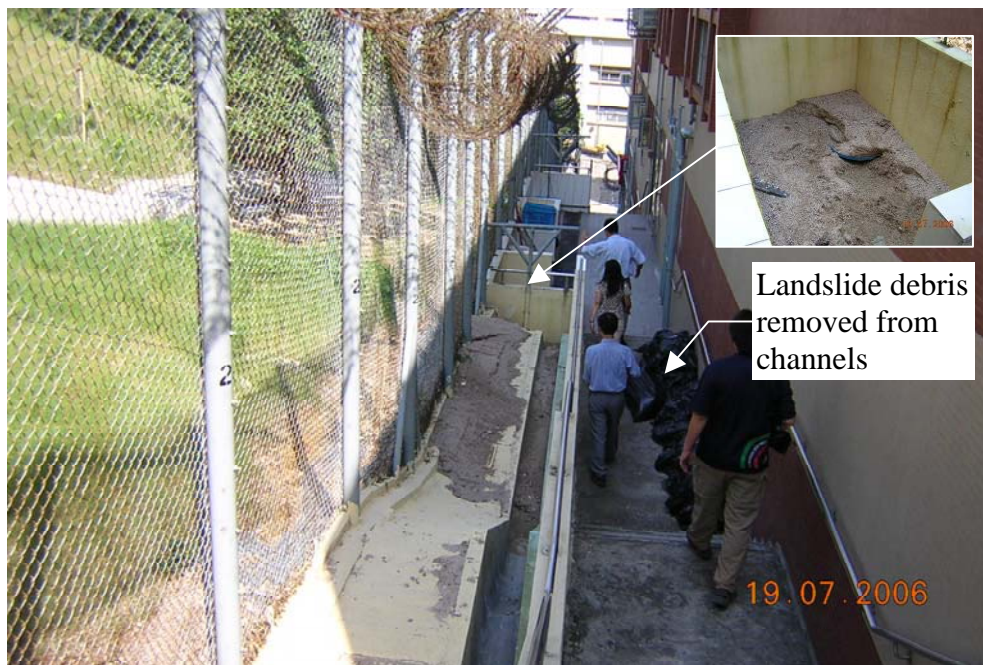
Plate 11 - Landslide Debris Deposited along the Toe Channels of Slope No. 11NW-B/FR60 (Photograph taken by Arch SD on 19 July 2006)
