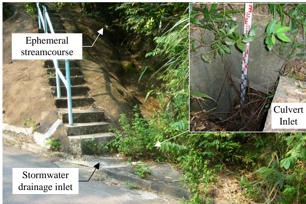
Plate 8 - View of the Ephemeral Streamcourse at East End of Slope No. 11NW-B/C506 and the Drainage Inlet of the Cross-road Culvert (Photograph taken on 20 September 2006)
