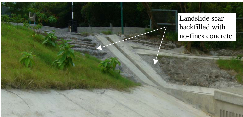
Plate 13 - Urgent Repair Works for the July 2006 Washout (Photograph taken on 18 August 2006)
