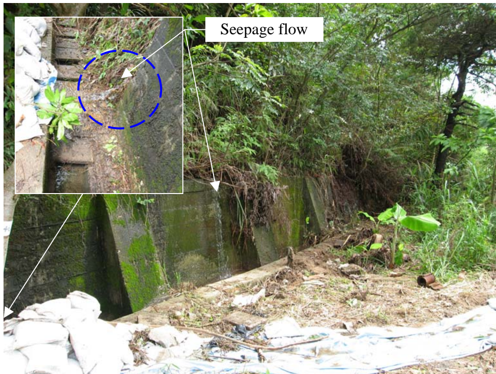
Plate 15 - Counterfort Wall on Slope No. 7NE-D/C178 with Active Seepage (Photograph taken by Lands D on 13 June 2006)
