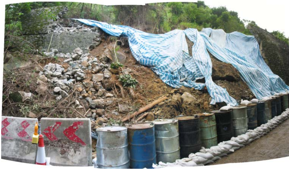
Plate 9 - View of the Landslide Debris and Masonry Wall Fragment (Photograph taken by Lands D on 5 June 2006)
