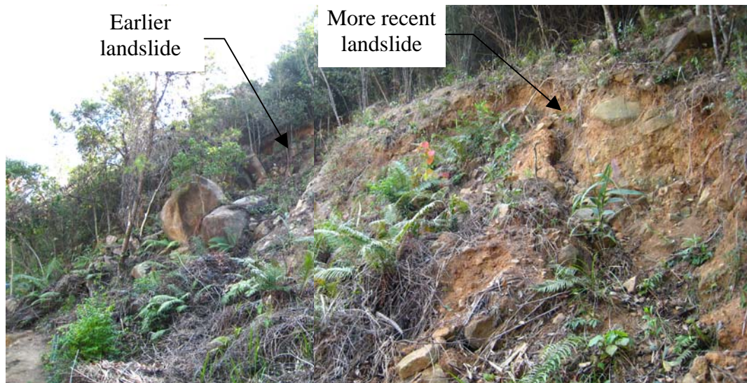
Plate 14 - Major Landslide on Slope No. 7NE-D/C178 (Photograph taken on 7 February 2007)
