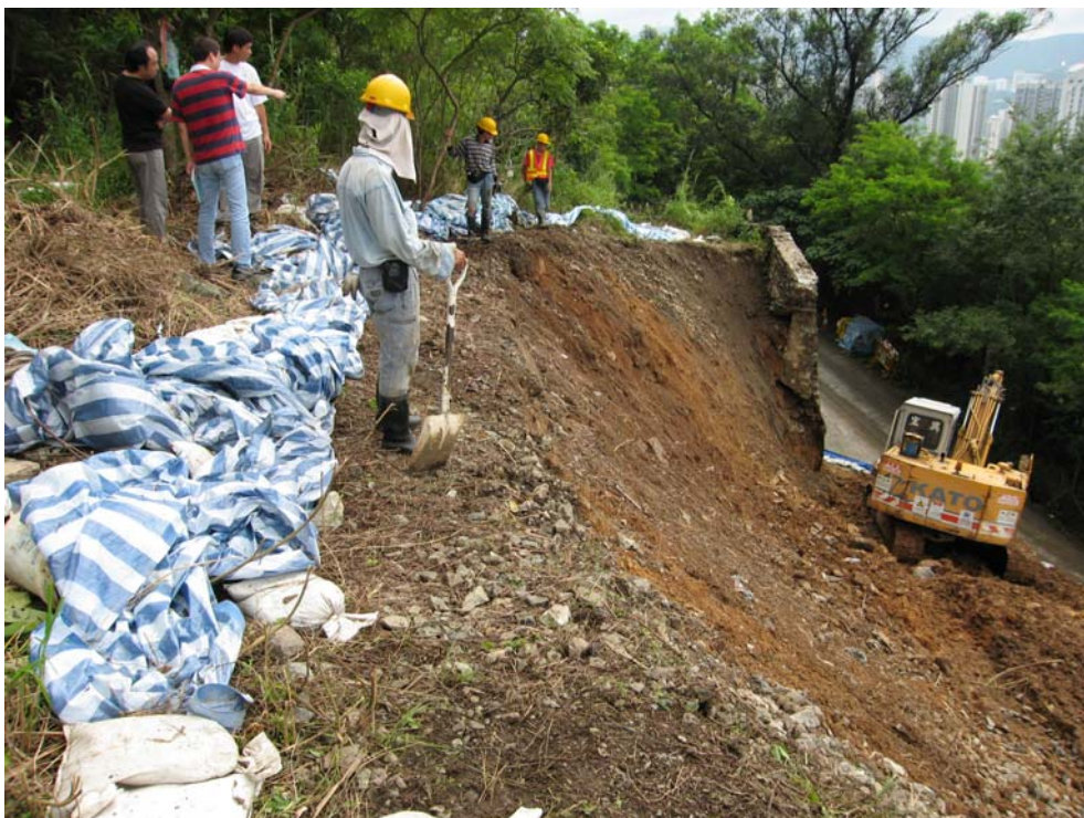
Plate 10 - View of the Exposed Wall Stem during the Urgent Repair Works (Photograph taken by Lands D on 13 June 2006)
