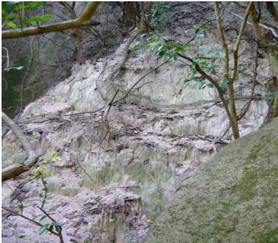
Plate 10 - Accumulation of Possible Debris from Previous Failures (Photograph taken on 13 April 2007)
