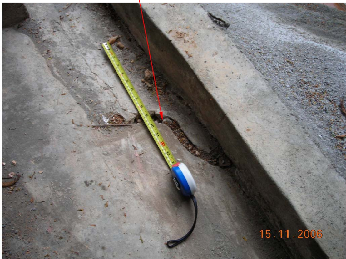
Plate 8 - Close View of Example of Cracking in Crest U-channel (Photograph taken on 15 November 2006)
