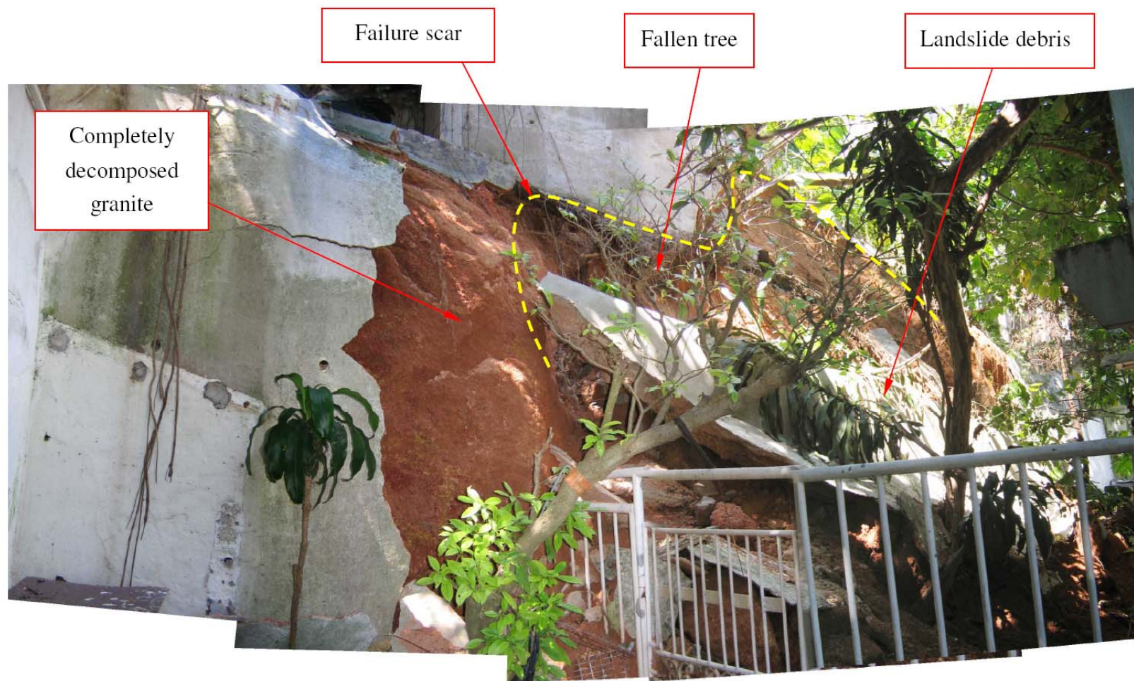
Plate 1 - View Northeast across Slope No. 14NE-B/CR180 above No. 49 Po Wah Yuen Showing Landslide Scar (Photograph taken by GEO on 20 July 2006)
