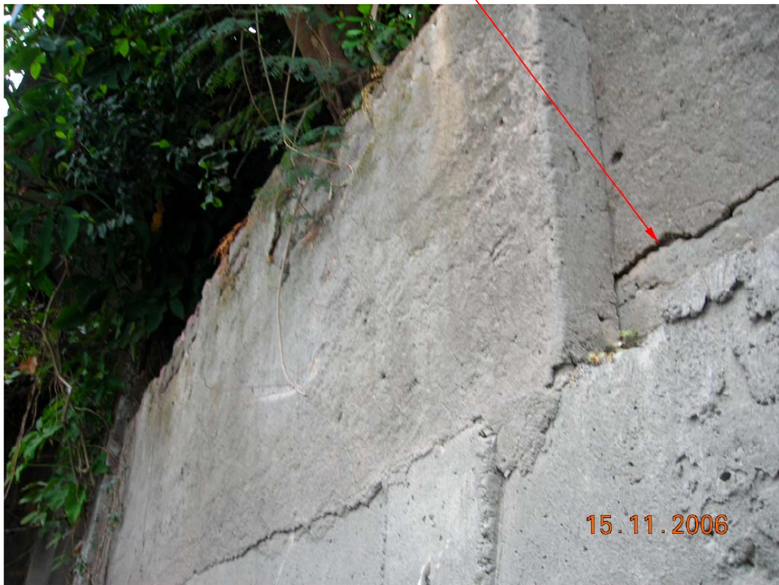
Plate 9 - Close View of Retaining Wall at Crest of Slope No. 14NE-B/CR180 above No. 49 Po Wah Yuen Showing Existing Cracks (Photograph taken on 15 November 2006)
