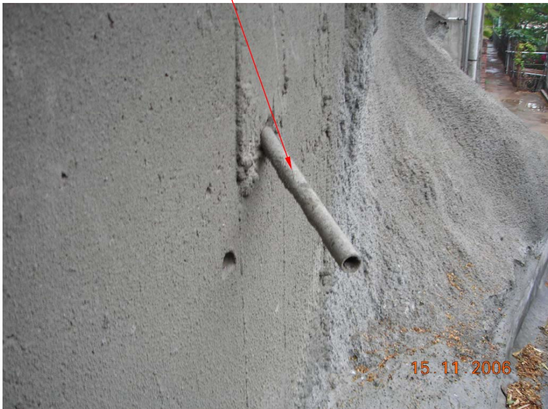
Plate 11 - Close View of 19 mm Diameter Galvanised Iron Pipe Protruding from Retaining Wall at Crest of Slope No. 14NE-B/CR180 above No. 49 Po Wah Yuen (Photograph taken on 15 November 2006)
