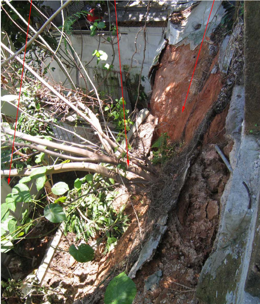
Plate 4 - View West across Slope No. 14NE-B/CR180 above No. 49 Po Wah Yuen Showing 16 July 2006 Landslide Scar and Mature Tree with Chunam Surround to Root Mass Remaining within Scar (Photograph taken by GEO on 20 July 2006)
