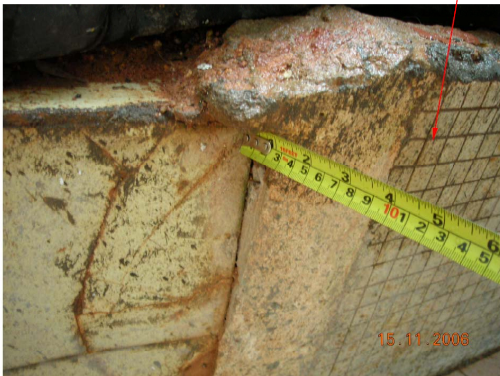
Plate 6 - Close View of Toe Planter Wall Showing Bulging and Cracking (Photograph taken on 15 November 2006)
