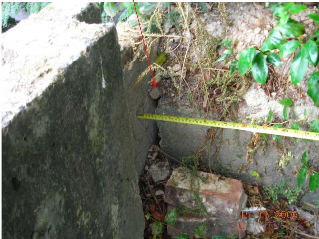
Plate 10 - Close View of Crest Area of the Retaining Wall at Crest of Slope No. 14NE-B/CR180 above No. 49 Po Wah Yuen Showing Gaps between Concrete Elements (Photograph taken on 15 November 2006)
