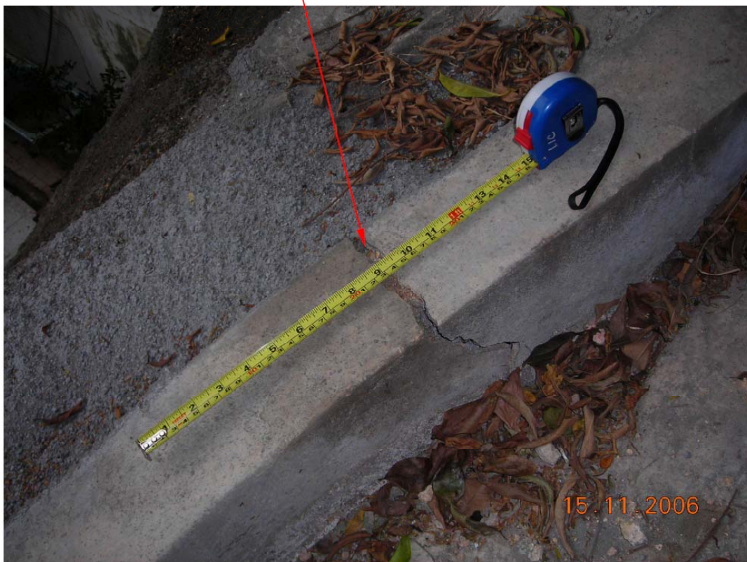
Plate 7 - Close View of Example of Cracking in Crest U-channel (Photograph taken on 15 November 2006)
