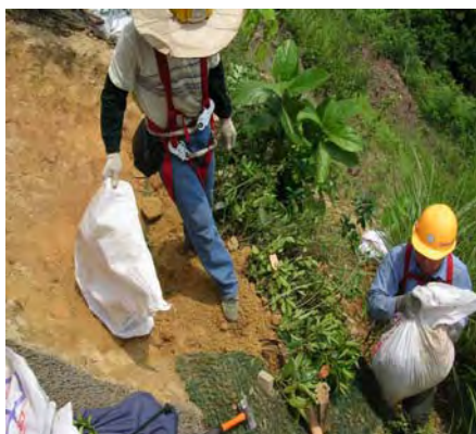
Plate 44 - Placing and Compacting Soil Fill on the Live Gully Repair (Cloudy Hill)
