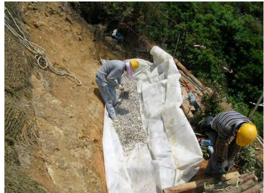
Plate 51 - Placing Rock Filter with Geotextile on Live Cribwall Platform (Cloudy Hill)
