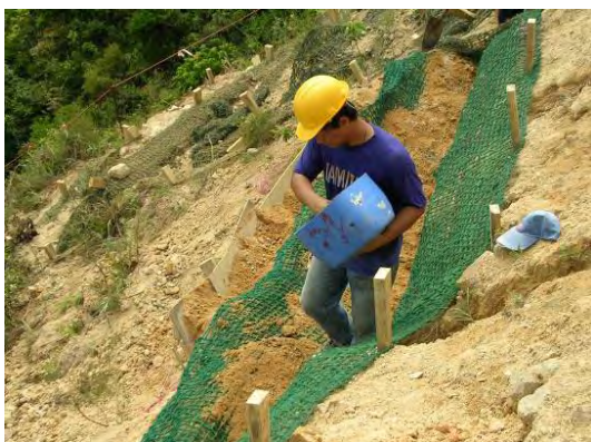
Plate 28 - Placing Soil Fill with Additives on Lined Hedgelay Bench (Cloudy Hill)
