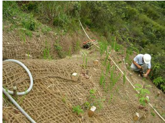
Plate 49 - Completion of Berm Prior to Installation of Live Stakes/Pit Plants (Cloudy Hill)
