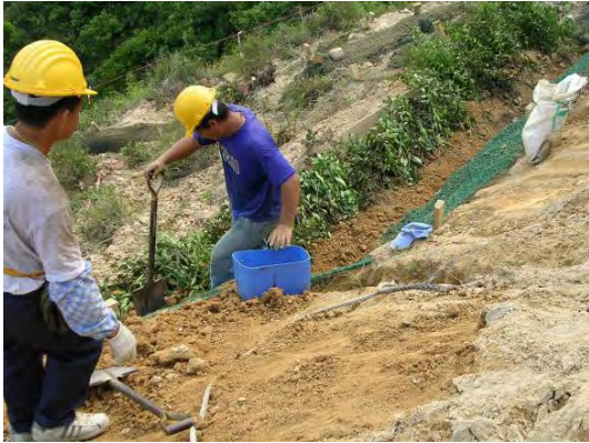
Plate 23 - Soil Backfilling over the Completed Brushlayer (Cloudy Hill)
