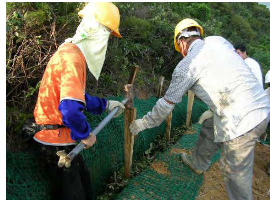
Plate 11 -Driving Dead Stakes through the Installed Live Fascine (Cloudy Hill)
