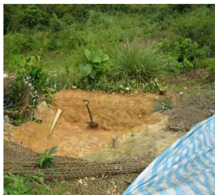
Plate 45 - Completion of One Layer of Live Gully Repair (Cloudy Hill)
