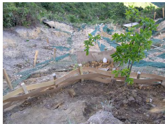
Plate 58 - Completed Bender Fence Prior to Backfilling with Soil (Cloudy Hill)
