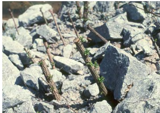
Plate 65 - Newly Installed Joint Planting in Kentucky, USA (Sotir, 1994)
