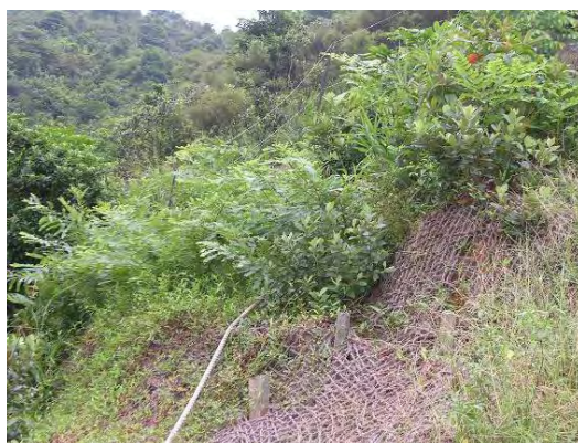
Plate 61 - Established Vegetation in Bender Fence after One Year (Cloudy Hill)
