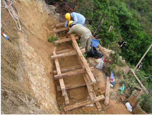
Plate 54 - Soil Fill and Live Branch Cuttings/Rooted Plants in Live Cribwall (Cloudy Hill)
