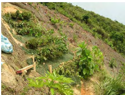
Plate 46 - Completed Live Gully Repair (Cloudy Hill)
