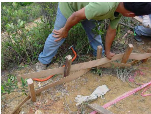
Plate 57 - Weaving Wooden Boards around Wooden Poles for Bender Fence (Cloudy Hill)
