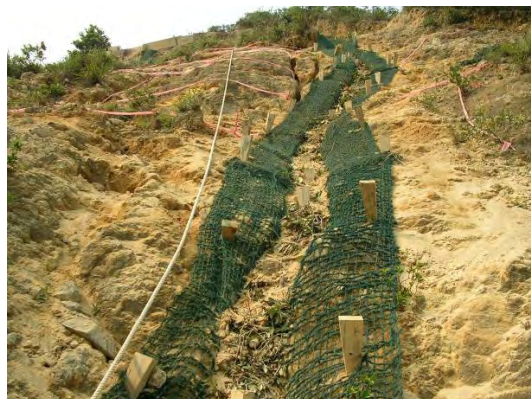
Plate 13 - Completed Live Fascines (Cloudy Hill)
