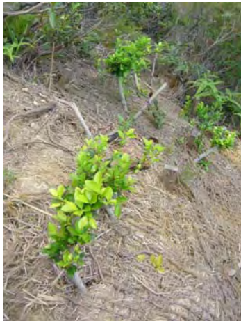
Plate 48 - Established Live Stakes in Tension Crack Repair after Six Months (Sham Wat)
