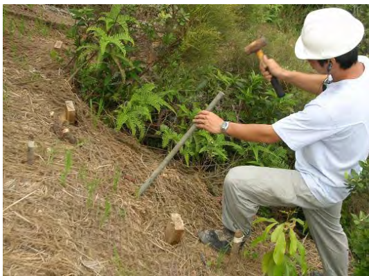
Plate 2 - Driving a Steel Bar to Ream a Hole for a Live Stake (Cloudy Hill)
