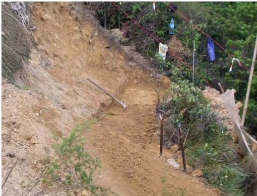
Plate 50 - Excavating Platform for Live Cribwall (Cloudy Hill)
