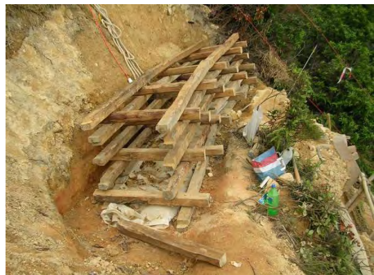
Plate 53 - Completed Timber Framework for Live Cribwall (Cloudy Hill)
