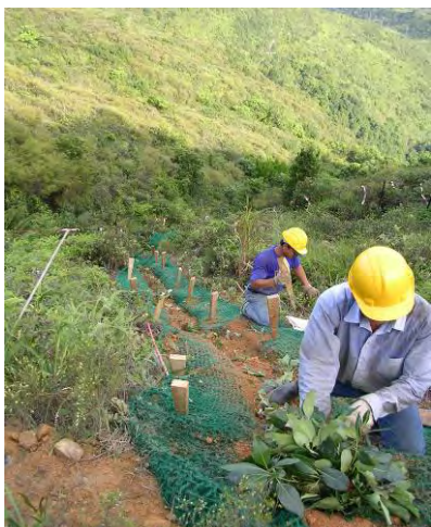
Plate 12 - Placing Soil Fill with Additives over Secured Live Fascine (Cloudy Hill)
