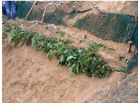
Plate 24 - Completed Brushlayer (Cloudy Hill)
