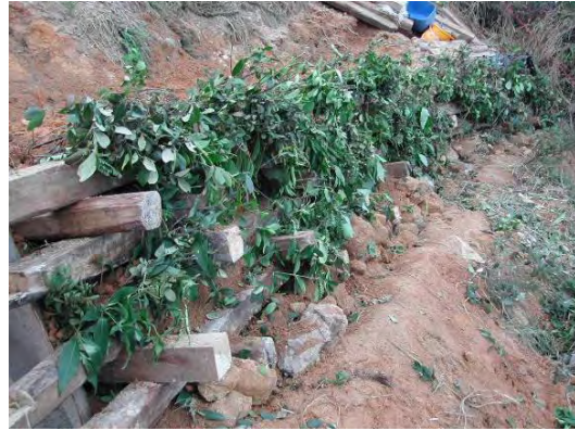
Plate 55 - Completed Live Cribwall (Cloudy Hill)
