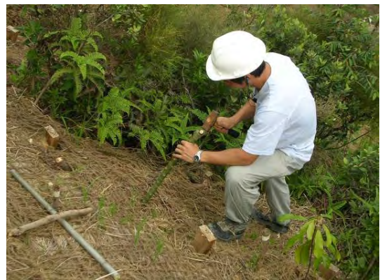
Plate 3 - Installation of an Harvested Live Stake (Cloudy Hill)
