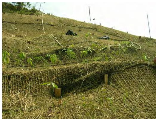
Plate 60 - Completed Bender Fence with Backfill and Erosion Control Mat (Cloudy Hill)
