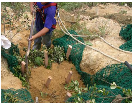
Plate 37 - Placing and Compacting Soil Fill with Additives over Branchpacking (Cloudy Hill)
