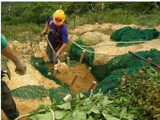
Plate 35 - Placing Soil Fill with Additives onto the Branchpacking Platform (Cloudy Hill)
