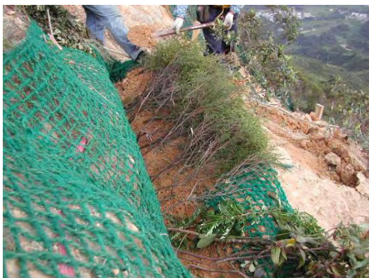
Plate 21 - Overlapping Arrangement of Live Branch Cuttings for Brushlayer (Cloudy Hill)
