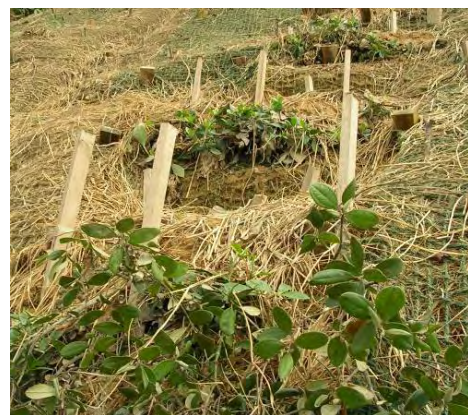
Plate 38 - Completed Branchpacking Installation (Cloudy Hill)
