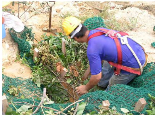
Plate 36 - Placing Live Branch Cuttings/Rooted Plants for Branchpacking (Cloudy Hill)
