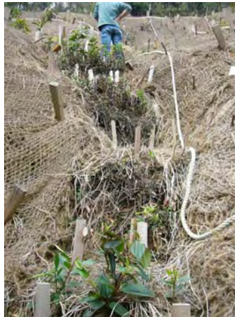
Plate 39 - Established Branchpacking after One Year (Cloudy Hill)
