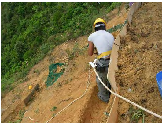
Plate 26 - Hedgelay Bench Excavation (Cloudy Hill)
