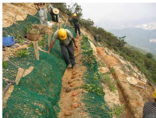
Plate 29 - Laying out Rooted Plants for Hedgelay Installation (Cloudy Hill)
