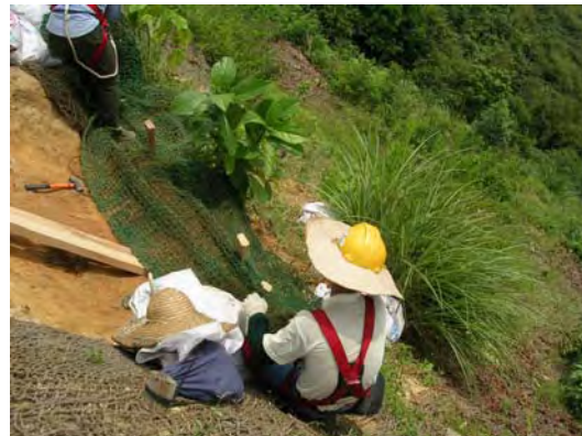
Plate 41 - Installing Degradable Erosion Control Mat at the Base of the Gully (Cloudy Hill)
