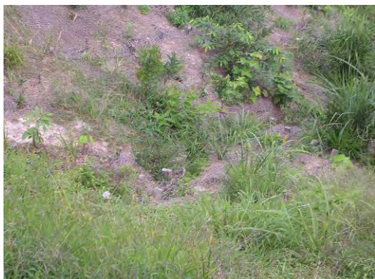
Plate 14 - Established Live Fascine after One Year (Cloudy Hill)
