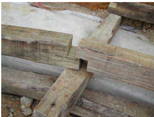
Plate 52 -Placing Live Cribwall Timbers Prior to Installation of Rebar Pins (Cloudy Hill)
