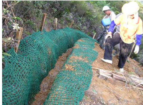
Plate 9 -Placing Soil Fill with Additives in Lined Live Fascine Trench (Cloudy Hill)
