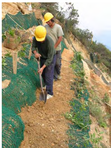
Plate 30 - Placing and Compacting Soil Fill with Additives over Hedgelay (Cloudy Hill)
