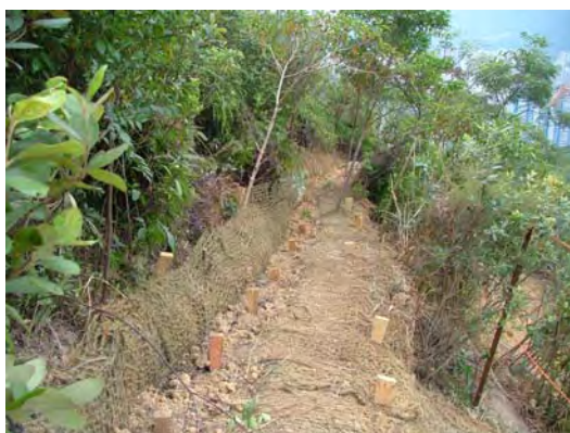
Plate 16 - Completed Pole Drain (Cloudy Hill)
