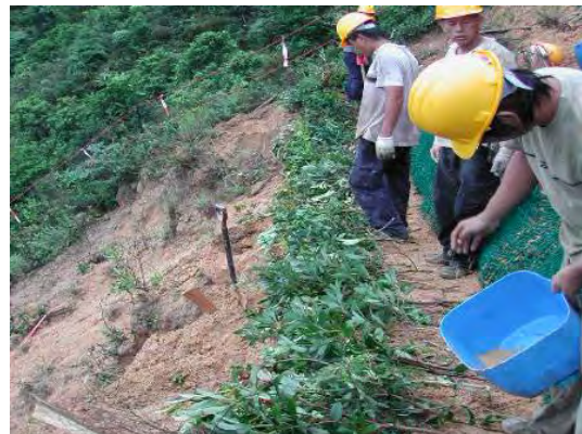
Plate 22 - Placing Soil Fill with Additives over Brushlayer Cuttings (Cloudy Hill)
