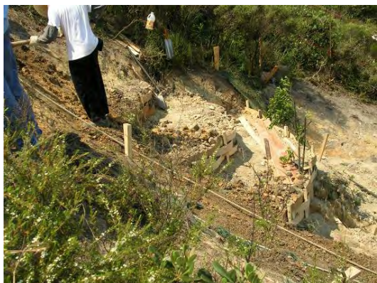
Plate 59 - Soil Backfilling behind Bender Fence (Cloudy Hill)
