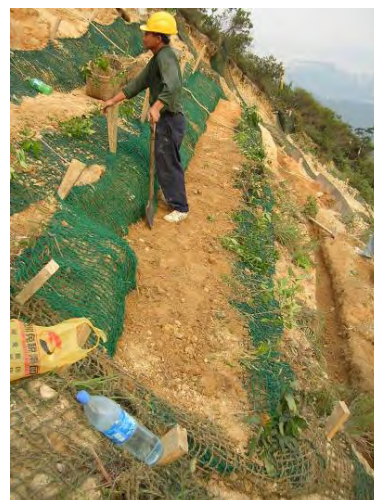
Plate 31 - Completed Hedgelay Installation (Cloudy Hill)
