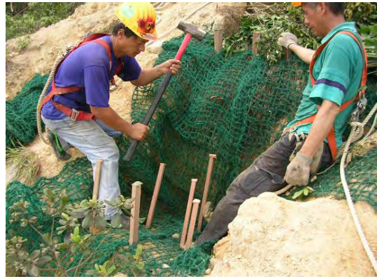
Plate 34 - Lining the Branchpacking Platform with Erosion Control Mat (Cloudy Hill)
