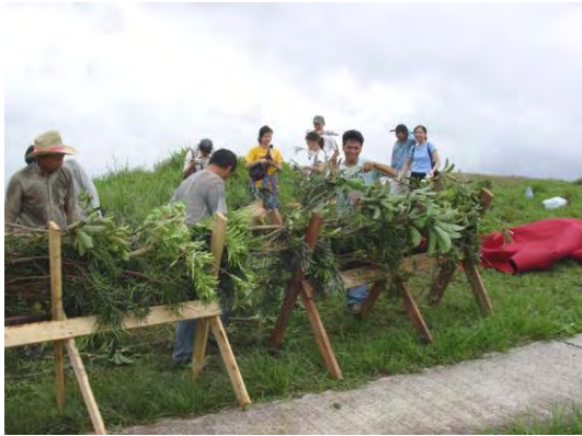
Plate 6 - Live Fascine Fabrication (Cloudy Hill)
