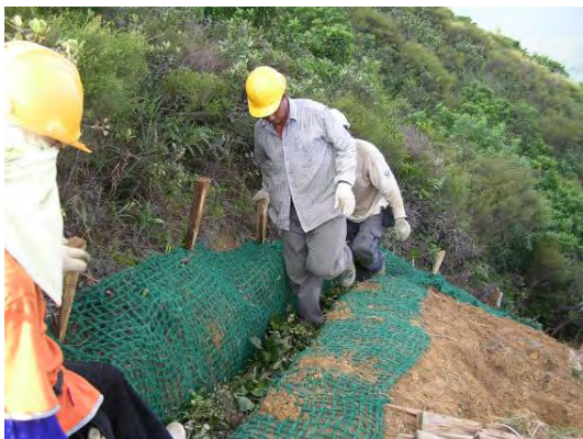
Plate 10 -Installing Live Fascine in Prepared Trench (Cloudy Hill)
