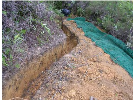
Plate 7 -Excavated Live Fascine Trench (Cloudy Hill)
