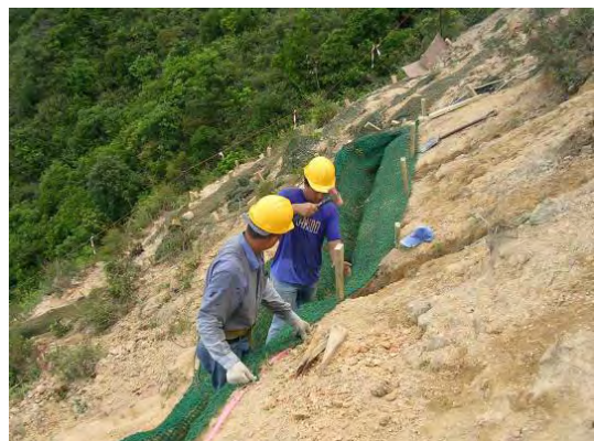
Plate 27 - Lining the Hedgelay Bench with Degradable Erosion Control Mat (Cloudy Hill)
