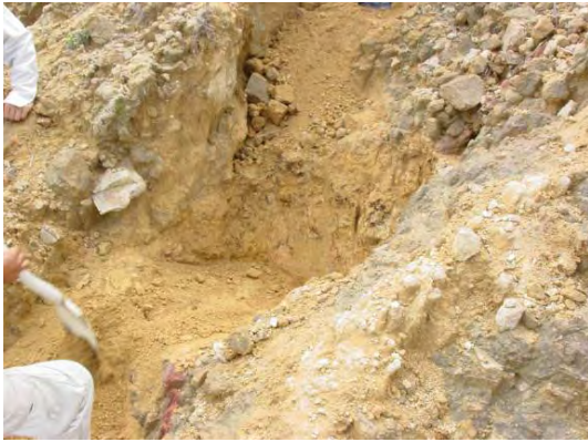
Plate 33 - Excavating a Sub-horizontal Platform for Branchpacking (Cloudy Hill)
