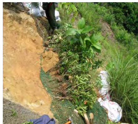
Plate 43 - Live Branch Cuttings/Rooted Plants for Live Gully Repair (Cloudy Hill)
