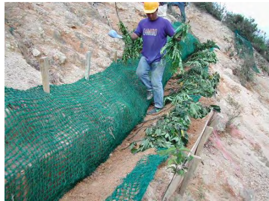
Plate 20 - Placing Live Branch Cuttings and Compacted Soil Fill on the Brushlayer Bench (Cloudy Hill)
