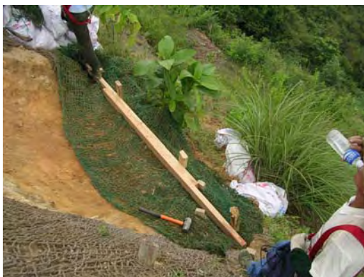
Plate 42 - Installing Wooden Poles for Live Gully Repair (Cloudy Hill)
