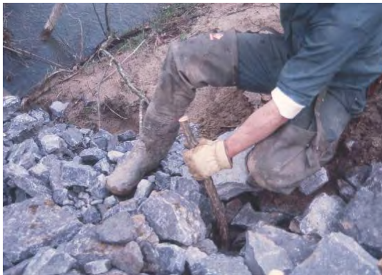
Plate 64 - Joint Planting Installation in Kentucky, USA (Sotir, 1994)
