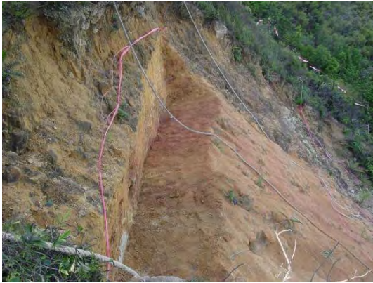
Plate 17 - Brushlayer Bench Excavation (Cloudy Hill)
