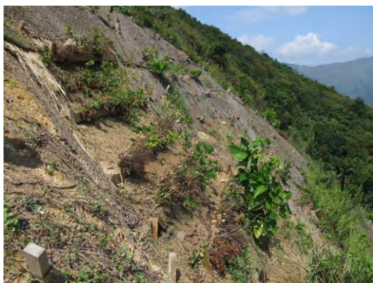
Plate 47 - Established Live Gully Repair after Six months (Cloudy Hill)
