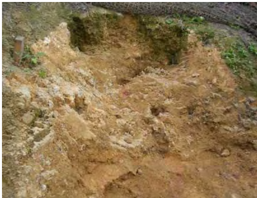
Plate 40 - Erosion Gully Prior to Repair (Cloudy Hill)
