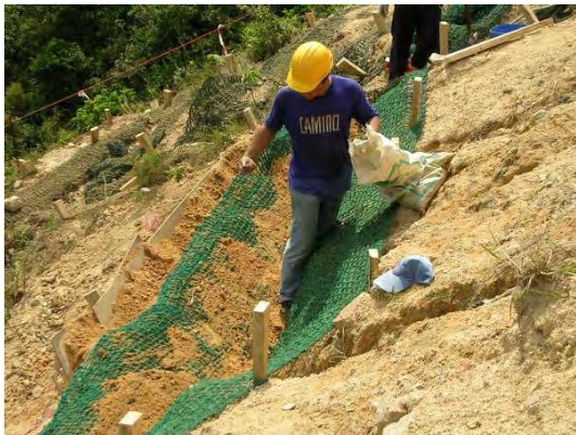
Plate 19 - Placing Soil Fill with Additives on Lined Brushlayer Bench (Cloudy Hill)
