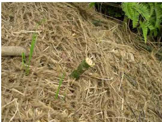
Plate 4 -Installed Live Stake (Cloudy Hill)
