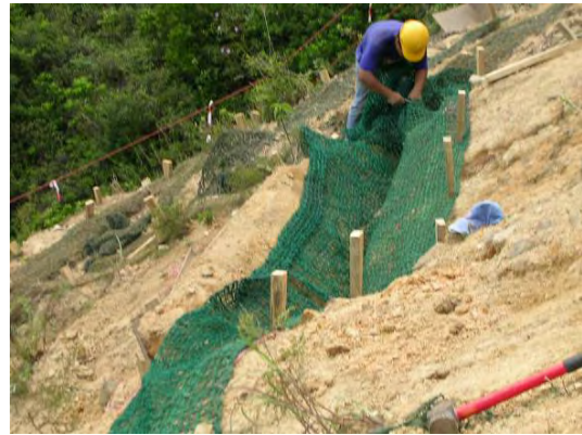
Plate 18 - Lining the Brushlayer Bench with Degradable Erosion Control Mat (Cloudy Hill)
