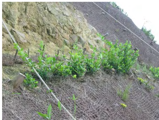
Plate 25 - Established Brushlayer after One Year (Cloudy Hill)
