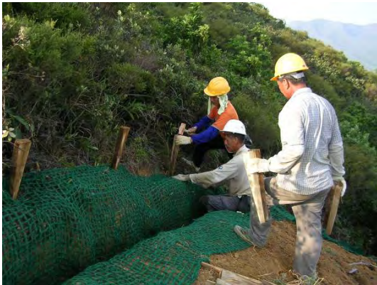
Plate 8 -Lining Live Fascine Trench with Degradable Erosion Control Mat (Cloudy Hill)
