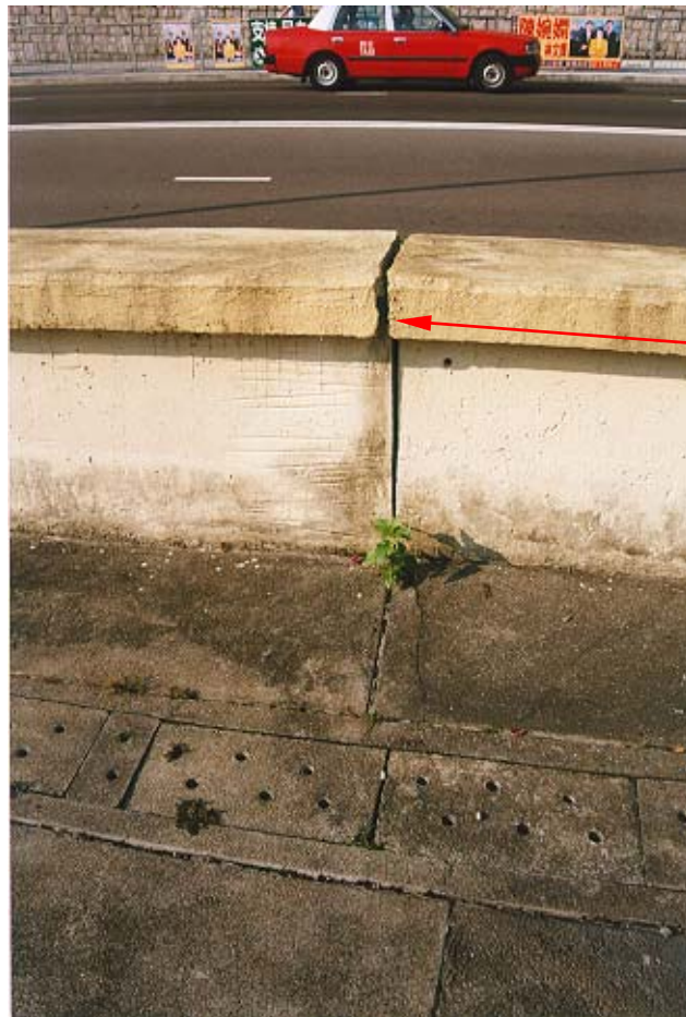
Cracking at Construction Joint in Parapet Wall
