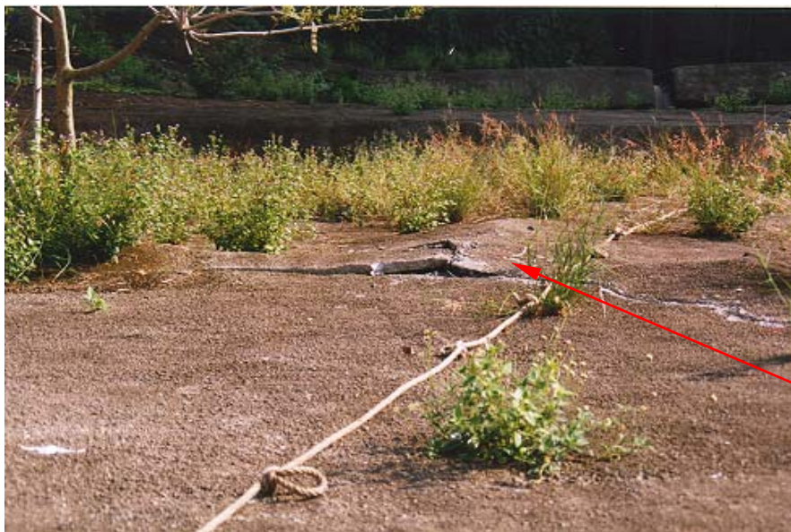
Plate 2 - Distress of Slope No. 11NE-D/F10 at Hiu Kwong Street
