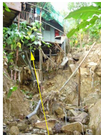
Support of a squatter structure exposed
