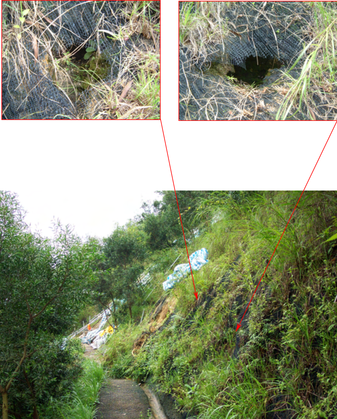
Plate 16 - View of the Erosion Scars on Slope No. 6NE-B/C8 above the Berm (Photograph taken on 14 June 2003)
