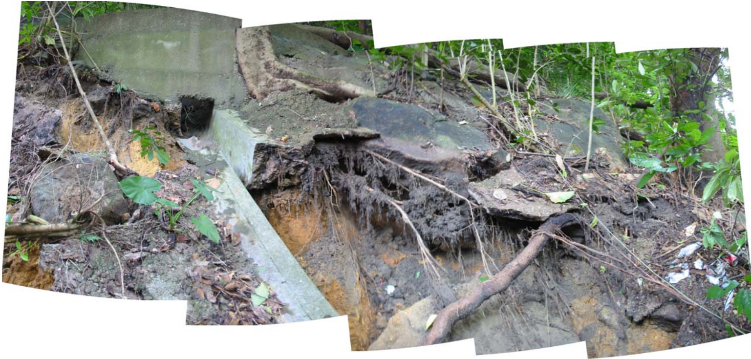
Plate 29 - View of the Minor Slope Displacement adjacent to the Baffle Wall at the Southwestern Part of the Landslide Scar (Photograph taken by FSW on 24 August 2005)
