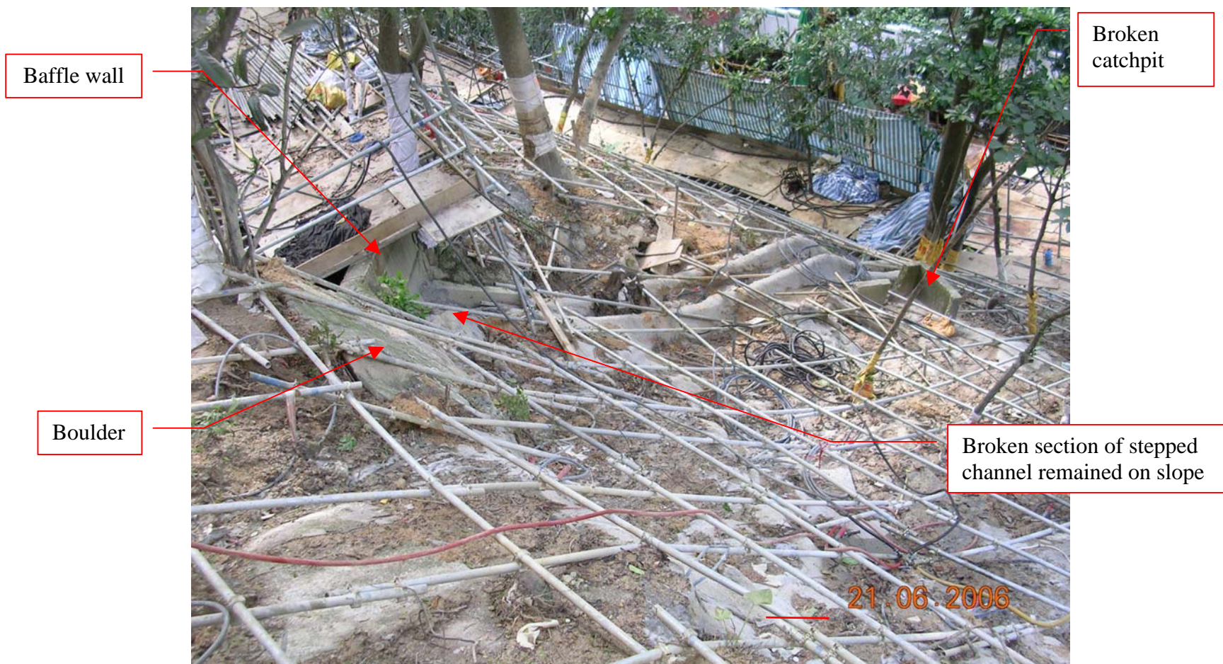
Plate 25 - Side View of the Slope below the Baffle Wall (Photograph taken by FSW on 21 June 2006)
