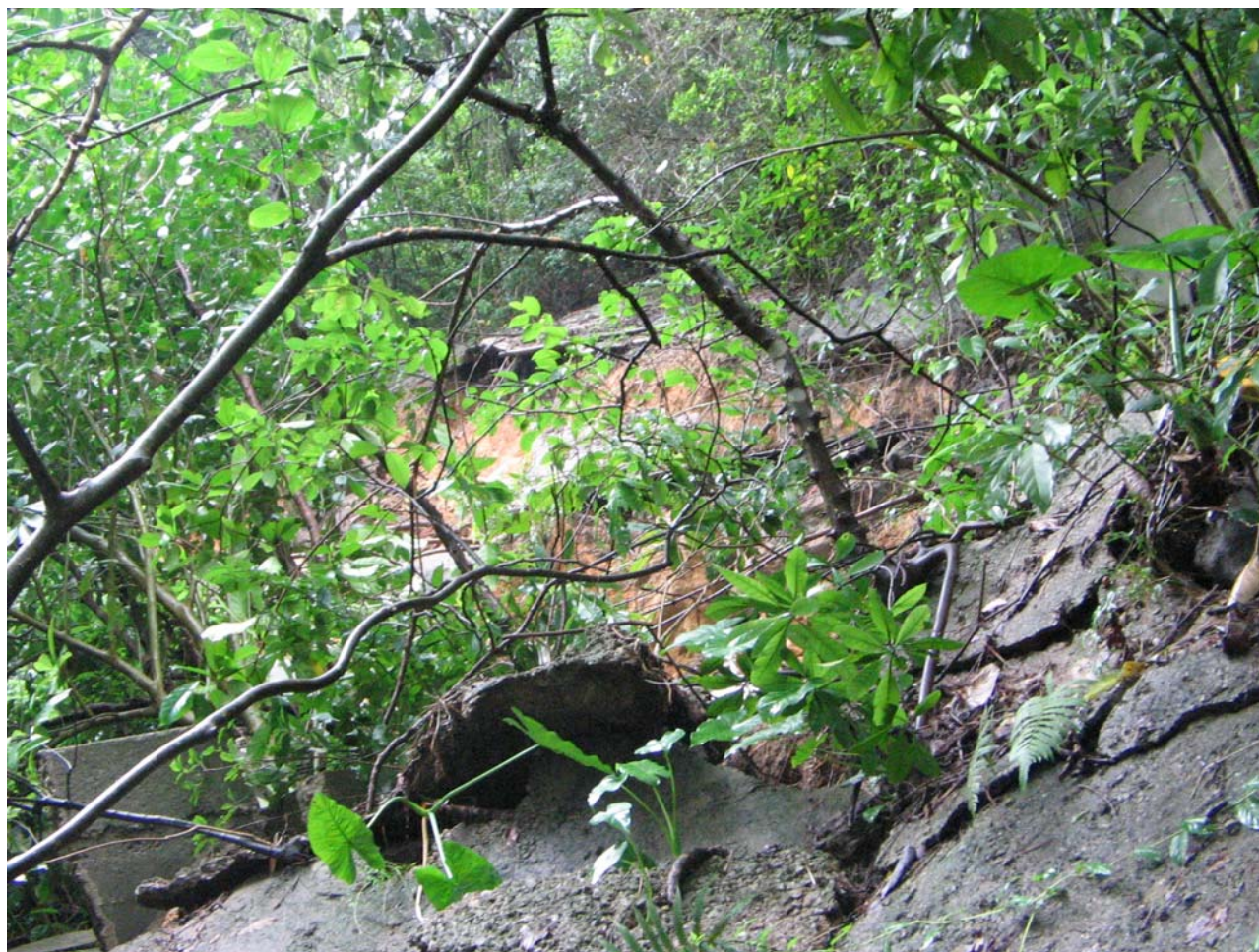
Plate 27 - View of a Cracked Chunam Cover at the Western Flank (Photograph taken by FSW on 24 August 2005)
