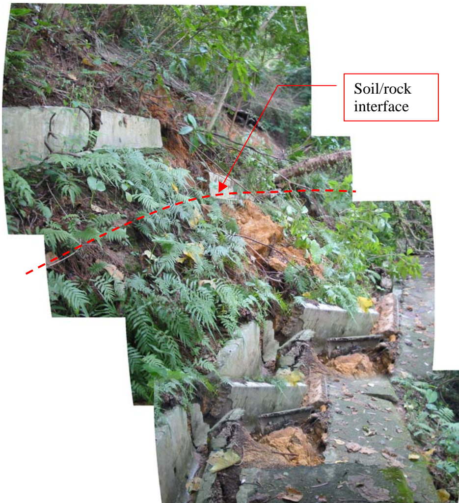
Plate 28 - View of the Soil/Rock Interface at the Lower Slope Batter (Photograph taken by FSW on 24 August 2005)
