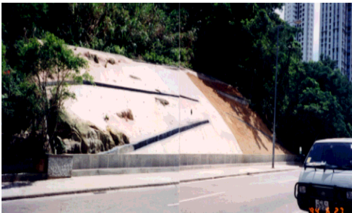
Plate 13 - View Showing the Completed Repair Works on Slope No. 11SE-A/C285 in June 1994 Following the Landslide in September 1993 (Photograph taken by GEO on 27 June 1994)
