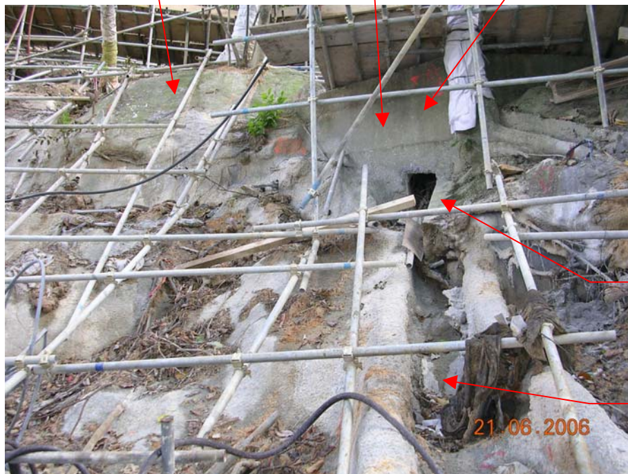
Plate 11 - View of the Baffle Wall above Slope No. 11SE-A/C285 (Photograph taken by FSW on 21 June 2006)
