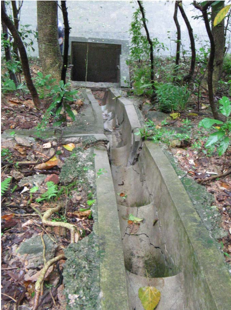
Plate 22 - Stepped Channel Showing Signs of Distress Resulting from the Landslide and from Scouring due to Excessive Flow of Water (Photograph taken by FSW on 24 August 2005)
