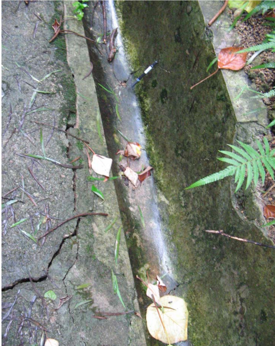
Plate 23 - View of a Surface Channel with Minor Cracks (Photograph taken by FSW on 24 August 2005)
