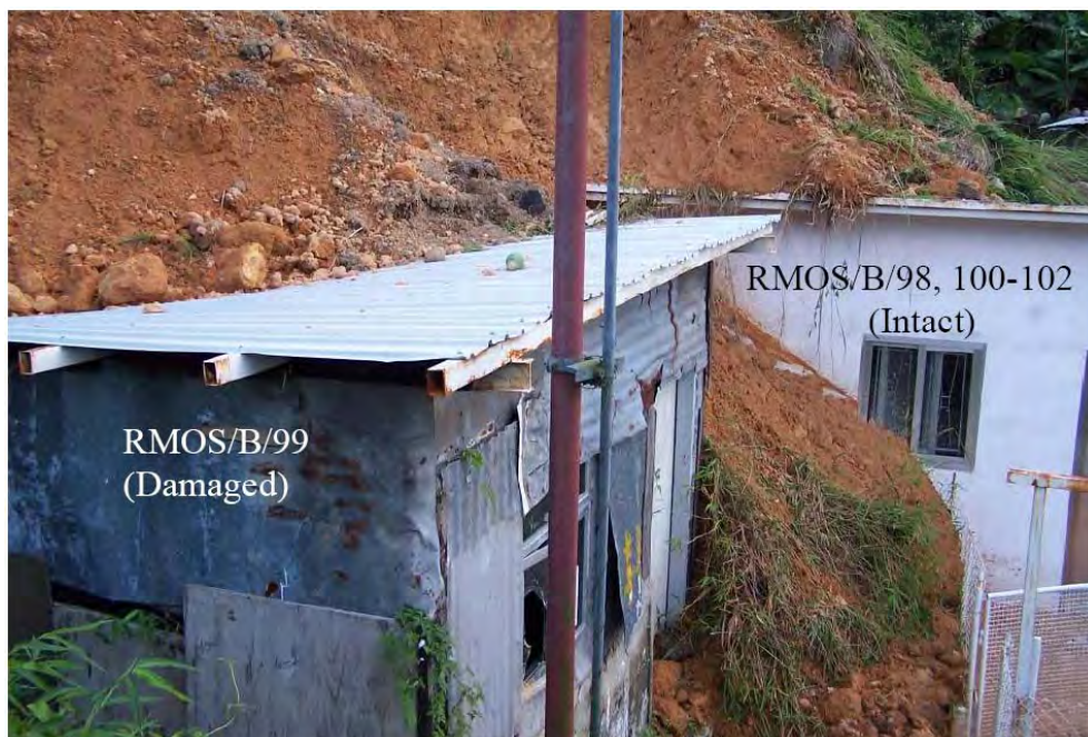
Plate 18 - Partly Buried and Damaged Registered Squatter Structures Nos. RMOS/B/98-102 at Northern Margin of the Debris Lobe (Photograph taken on 23 August 2005)
