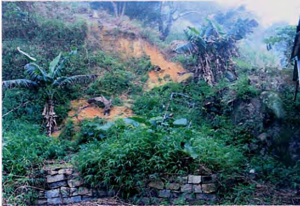
Plate 6 - View of the Landslide Observed by GEO in March 2003 on the Western Portion of Slope No. 7SE-B/C122 (Photograph taken on 4 March 2003 as extracted from GEO inspection record)
