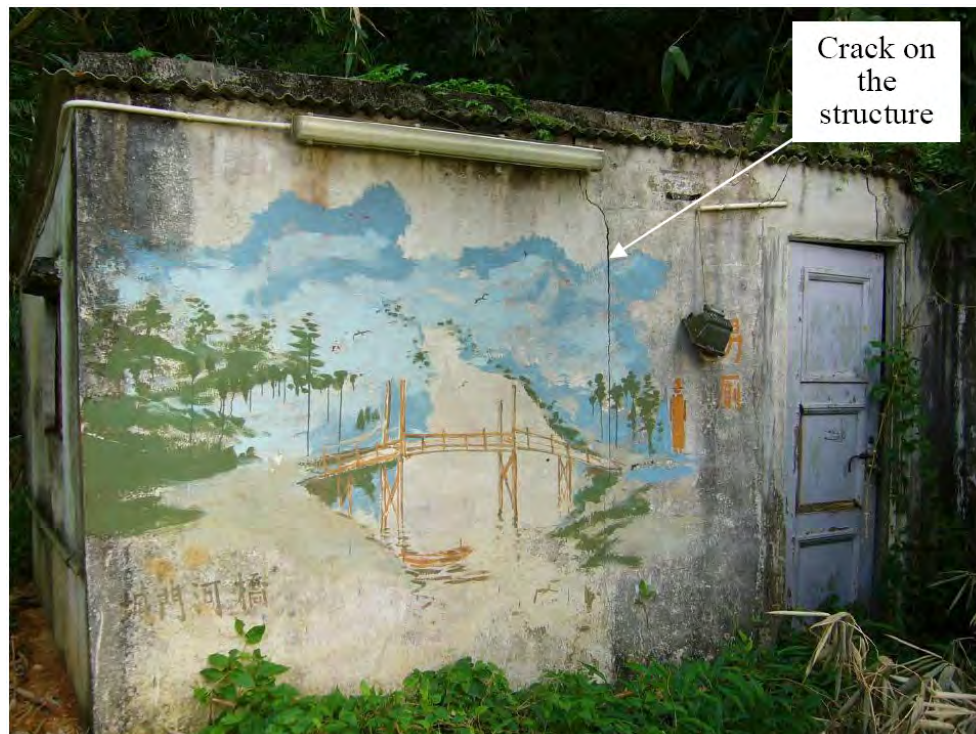
Plate 29 - Crack Observed on the Toilet/Shower Structure (Photograph taken on 14 October 2005)
