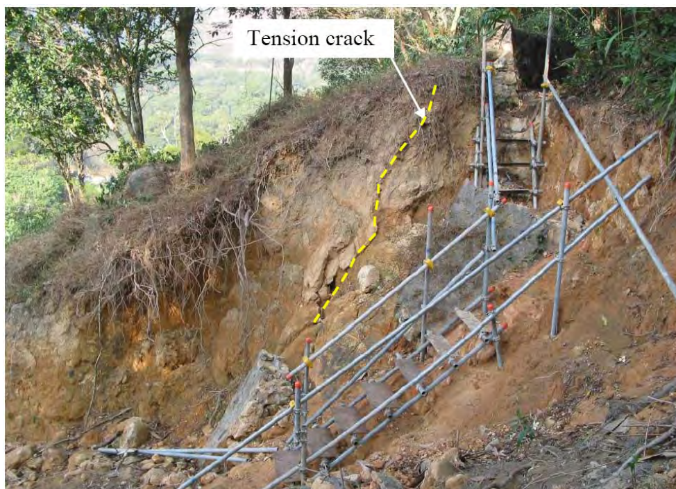
Plate 16 - Tension Crack Exposed on the Eastern Flank of the August 2005 Landslide (Photograph taken on 2 December 2005)
