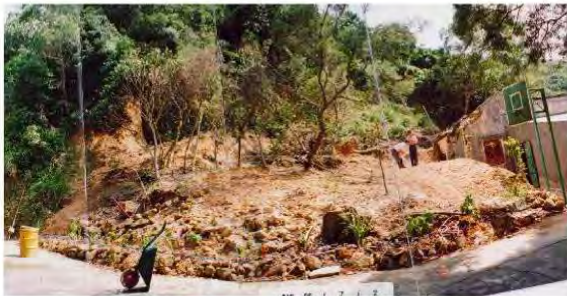
Plate 5 - View of Landslide Incident No. ME95/7/2 (Location A) at Slope No. 7SE-B/C122 with a Failure Volume of about 200 m 3 (Photograph taken on 10 July 1995 as extracted from Incident Report)
