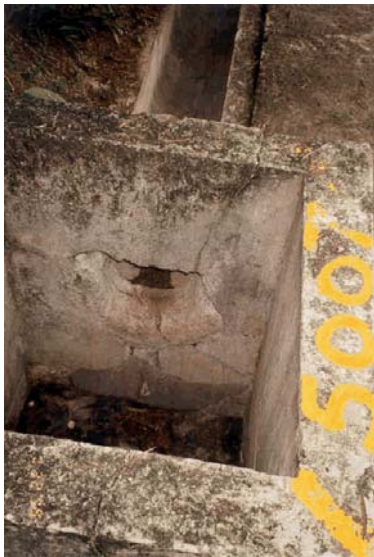
Cracked catchpit
