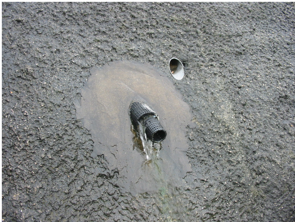
Plate 14 - Seepage from Raking Drain above the Lowest Batter of the Northern Part of Slope No. 11NE-A/C153 (Photograph taken on 24 August 2005)
