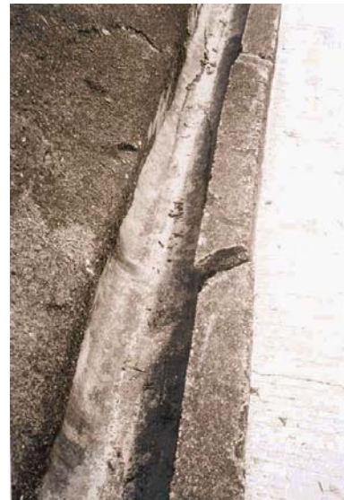
Cracked channel at slope toe
