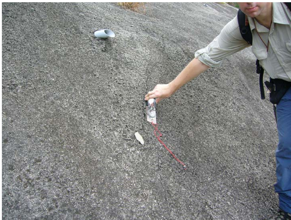
Plate 18 - Cracked Shotcrete Surface above the Displaced Rock Wedge (Photograph taken on 14 September 2005)
