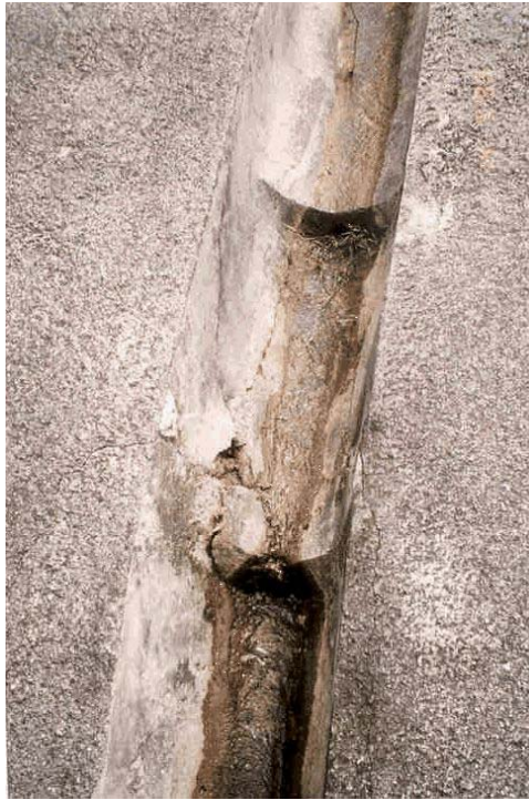
Cracked stepped channel and seepage
