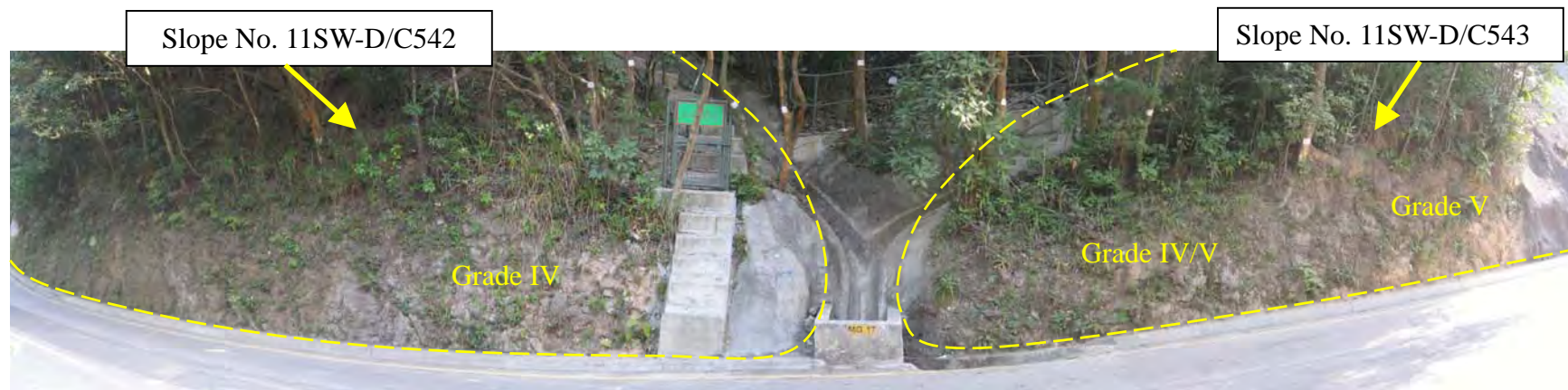
Plate 26 - View across Northern Extent of Slopes Nos. 11SW-D/C542 and 11SW-D/C543 Showing Weathering Gradient of Exposed Decomposed Volcanics
