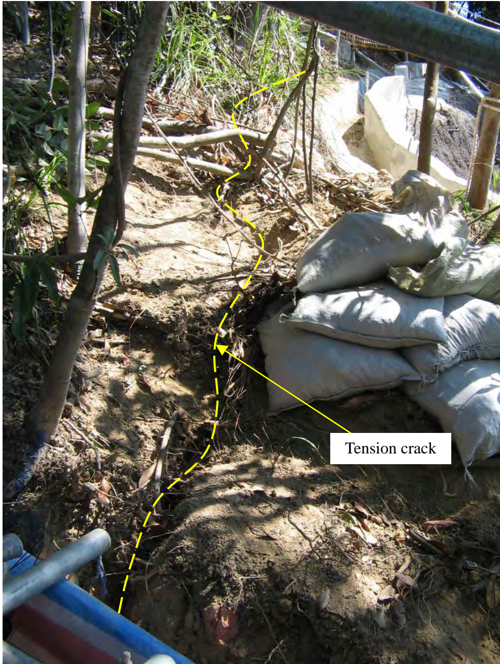
Plate 30 - Tension Crack Identified in Vegetation Strip VS3 behind Main Scarp (Photograph taken on 21 February 2006)
