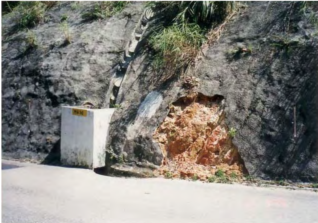
Plate 5 - Record Photograph of Slope No. 11SW-D/C543 Taken in August/September 1995 Showing Small Detachment from Central Portion of Slope (Photograph taken by Highways Department in August/September 1995)
