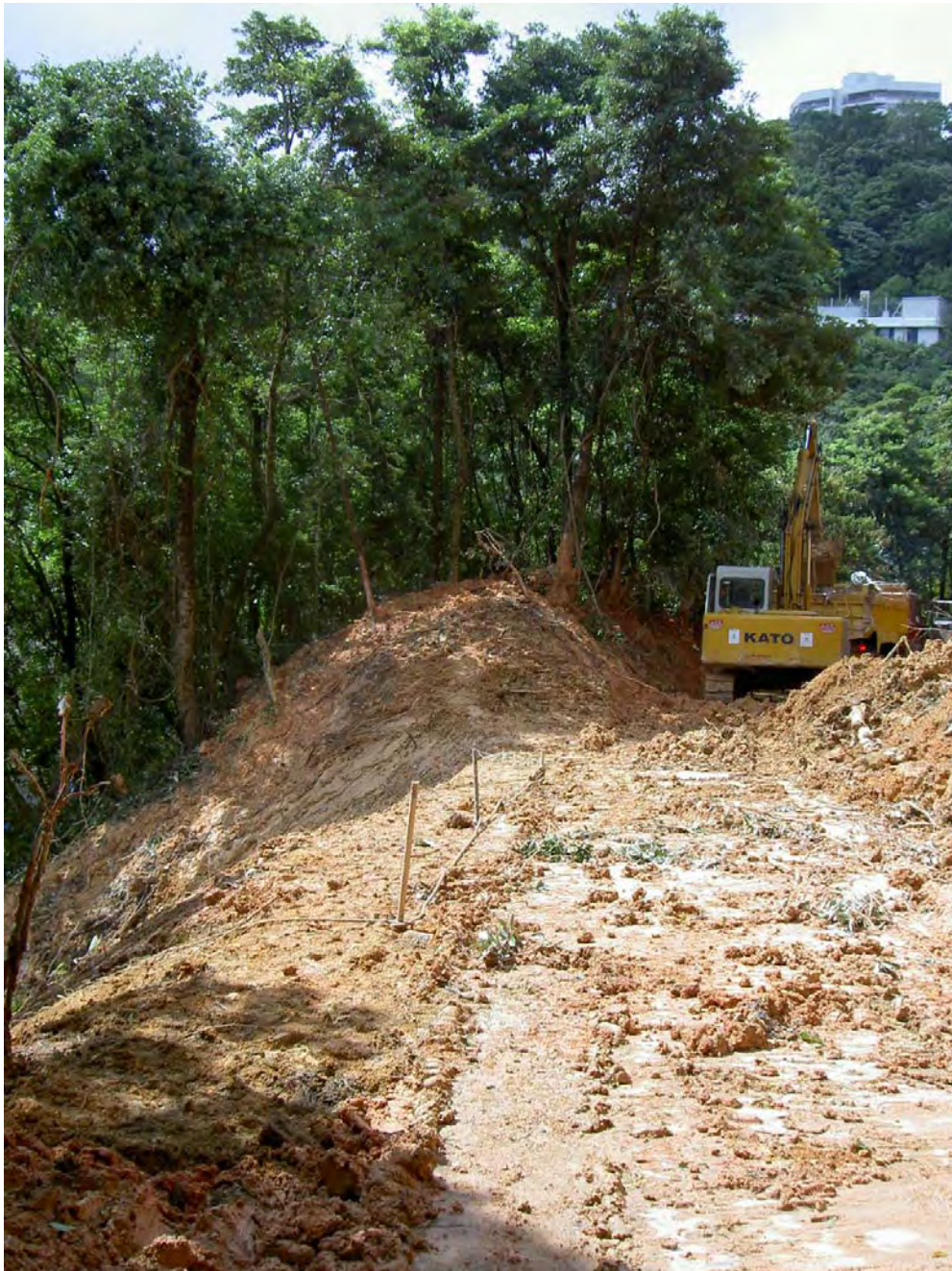
Plate 22 - View West across Middle Gap Road Showing Debris Mound Contained by Small Cutting
