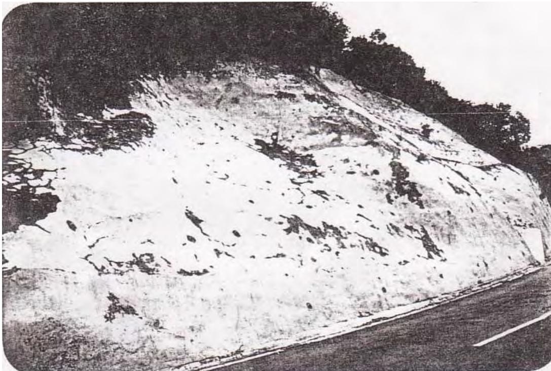
Plate 4 - Record Photograph of Slope No. 11SW-D/C543 Taken in April 1978 Showing Slope Geometry Modified by Previous Instability (Photograph extracted from Binnie & Partners (HK) Phase I Re-appraisal of Cut & Natural Slopes & Retaining Walls)
