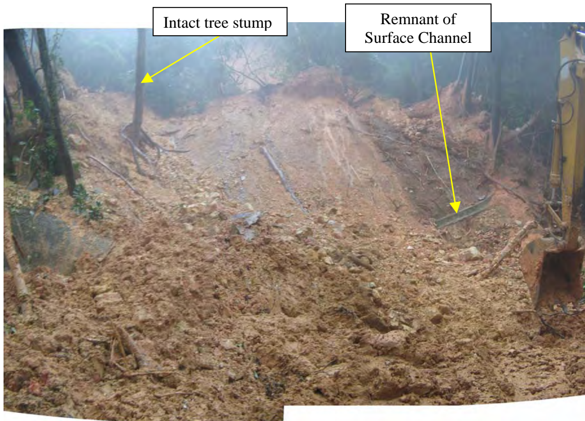
Plate 25 - View East from Mount Cameron Road Showing Sloping Ground in Debris Trail with Intact Tree Stumps and Remnants of Surface Channel
