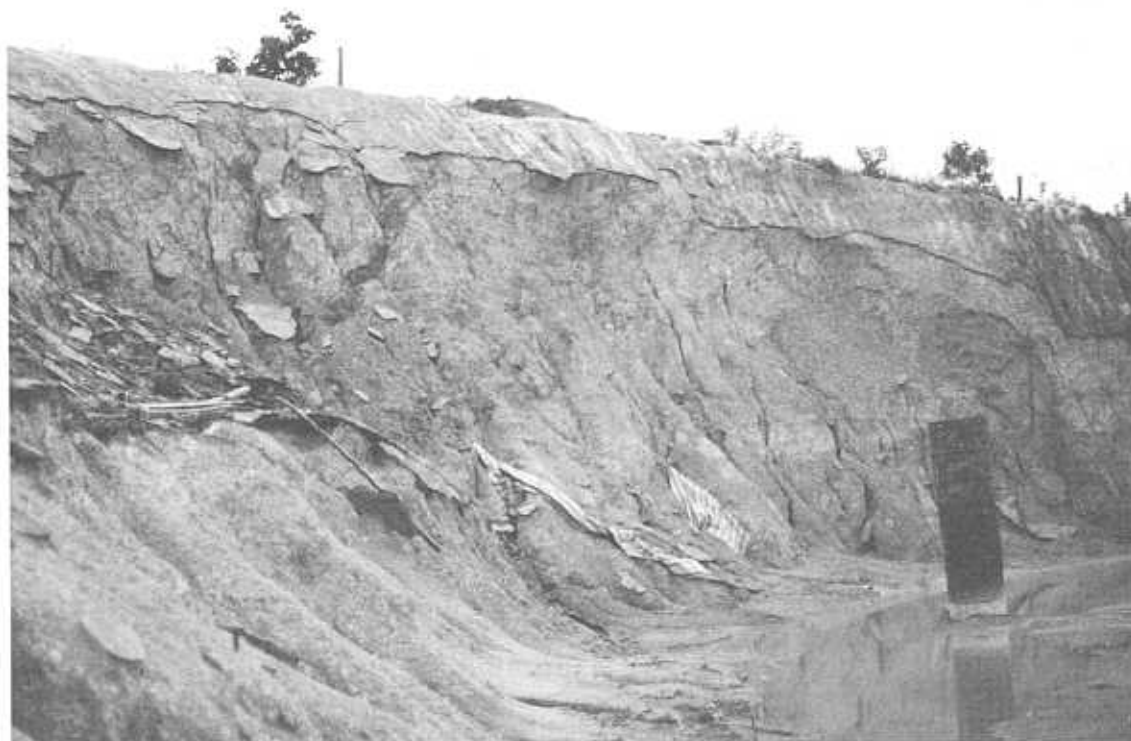
Plate 7 - Faults Exposed in a Temporary Cut Slope behind the Ma On Shan Water Reservoir (see Figure 10)
