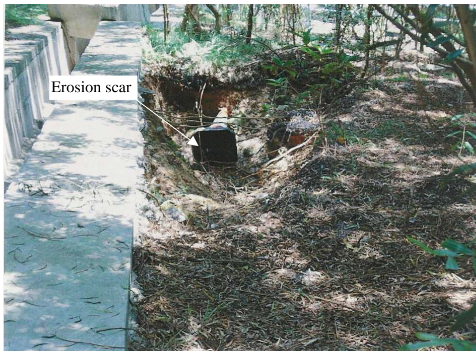
Plate 5 - Slope Distress and Erosion on a Fill Slope below Shek O Road near Lan Nai Wan, Shek O
