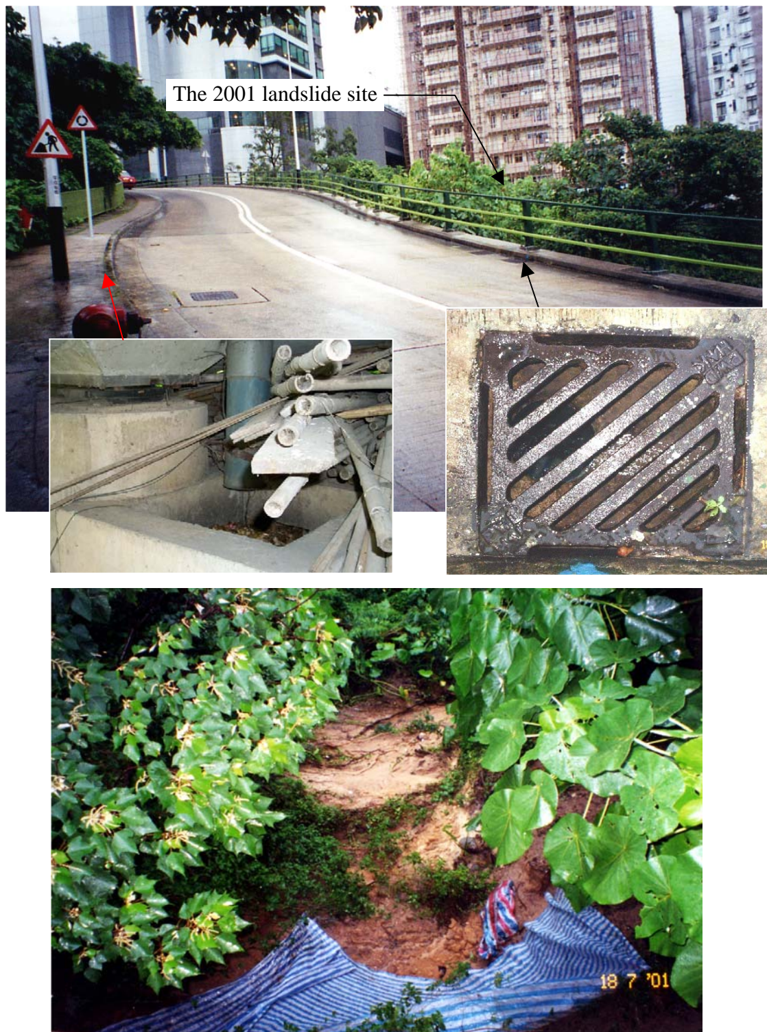
Plate 6 - The July 2001 Landslide on a Fill Slope below Broadwood Road, Happy Valley
