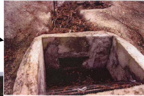
Blocked catchpit 50 m from landslide
