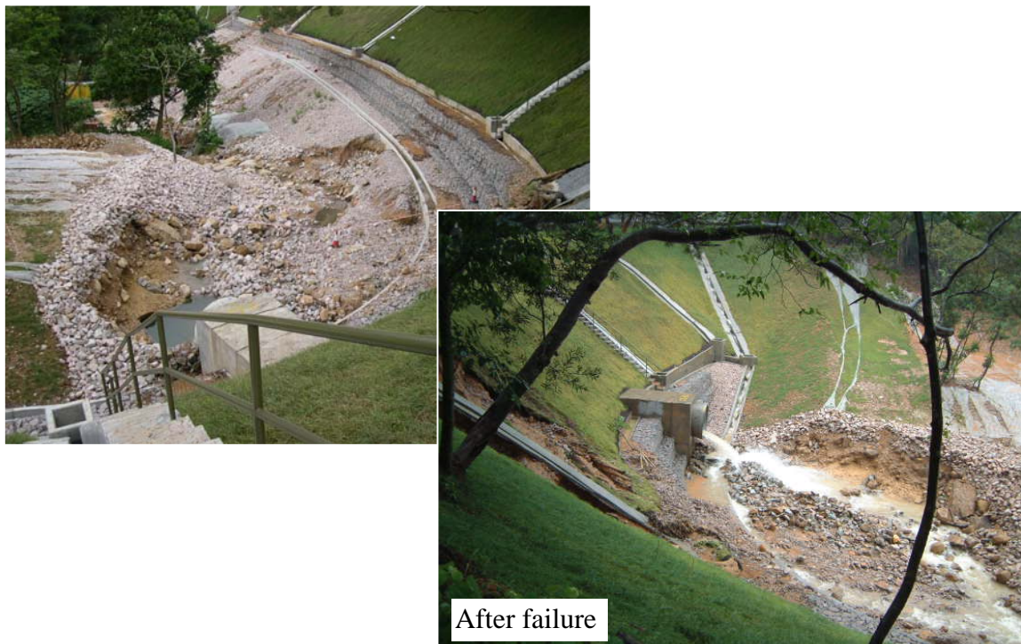
Plate 4 - The Energy Disperser for a 1350 mm Diameter Pipe Culvert and Erosion during the 5 May 2003 Washouts at South Lantau Road
