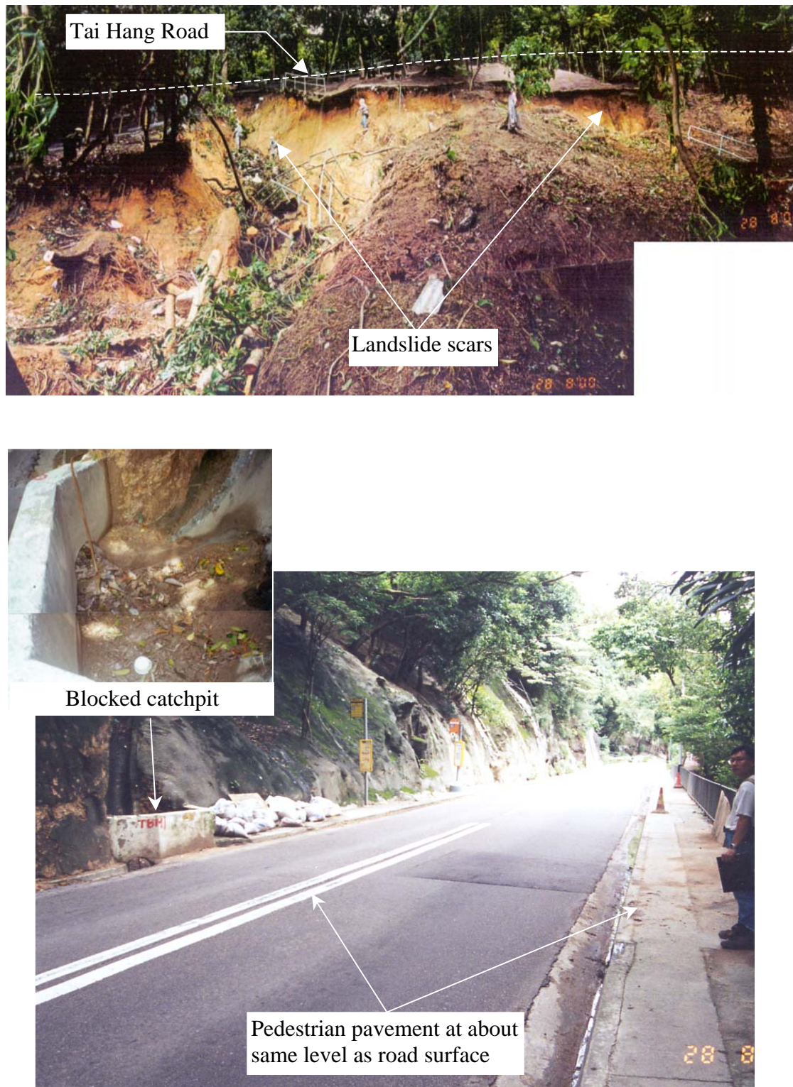
Plate 14 - The 24 August 2000 Landslide on a Disturbed Hillside below Tai Hang Road
