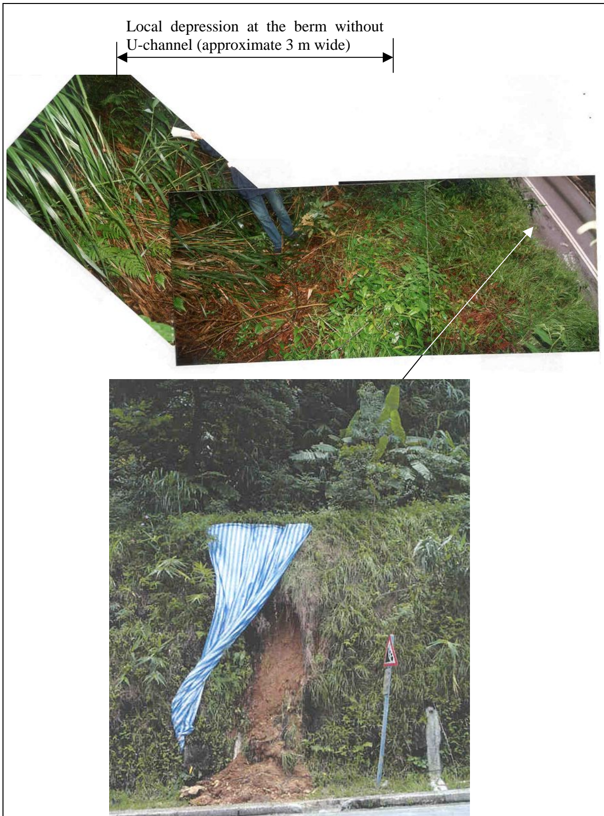
Plate 13 - The June 2001 Landslide on a Cut Slope at Route Twisk
