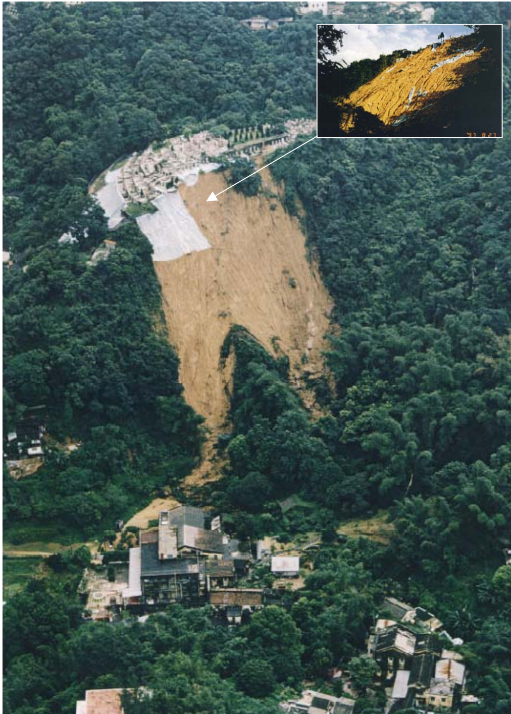
Plate 7 - The 2 July 1997 Landslide A on a Cut Slope at Tao Fung Shan Christian Cemetery, Sha Tin
