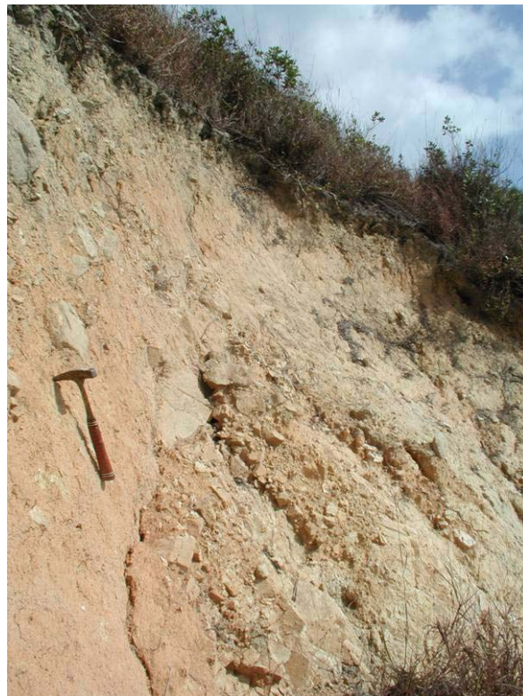
Plate 6 – View of Planar Main Scarp at Landslide 01B (Photograph Taken on 30 November 2001)
