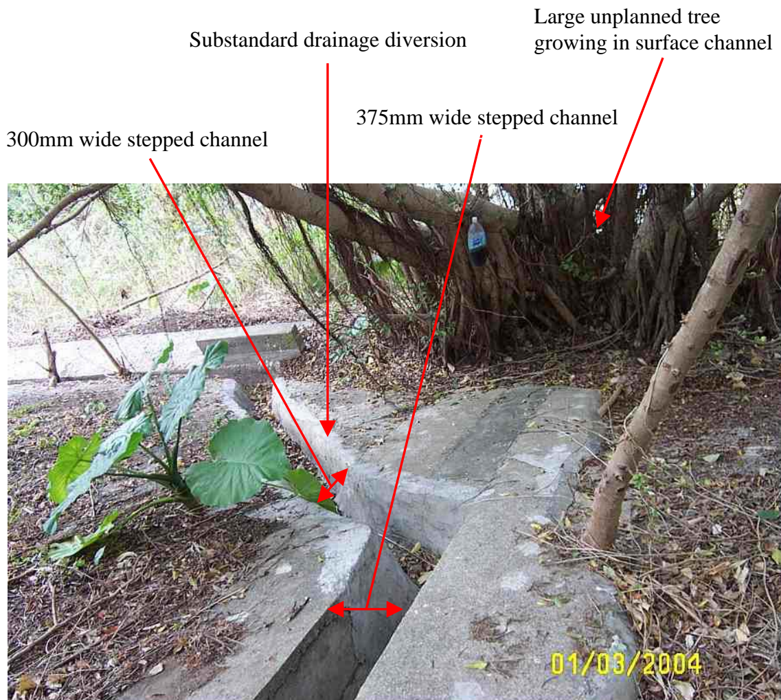
Plate 24 - Unplanned Vegetation Blocks Surface Drainage System (Photograph taken on 1 March 2004)
