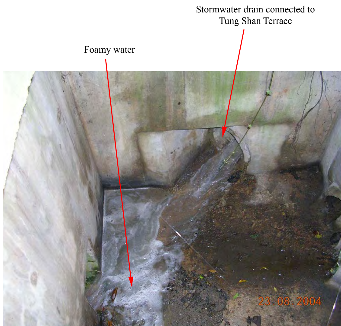
Plate 38 - Anomalous Flow of Foamy Water Observed at Stormwater Outlet Entering Surface Drainage System of Slope No. 11SW-D/FR1 at Slope Crest (Photograph taken on 23 August 2004)
