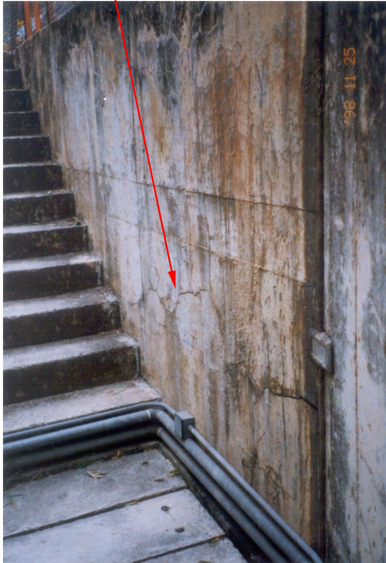
Plate 14 - Cracking in Mass Concrete Gravity Retaining Wall near Access Stairs (Photograph taken by Highways Department on 25 November 1998)
