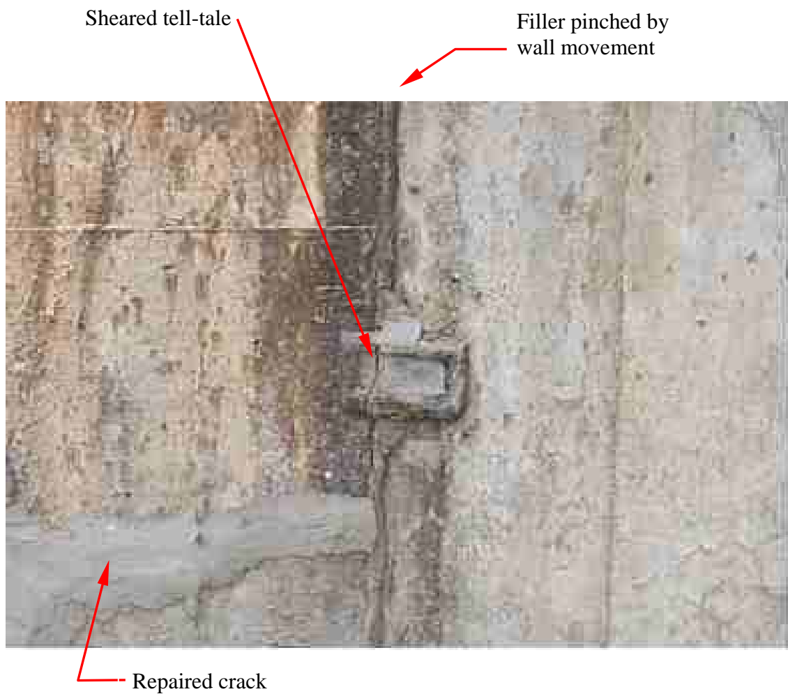
Plate 26 - Expansion Joint in Mass Concrete Gravity Retaining Wall (Photograph taken on 25 February 2004)
