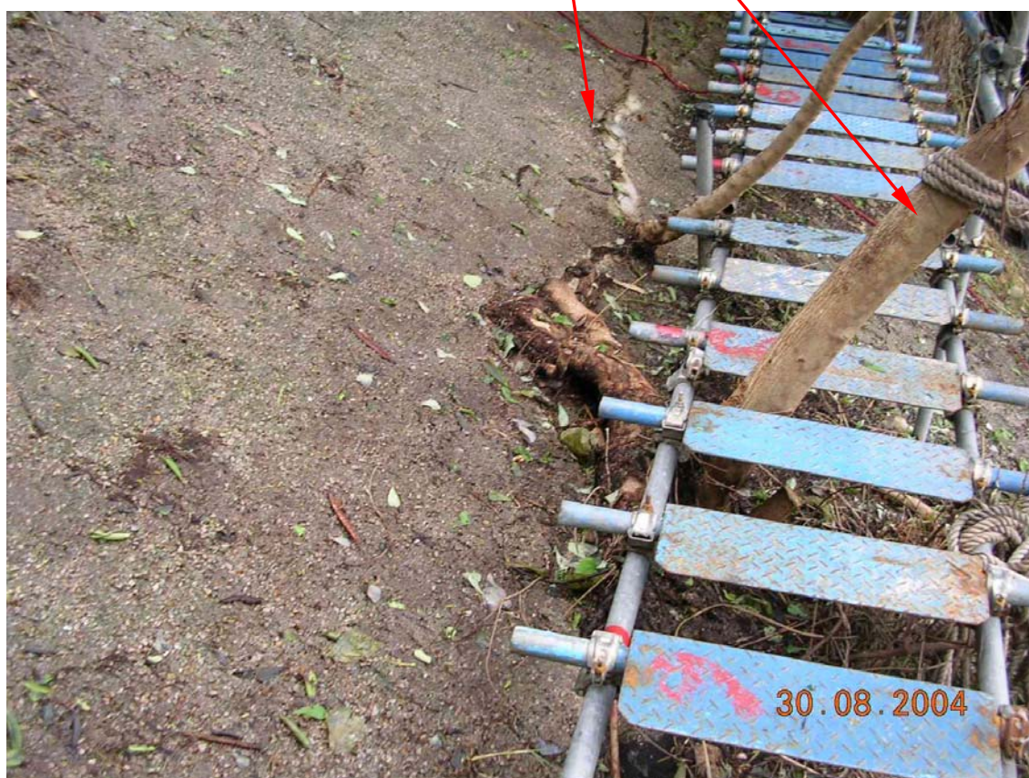
Plate 23 - Example of Unplanned Vegetation Exploiting Cracks in Shotcrete Surfacing on Third Batter above Slope Toe (Photograph taken on 30 August 2004)
