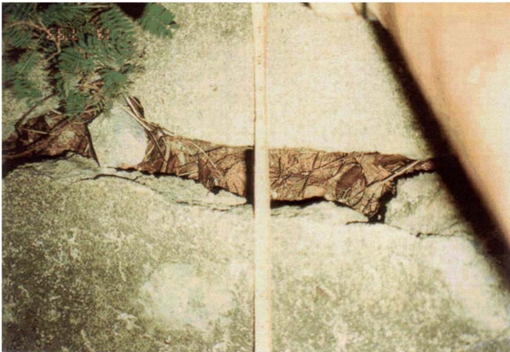
Plate 16 - Close View of Cracking between Stepped Channel Apron and Shotcrete on 4 th Batter above Slope Toe (Photograph taken by Maunsell Geotechnical Services in July 1999)
