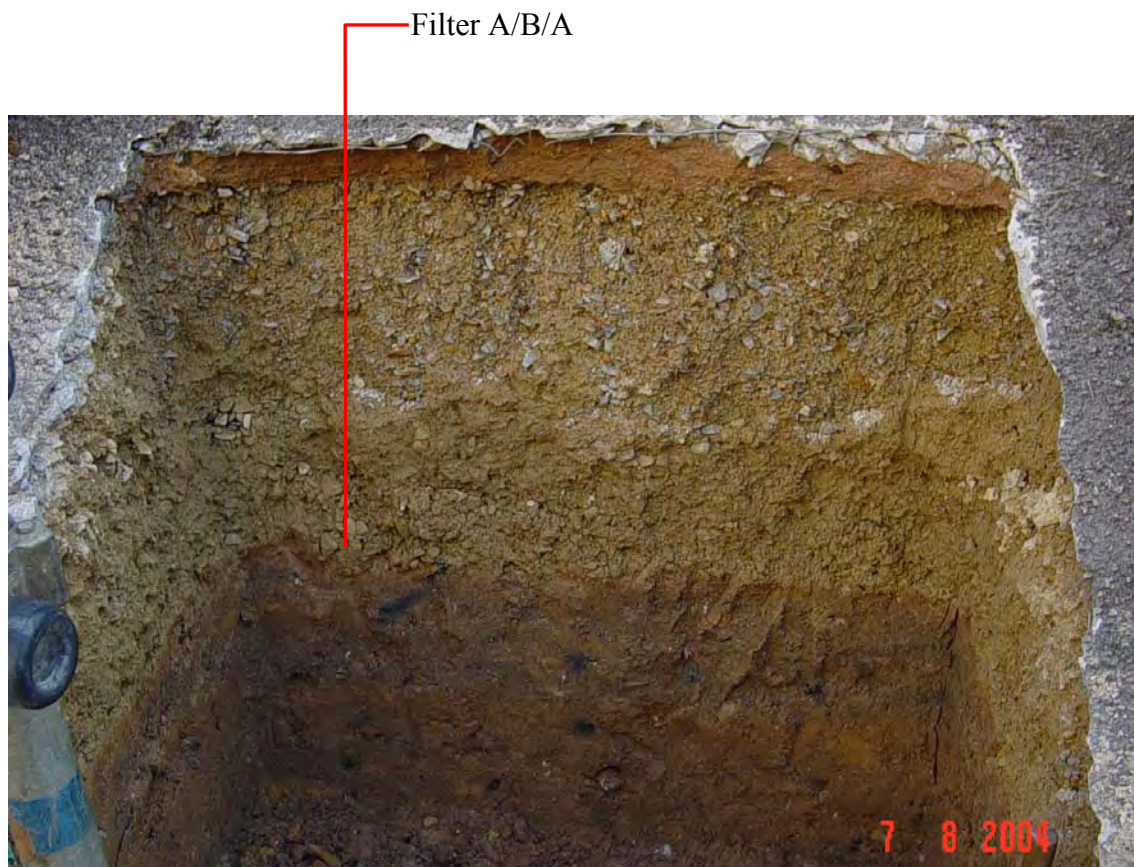
Plate 34 - Close View of Filter A/B/A Arrangement Exposed in Trial Pit TP5 Showing Lack of Definition between Individual Filter Layers (Photograph taken on 7 August 2004)
