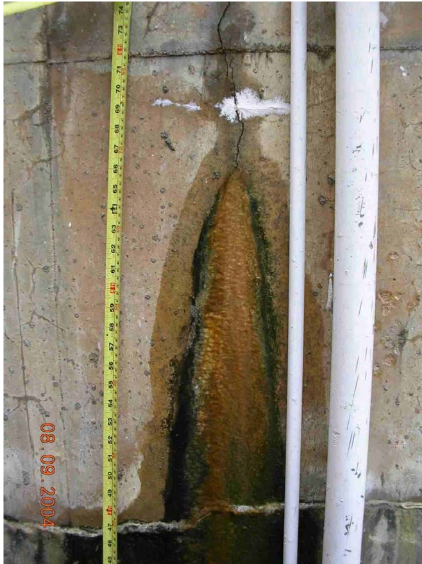
Plate 25 - Sustained Seepage Observed Issuing from Crack in Mass Concrete Gravity Retaining Wall (Photograph taken on 8 September 2004)
