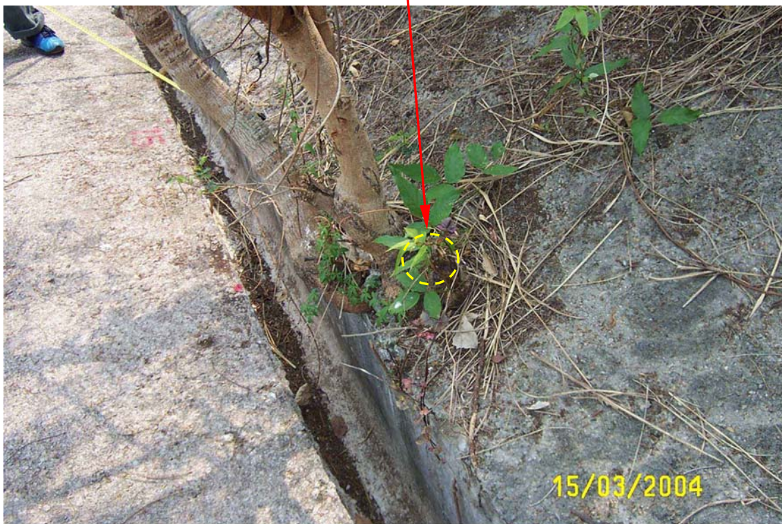
Plate 22 - Example of Blocked 75 mm Diameter Drainage Pipe Exploited by Unplanned Vegetation (Photograph taken on 15 March 2004)
