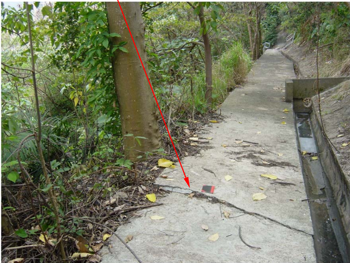
Plate 17 - Typical Example of Transverse Crack in Berm Slab (Photograph taken on 28 February 2004)
