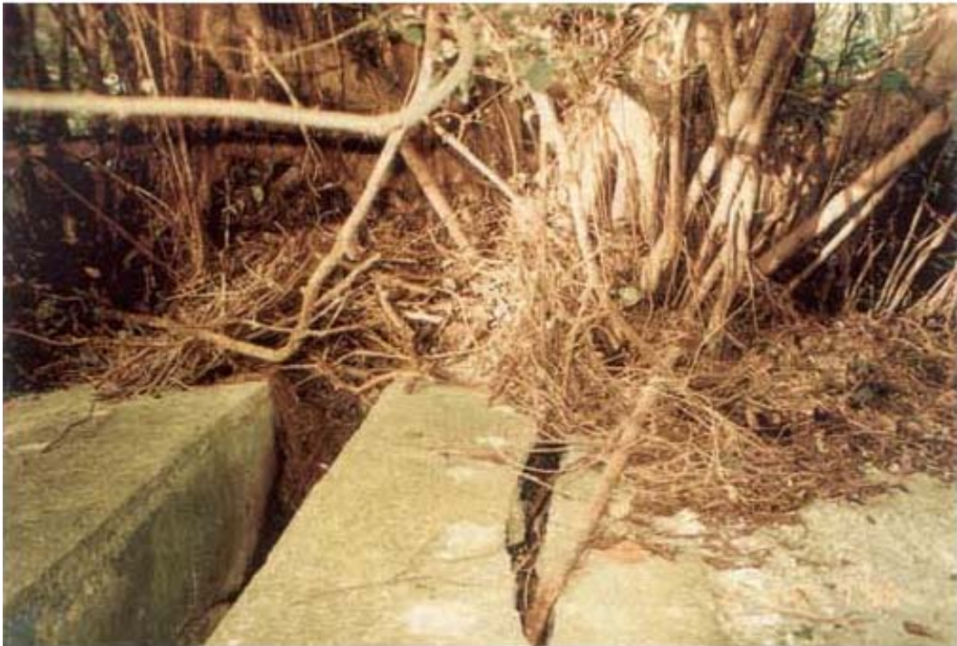
Plate 15 - View Down Stepped Channel on 4 th Batter above Slope Toe Showing Severe Cracking between Channel Apron and Adjacent Shotcrete and Growth of Unplanned Vegetation (Photograph taken by Maunsell Geotechnical Services in July 1999)
