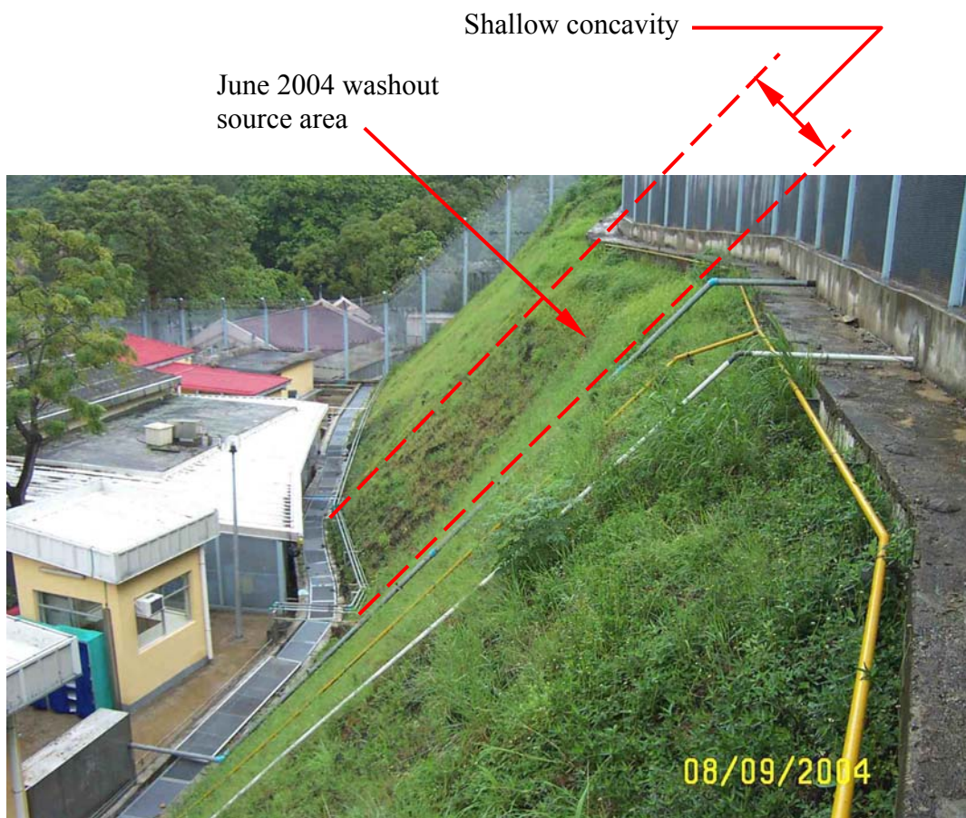
Plate 6 - View North along Crest Towards Location of the June 2004 Washout at Slope No. 10SW-D/C97 (Photograph taken on 8 September 2004)
