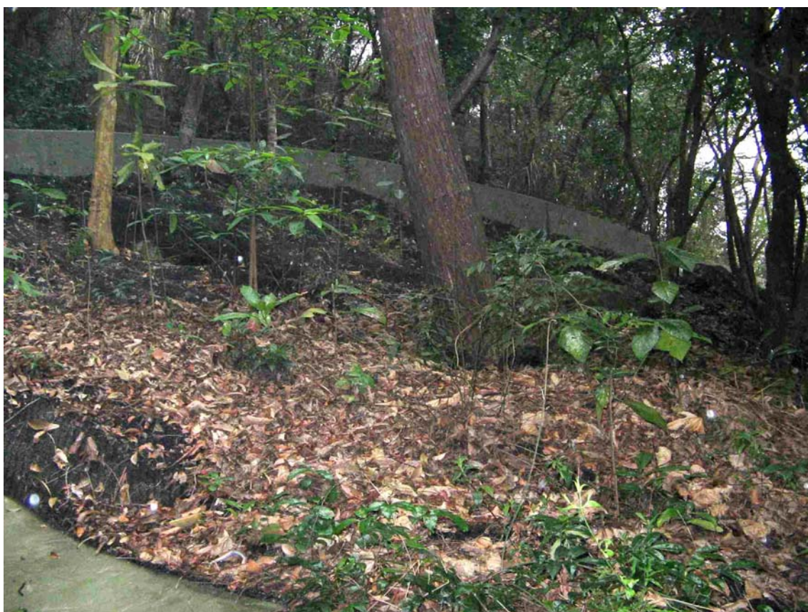
Plate 29 - Northeastern Portion of Slope No. 10SW-D/C101 where Establishment of Ground Cover Vegetation Limited by Tree Canopy and Leaf Litter (Photograph taken on 11 March 2005)
