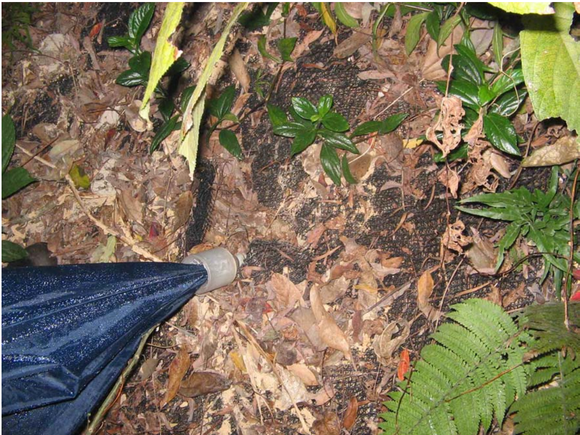
Plate 26 - Example of Erosion Control Mat having been Cut on Slope No. 10SW-D/C101 (Photograph taken on 11 March 2005)
