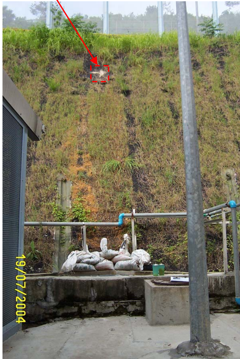
Plate 4 - General View of the Washout Scar on Slope No. 10SW-D/C97 (Photograph taken on 19 July 2004)
