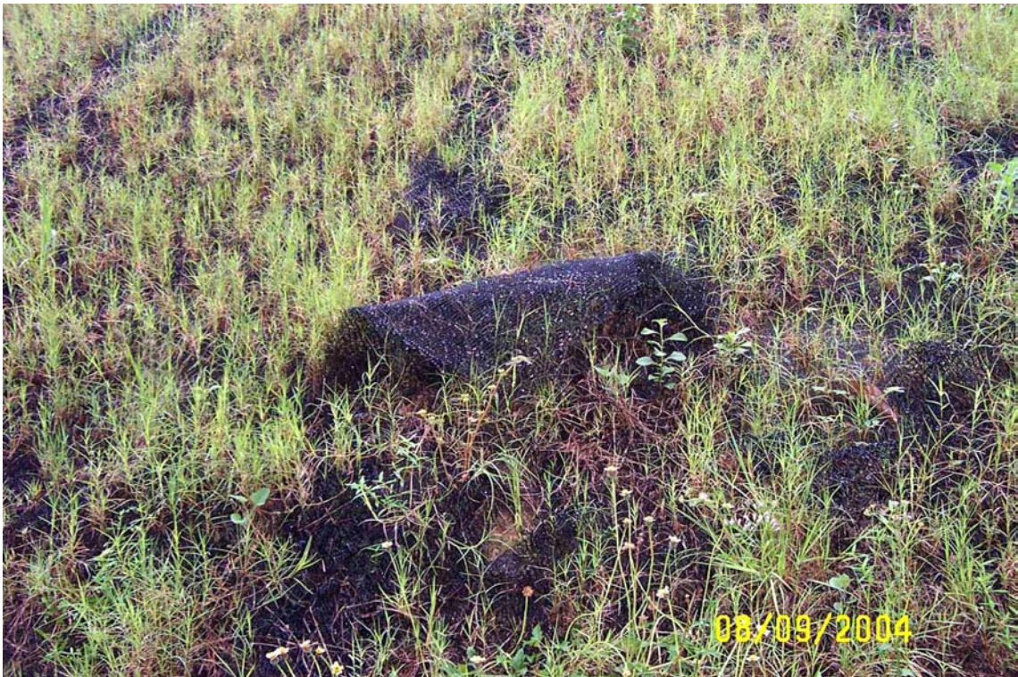
Plate 9 - Example of Erosion Control Mat having been Cut and Loose Flap Hanging Down Slope Face of Slope No. 10SW-D/C97 (Photograph taken on 8 September 2004)
