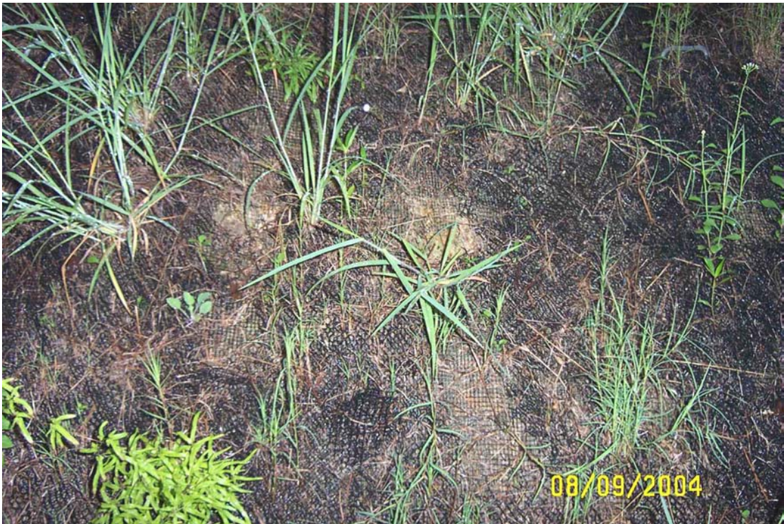
Plate 11 - Example of Location where Backing Mesh has been Torn to Expose Slope Face of Slope No. 10SW-D/C97 (Photograph taken on 8 September 2004)
