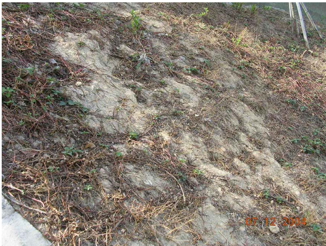
Plate 33 - Close View of Area of Exposed Ground on Face of Slope No. 10SW-D/F55 following Recent Vegetation Trimming (Photograph taken on 7 December 2004)
