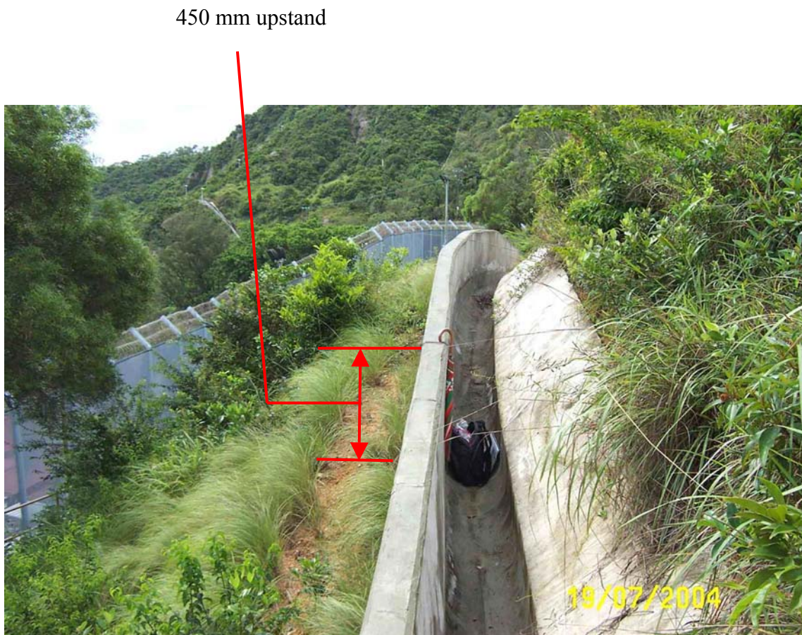
Plate 3 - General View of the 375 mm U-Channel Located Upslope of the Crest Berm of Slope No. 10SW-D/C97 Showing 450 mm Upstand on Channel Wall (Photograph taken on 19 July 2004)
