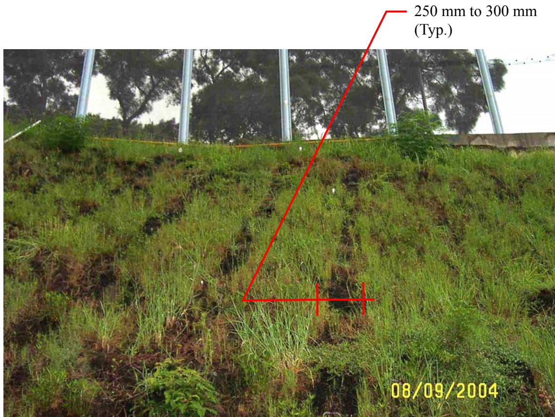
Plate 8 - General View of Central Portion of Slope Face from Toe Showing Typical Lap of Adjacent Sheets of Erosion Control Mats at Slope No. 10SW-D/C97 (Photograph taken on 8 September 2004)
