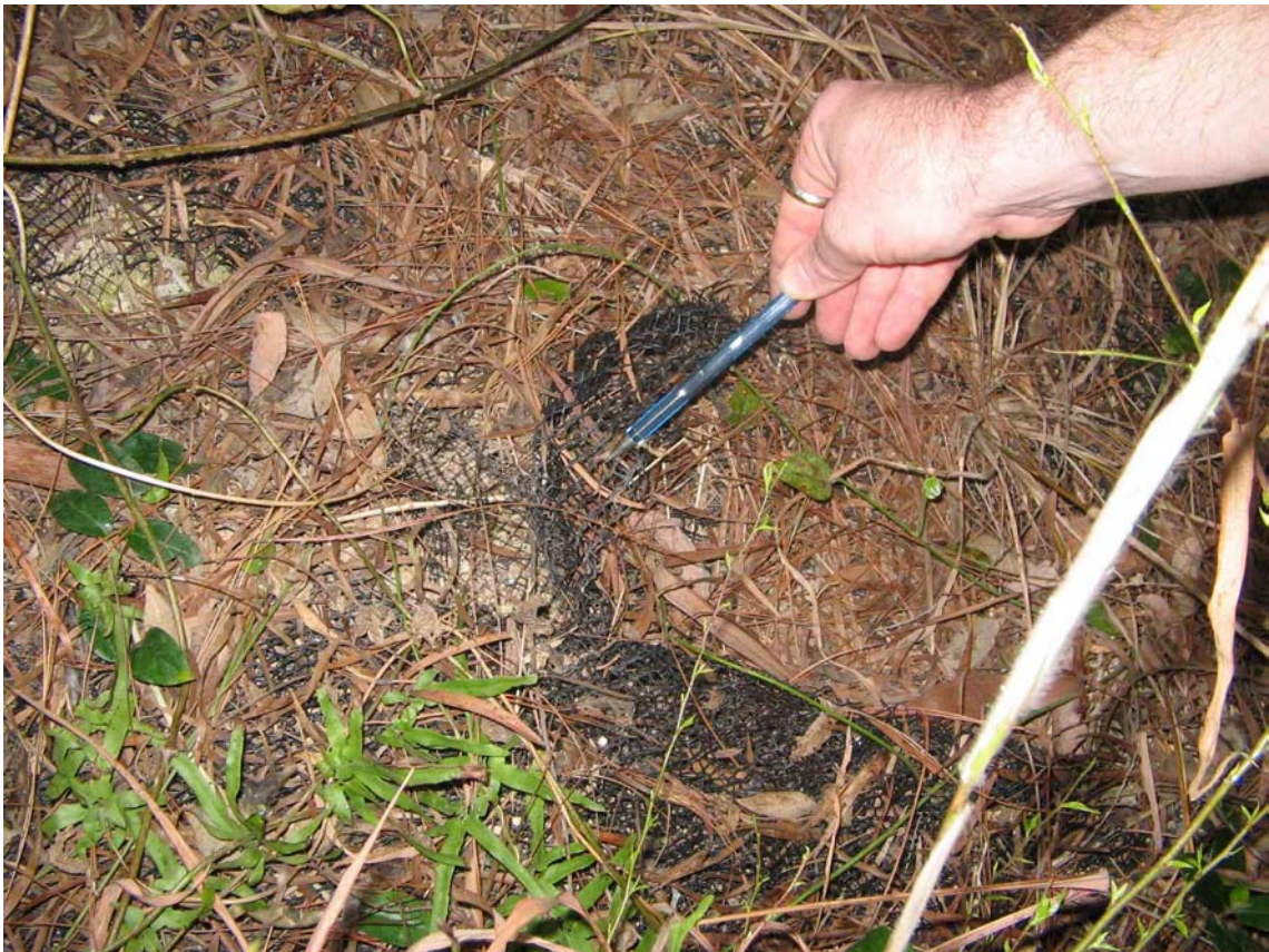
Plate 27 - Example of Erosion Control Mat having been Cut on Face of Slope No. 10SW-D/C102 (Photograph taken on 11 March 2005)
