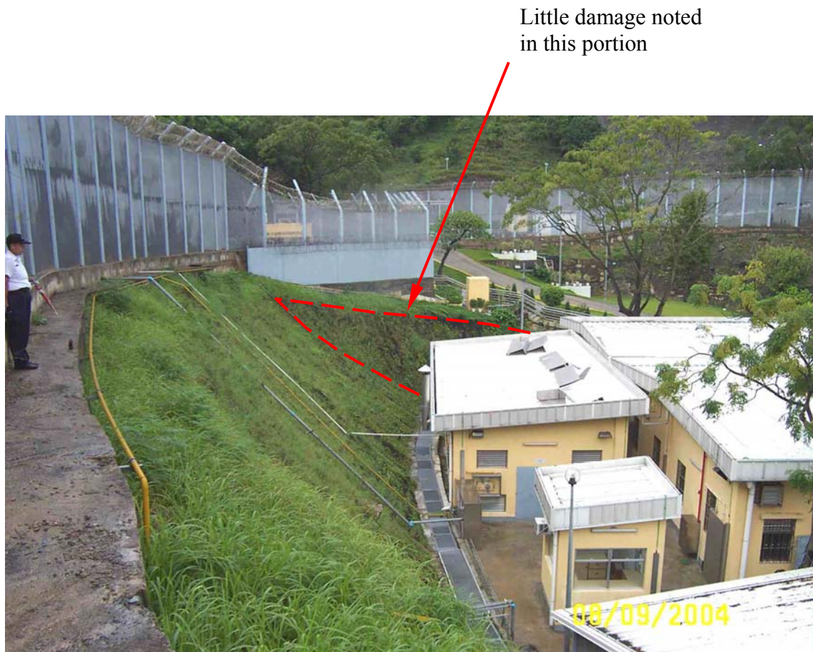
Plate 14 - View South Along Slope Crest Indicating Steeper Southern Portion of Slope No. 10SW-D/C97 where Little Damage to Erosion Control Mats (Photograph taken on 8 September 2004)
