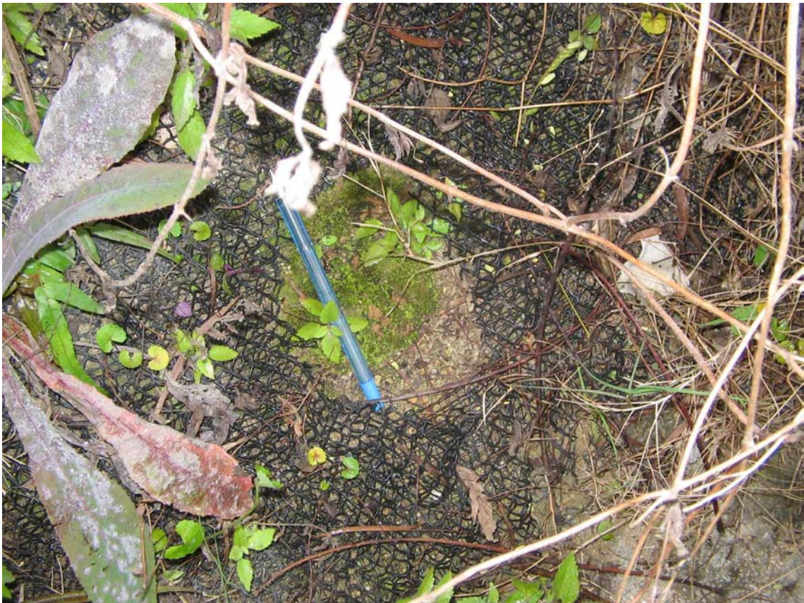
Plate 25 - Isolated Location on Lower Batter of Slope No. 10SW-D/C28 where Erosion Control Mat has been Cut (Photograph taken on 11 March 2005)
