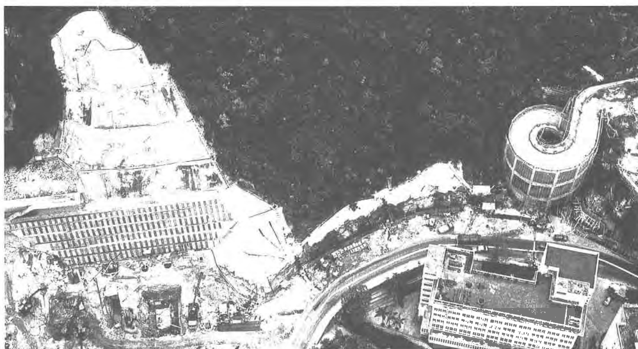
Plate 214. Oblique Aerial Photograph of Construction Associated with Private Development and the Realignment of Kennedy Road in 1979. Major slope works were carried out as part of the realignment of Kennedy Road and associated residential development. A spiral ramp has been used to provide access to a nearby apartment block. (GCO/OAP/1979/PS28-31).
