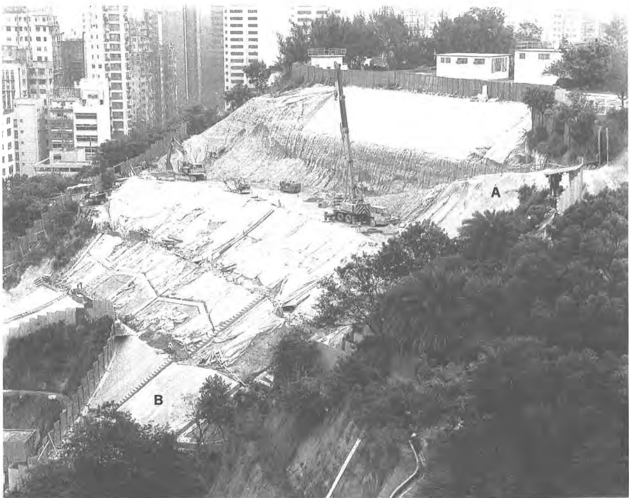
Plate 188. Slope Reconstruction at King's Park in April 1987. This photograph, taken on 27.4.87, provides a general view of the site. Temporary chunam is evident (A) above 60mPD, and permanent chunam is in place (B) below the first berm. Reconstruction of this fill slope cost in the order of $1.6m over a 17-month period. (Contract No. GC/84/03; Slope 11NW-D/F97).
