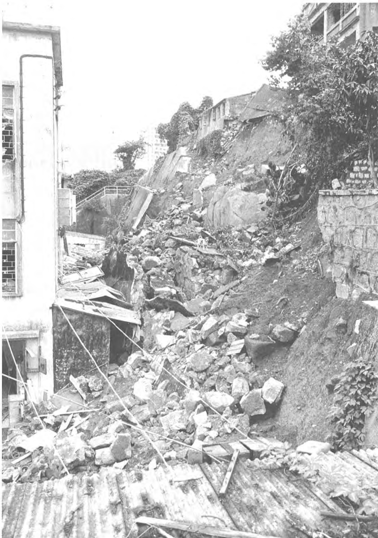
Plate 150. Landslip at Wa On Terrace in 1982. Failure of a cut slope and retaining wall caused damage to this residential property in the Tsuen Wan district. (GCO/1982/19/70/82).
