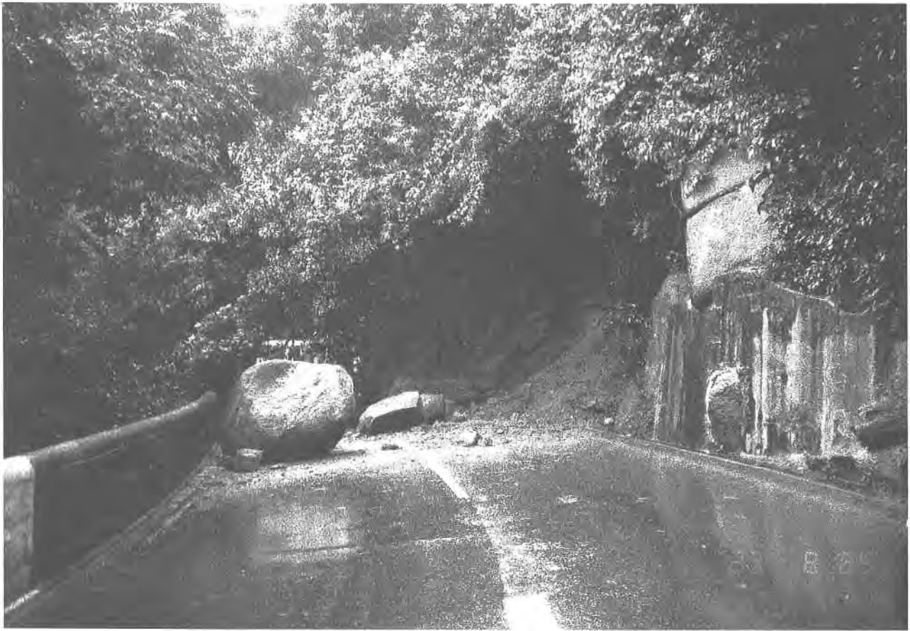
Plate 161. Landslip on Stubbs Road in 1985. A landslip and rockfall near 34 Stubbs Road resulted in disruption of road traffic. (GCO/IW/1985/IW85/267/0).
