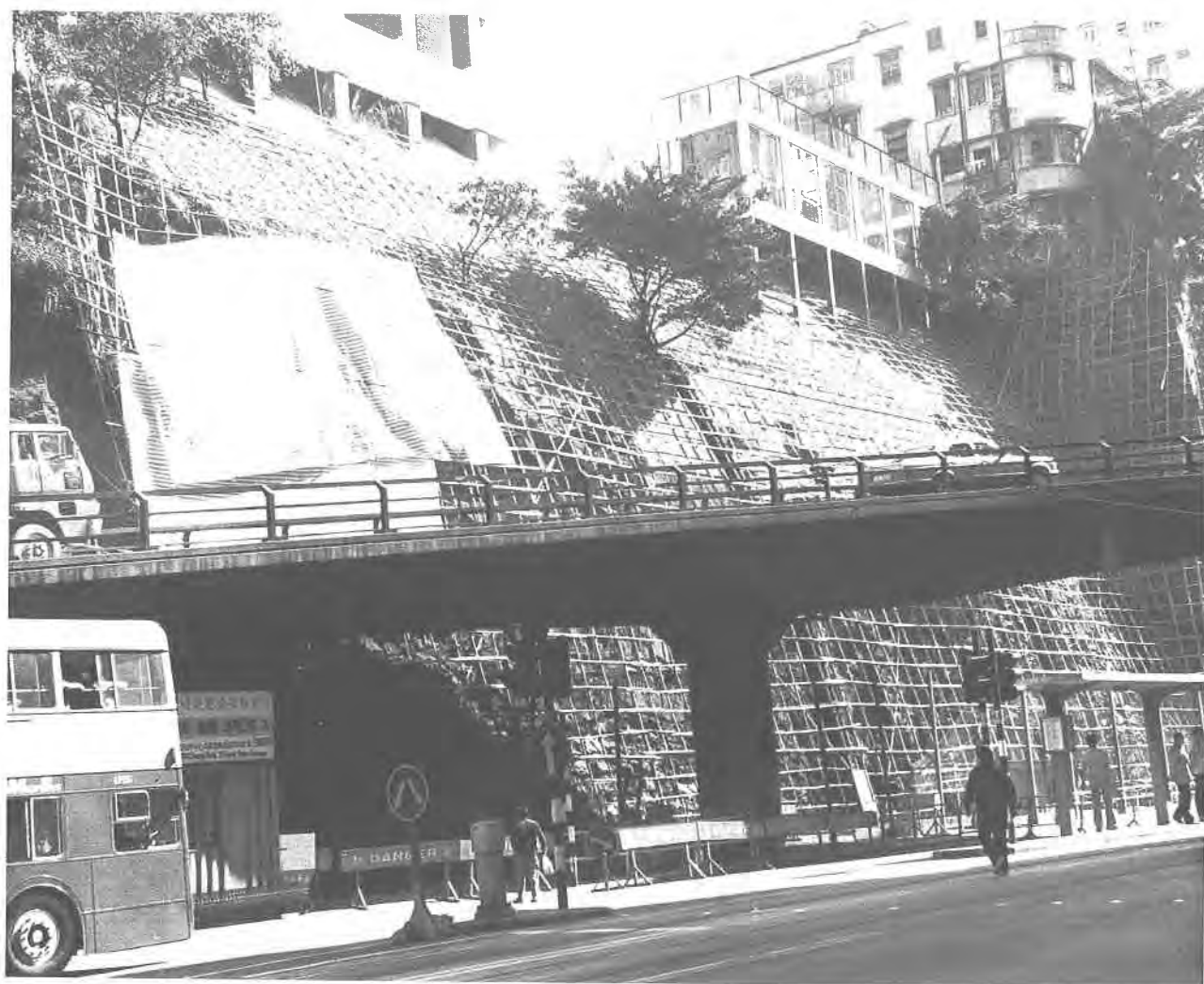
Plate 176. Stabilization of a Rock Slope on King's Road in December 1983. This large, almost vertical rock slope was treated by the Geotechnical Control Office within the Landslip Preventive Measures Programme, at a cost of some $710,000 over a period of 12 months. This photograph was taken on 6.12.83. (3/GCO/82 & 5/GCO/83, 11SE-A/C13 & 14).
