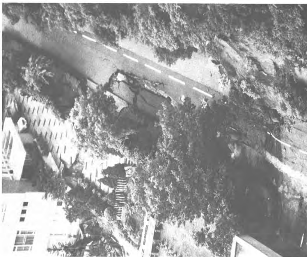
Plate 100. Distress Evident on the Lawn and Garage Area of 21 Po Shan Road prior to the Landslip in 1972.
