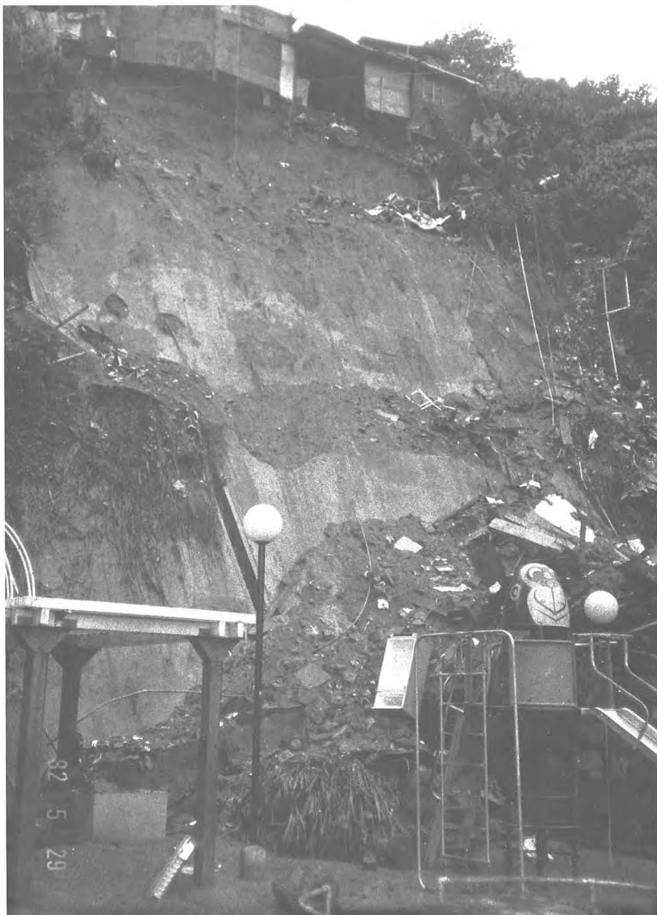
Plate 139. Landslip at Tsin Shui Ma Tau in 1982. The landslide is viewed from the playground at the base of the slope, and the precarious position of the undermined squatter huts is evident. An aerial view of the landslide is presented in Plate 140. (GCO/ES/1982/206819).
