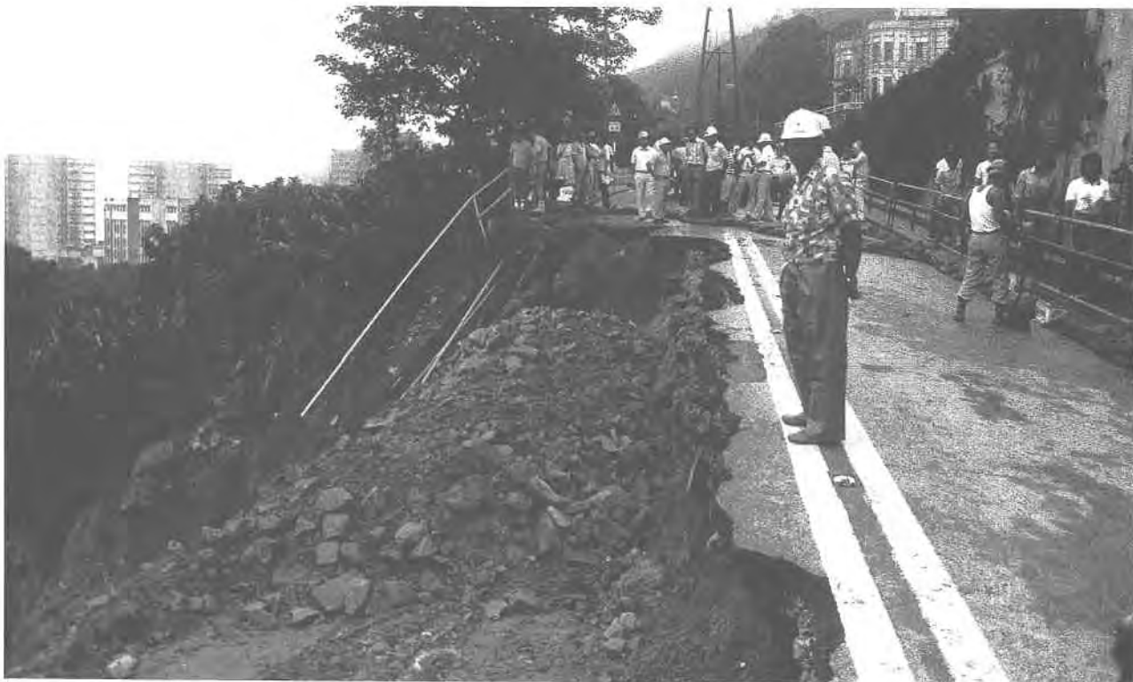
Plate 153. Landslip on Peak Road in 1983. This landslide severely damaged the westbound carriageway of Peak Road near the junction with Magazine Gap Road and resulted in the closure of the only access to The Peak for a week. An aerial view of site is given in Plate 57, and remedial works are shown at B in Plate 190. (GCO/1983/83/122/12A).
