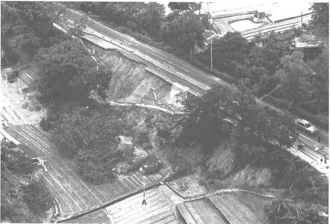
Plate 152. Landslip on Road Embankment near Sui Wo Village in 1982. This landslide occurred near the 17.5 milestone on Castle Peak Road and damaged agricultural land. A vehicle, presumably parked on the carriageway at the time of failure, is evident at A. (GCO/OAP/1982/PS275-9A).
