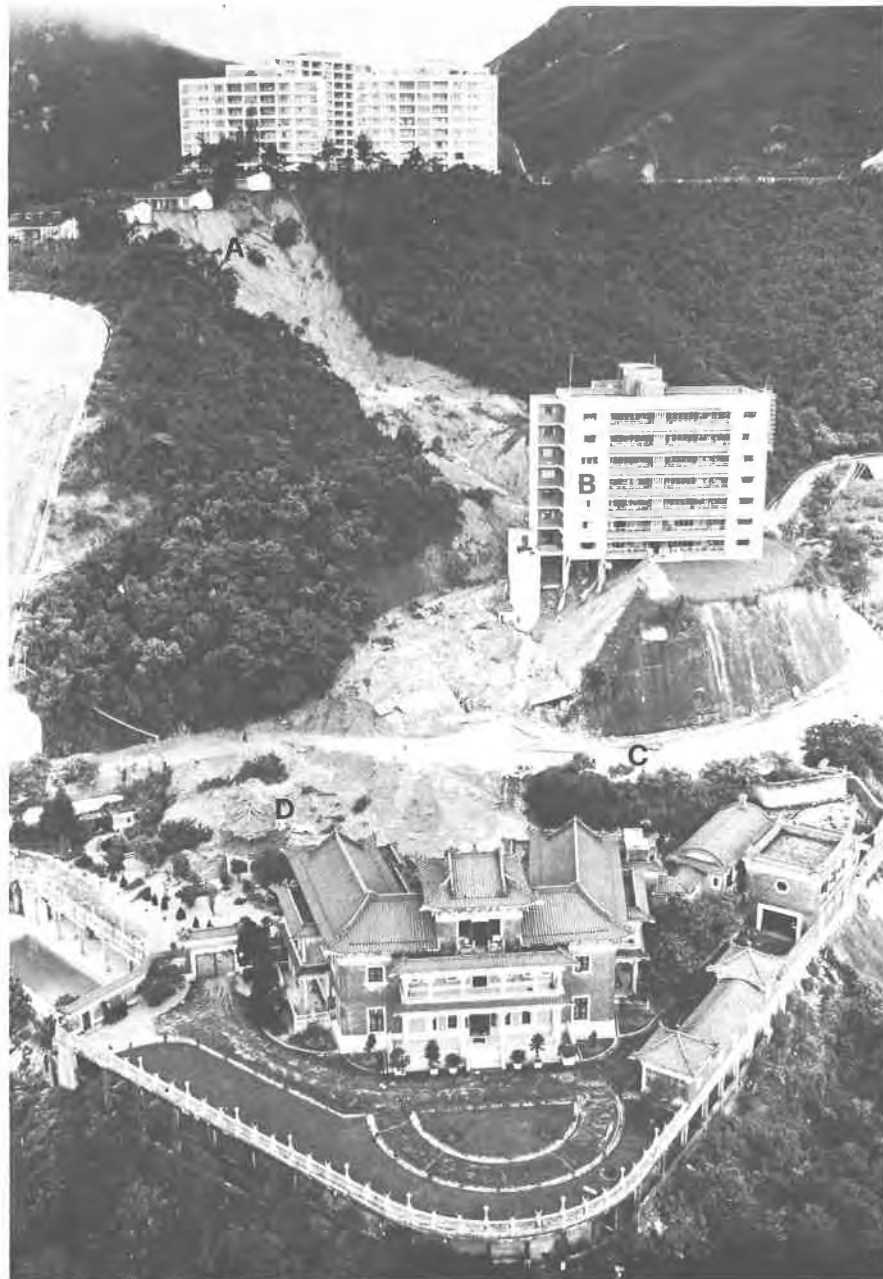
Plate 81. Landslip below Mt Nicholson Bungalows in 1966. Failure (A) of portion of a fill slope, forming part of the platform for the Mt Nicholson Bungalows, resulted in a large landslip which damaged Victoria Heights (B) and flowed across Stubbs Road (C) into a neighbouring garden (D). The Assistant Director of Education was fatally injured in the landslip. (Reproduced from Chen (1969), ISD/3982/284).
