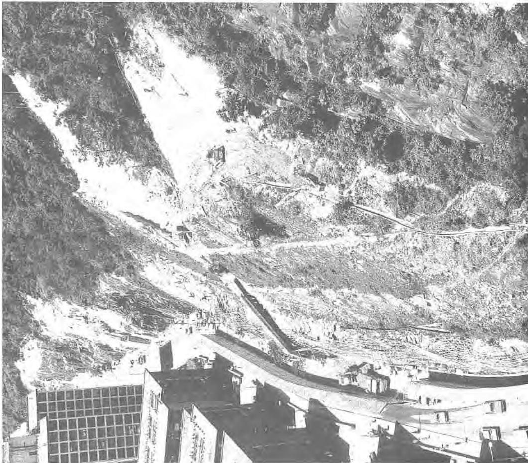
Plate 183. Slope Reconstruction at A Kung Ngam Road in June 1985. This photograph, taken on 29.6.85, shows the slope in the initial stages of remedial treatment within the Landslip Preventive Measures Programme. The rock slope shown in Plate 182 is located in the upper left hand corner of this Plate. Plate 184 shows the slope works nearing completion (Contract No. GC/84/02; Slope 11SE-B/C85 & 86).
