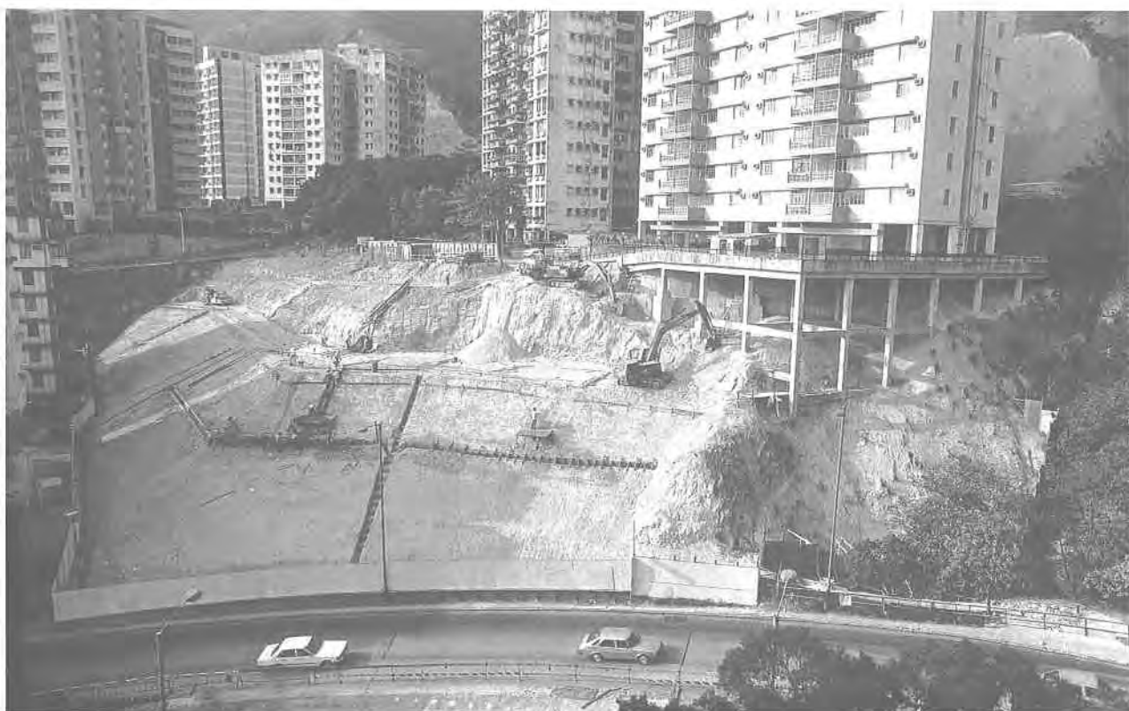
Plate 178. Stabilization Works on the Rhondda Road Slope in December 1984. This photograph, taken on 10.12.84, shows recompaction of loose fill and surface drainage works in progress. Compare this with Plates 177 and 179.
