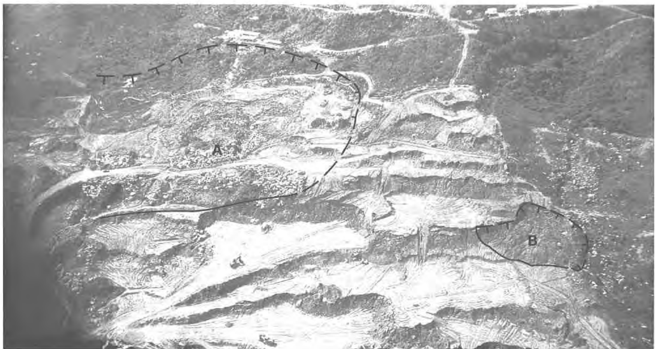
Plate 121. Oblique Aerial Photograph of Progress on Site Formation for Tuen Mun Borrow Area 19 in 1978. This photograph illustrates the state of extensive cutting of the footslope terrain in Area 19 on 28.9.1978. The general area of instability is indicated at A, whilst a smaller failure is at B. (GCO/OAP/1978/PS9-2).
