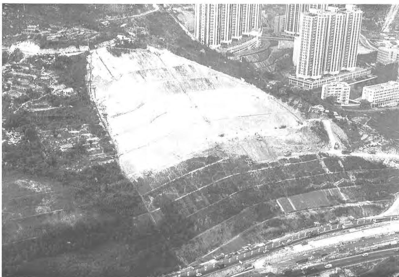
Plate 173. Oblique Aerial Photograph of Remedial Works at Pun Shan Tsuen in May 1984. The slope has been regraded and surface protection is being applied. (GCO/OAP/1984/PS448-3).
