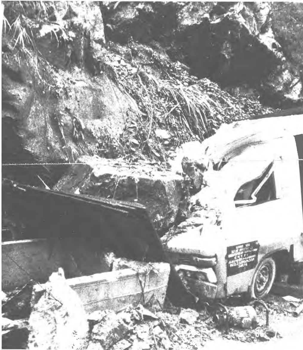
Plate 162. Rockfall at Wo Yi Hop Road in 1986. This incident occurred on a construction site at Tsuen Wan. The light goods vehicle did little damage to the boulder. (GCO/HQ/1986/HQ8603015).
