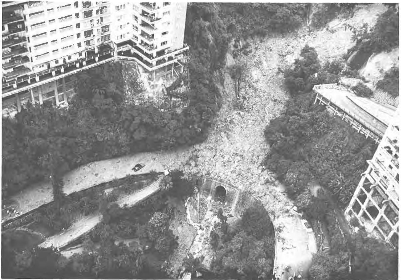
Plate 87. Landslip on Robinson Road in the Upper Glenealy Area in 1966. This was the result of the landslide near Chater Hall shown in Plate 86. (Reproduced from Chen (1969), ISD/3982/320).
