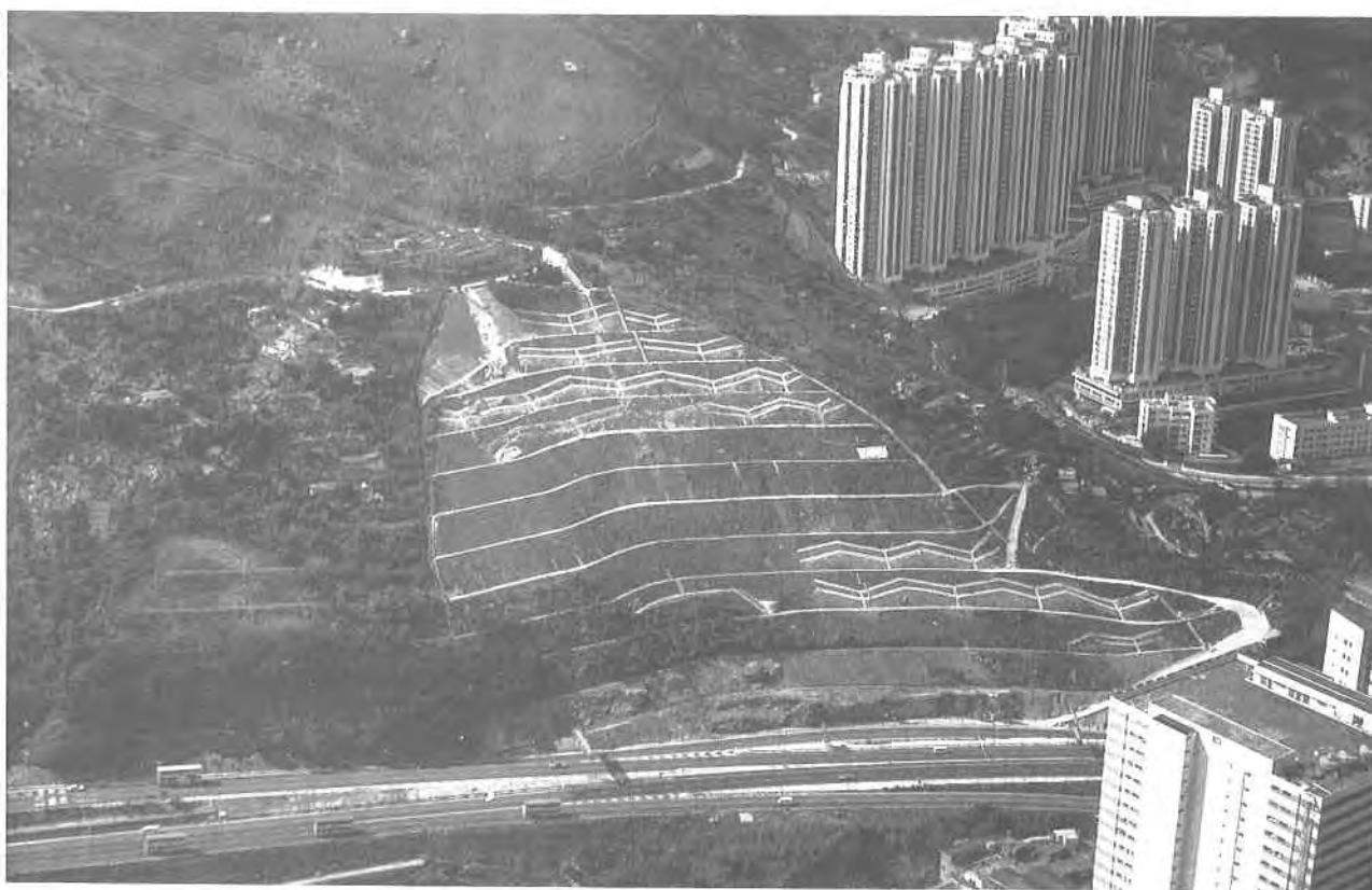
Plate 175. Oblique Aerial Photograph of Remedial Works to the Cut Slope at Pun Shan Tsuen in May 1986. Part of the upper slope has been chunamed and intensive drainage measures have been installed on the slope. Compare this with Plate 171, which shows the original cut slope in 1983. (GCO/OAP/1986/PS550-11A).
