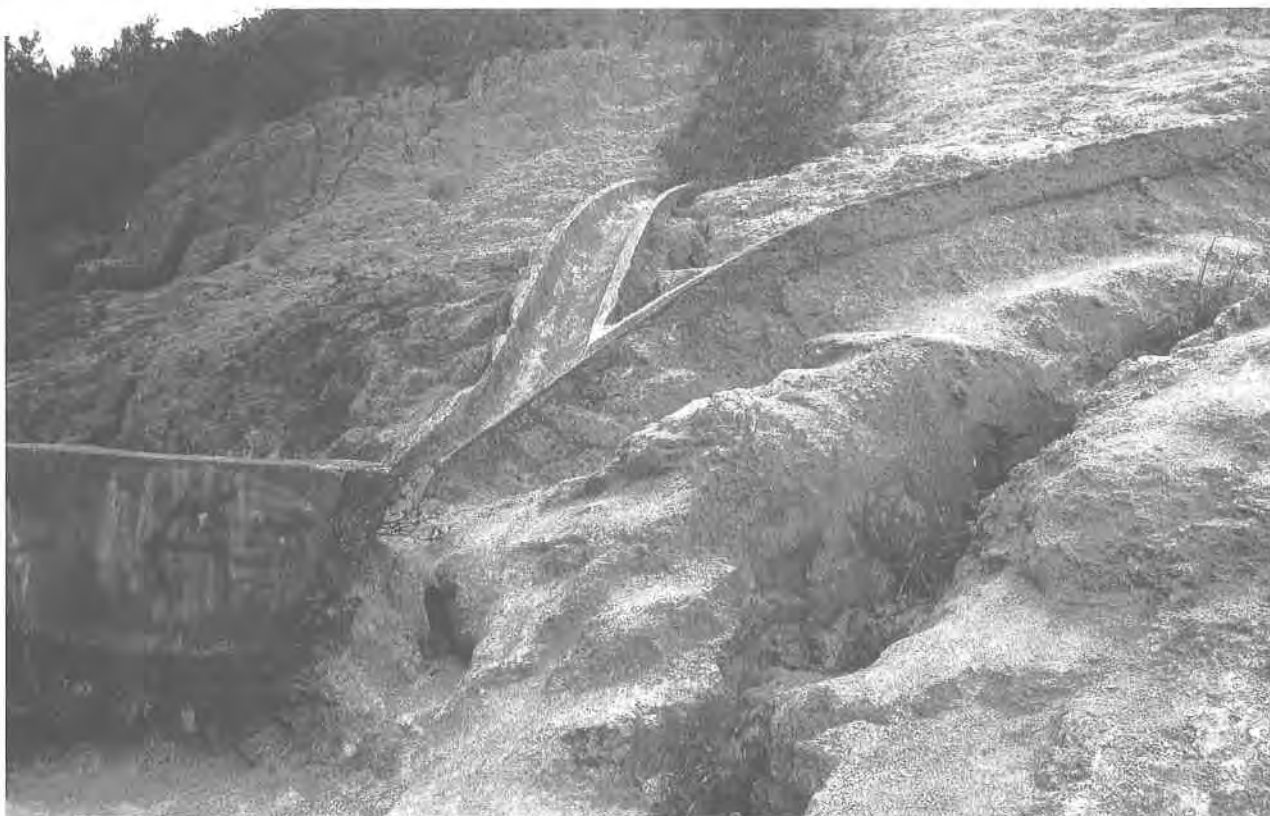
Plate 199. Severe Erosion affecting Services near Braemar Hill in 1984. Severe sheet erosion marginal to a surface drainage system is evident. Erosion has undermined the drainage channel and culvert and has rendered the drainage system essentially ineffective. (GCO/TP/1984/TP 58-22).
