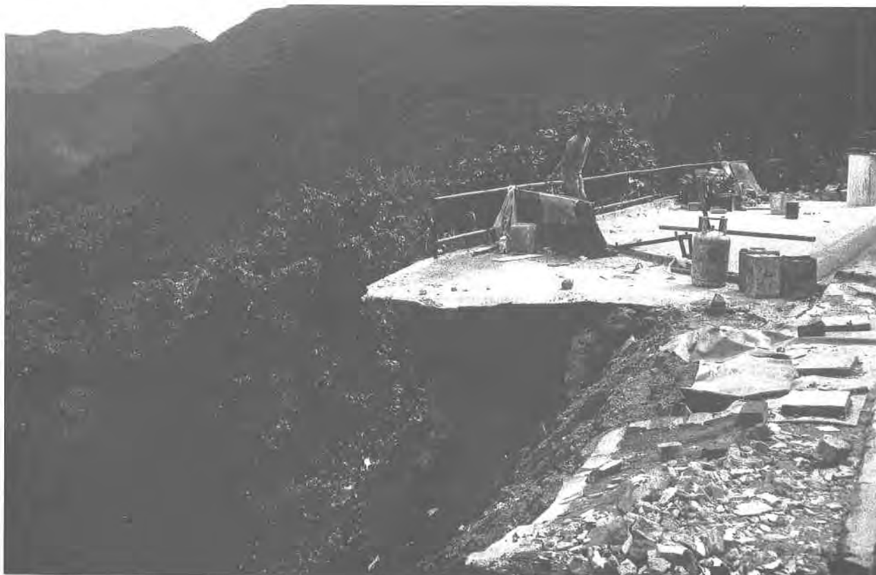
Plate 155. Landslip at Pak Tin in 1983. This failure resulted from the collapse of a 5 m high masonry retaining wall. The landslide debris blocked a Water Supplies Department access road. (GCO/1983/83/150/13).
