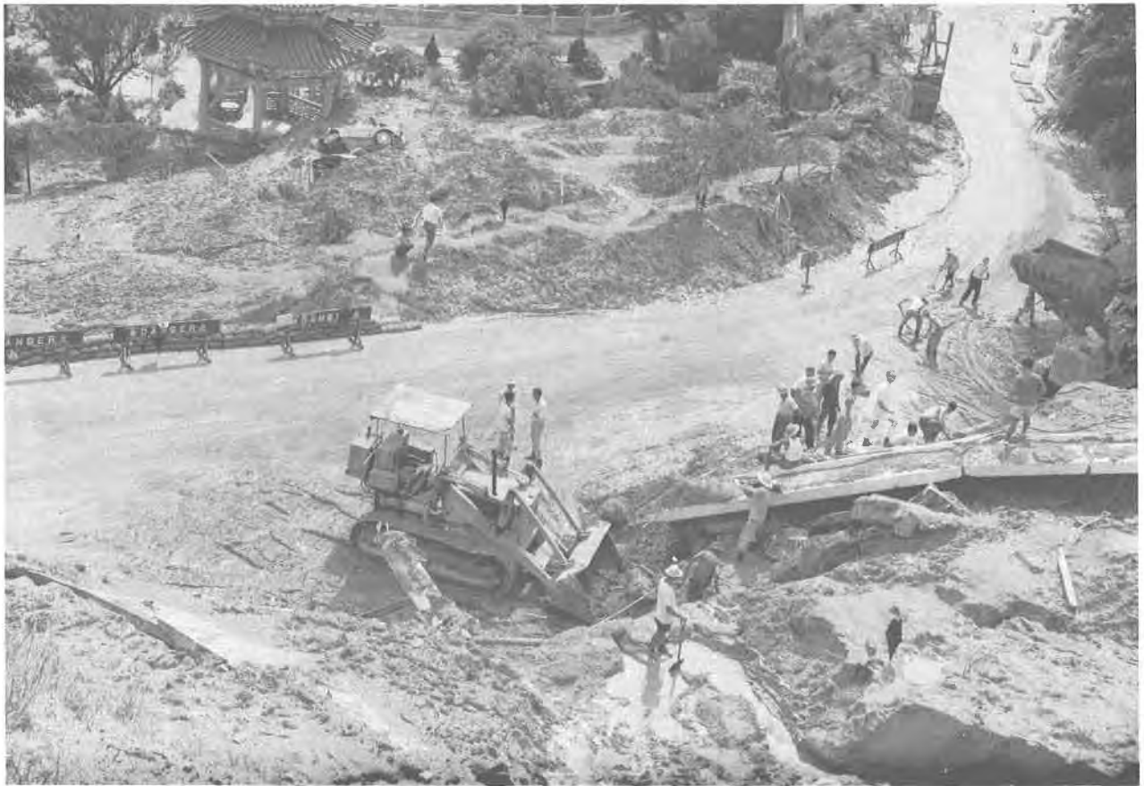
Plate 84. Clearing of Landslip Debris from Stubbs Road in 1966. Clearance work following the Mt Nicholson failure. (Reproduced from Chen (1969), ISD/3982/415).
