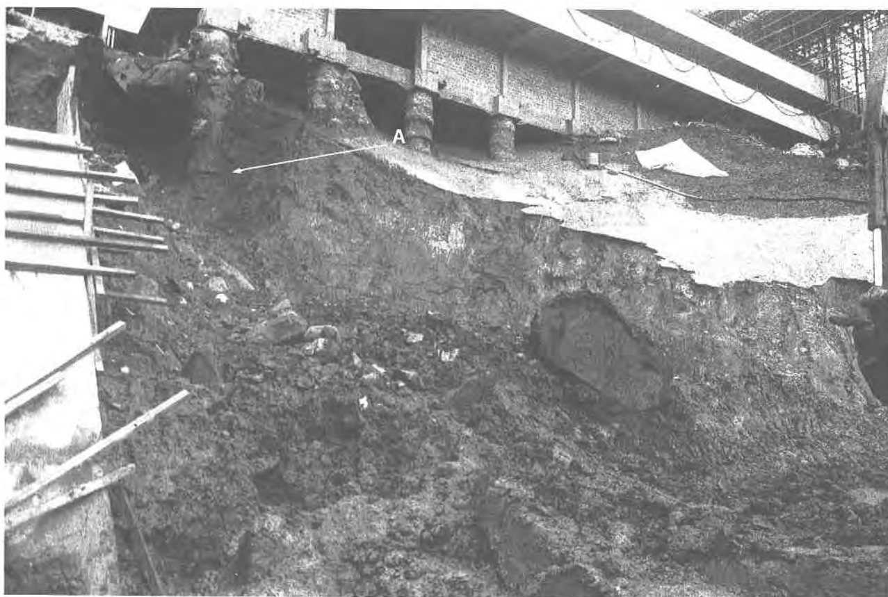
Plate 154. Landslip at Hing Man Estate in 1983. This landslide resulted from the failure of a colluvial slope beneath the car park podium of a housing estate under construction. Note the exposure of the foundations (A). Hing Man Estate is in the Chai Wan area. (GCO/1983/83/121/21).
