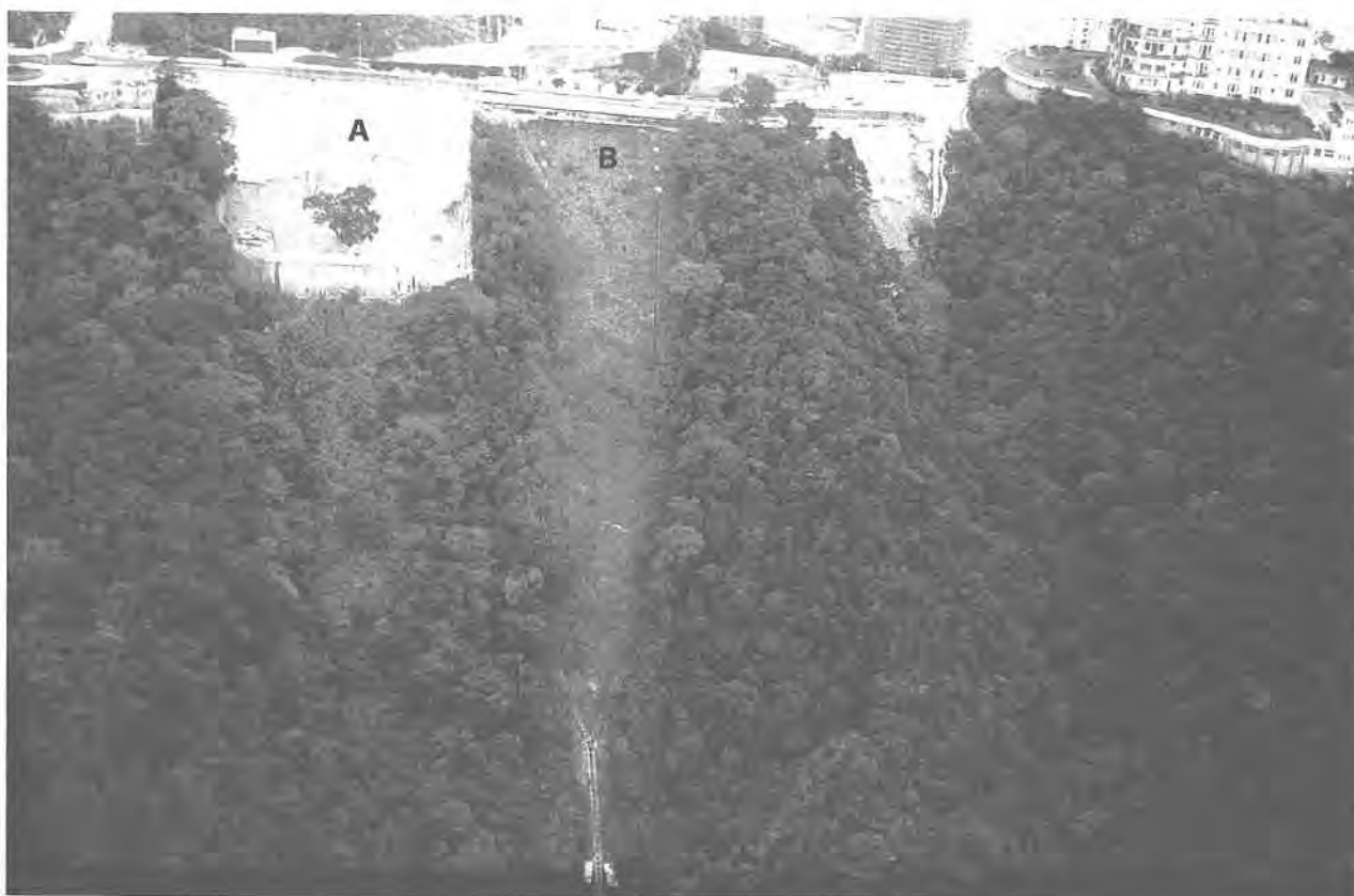
Plate 190. Oblique Aerial Photograph of Remedial Works to the Site of the 1966 Landslip on Peak Road. This photograph was taken in 1987, and shows remedial works to the site of a landslide in 1966 (A) shown in Plate 58 and also Plate 153. Remedial works were carried out on the old landslide site following a very disruptive failure nearby in 1983. The location of the failure is shown at B in this Plate and in Plate 57. (GCO/OAP/1987/PS607-18).
