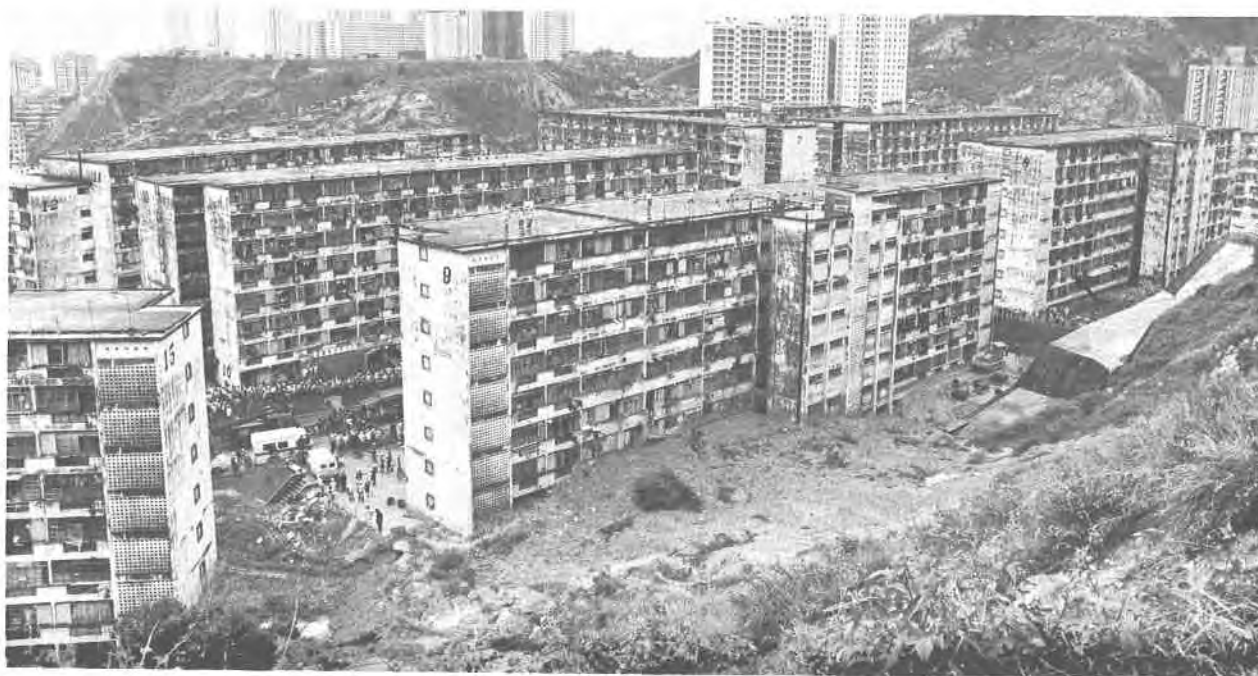
Plate 111. Landslip at Sau Mau Ping in 1976. Some four years after the 1972 landslip (Plates 107 to 109), a further three landslips occurred on the fill slopes above Sau Lai Street. The embankment adjoining Block 9, Sau Mau Ping Estate collapsed at 10.12 a.m. on 25.8.1976. The landslip debris buried most of the ground floor of the residential estate building below the slope. As a result, there were 18 killed and 24 injured. This landslip occurred following intense rainfall on 25–26.8.1976. The Royal Observatory recorded more than 545 mm of rainfall in the 2 day period. The failure was very similar to the 1972 Sau Mau Ping landslip, involving the 'liquefaction' of uncompacted fill. The location of Block 9 in relation to the 1972 landslip is shown in Plate 107. Plates 55 and 56, taken at the time of site formation, provide an interesting comparison with the location of the 1972 and 1976 failures highlighted in Plate 115. (ISD/25.8.1976/ 14949/76).
