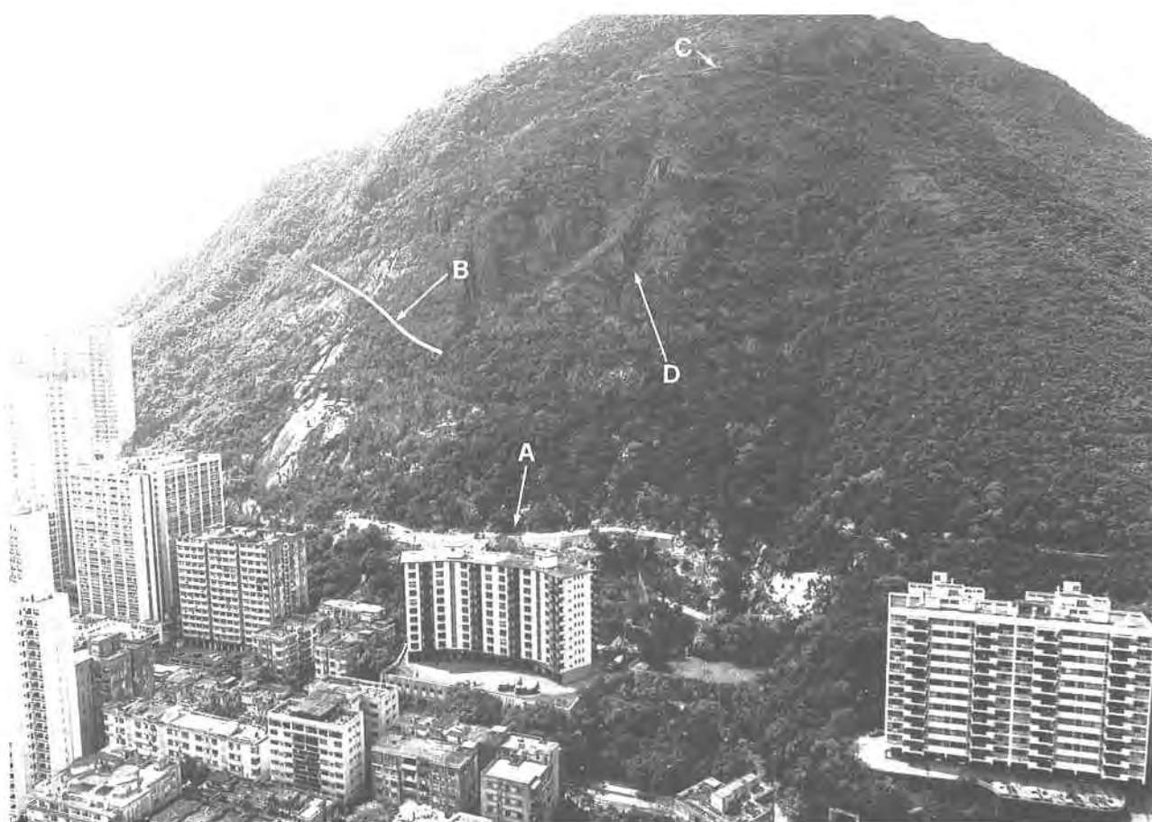
Plate 168. Oblique Aerial Photograph of Boulder Field Stabilization Measures on the Upper Slopes of Victoria Peak in 1985. This photograph taken in 1985, shows the location of the 'Boulder Fence' (A), upslope of Buxey Lodge. The Fence is located on an extensive boulder field, and was designed by GCO to counter the effects of possible rock and boulder falls from the steep colluvial footslopes and the precipitous cliffs on the north side of Victoria Peak. The geological contact between the volcanics and granitic bedrock is indicated at B. Lugard Road is indicated at C, and the general location of the rock outcrop shown in Plate 170 is shown at D. The natural slope above Conduit Road overlooks an area of intense development and has suffered from a number of boulder falls. In 1926, a 700-tonne boulder fell on a pumping station at 3 Conduit Road. In 1957, a boulder crushed a car parked on Conduit Road. In 1961, a 40-tonne boulder fell onto the west lawn of Buxey Lodge. More recently, incidents have been reported behind Pearl Gardens (1978), Conway Mansion (1979), Buxey Lodge (1981, 1982 and 1985), 39 Conduit Road (1981) and 41C Conduit Road (1982). The boulder field is located on the natural hillside behind 17 (Cliffview Mansion) to 37 (Buxey Lodge) Conduit Road. It is some 300m wide in an E-W direction and extends from the rear of the buildings (150mPD) southwards to the toe of Seymour Cliffs (280mPD). The total area is about 4.5 ha. (GCO/OAP/1985/PS514-5).
