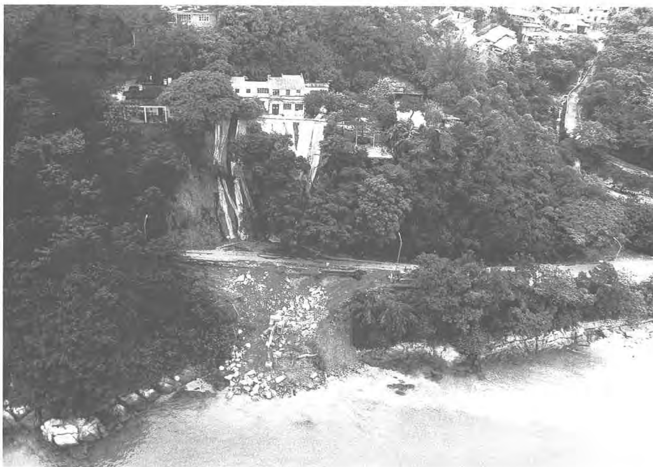
Plate 144. Oblique Aerial Photograph of Landslips on Castle Peak Road in 1982. During heavy rain on 29.5.82, a number of failures occurred in the vicinity of Lai Shum Villa off Castle Peak Road. These included three minor cut slope failures behind the Villa, one larger cut slope failure on Castle Peak Road, the subsidence of a 30 m by 30 m wide section of Castle Peak Road due to failure of a fill embankment, and the failure of the edge of a fill platform associated with the cracking of a masonry retaining wall. The interesting aspect of the Lai Shum Villa incidents is that six failures occurred in a very small area, on both cut and fill slopes. This could be attributed to extremely intense local rainfall, perhaps for only a few minutes during the storm. (GCO/OAP/1982/PS272-23).
