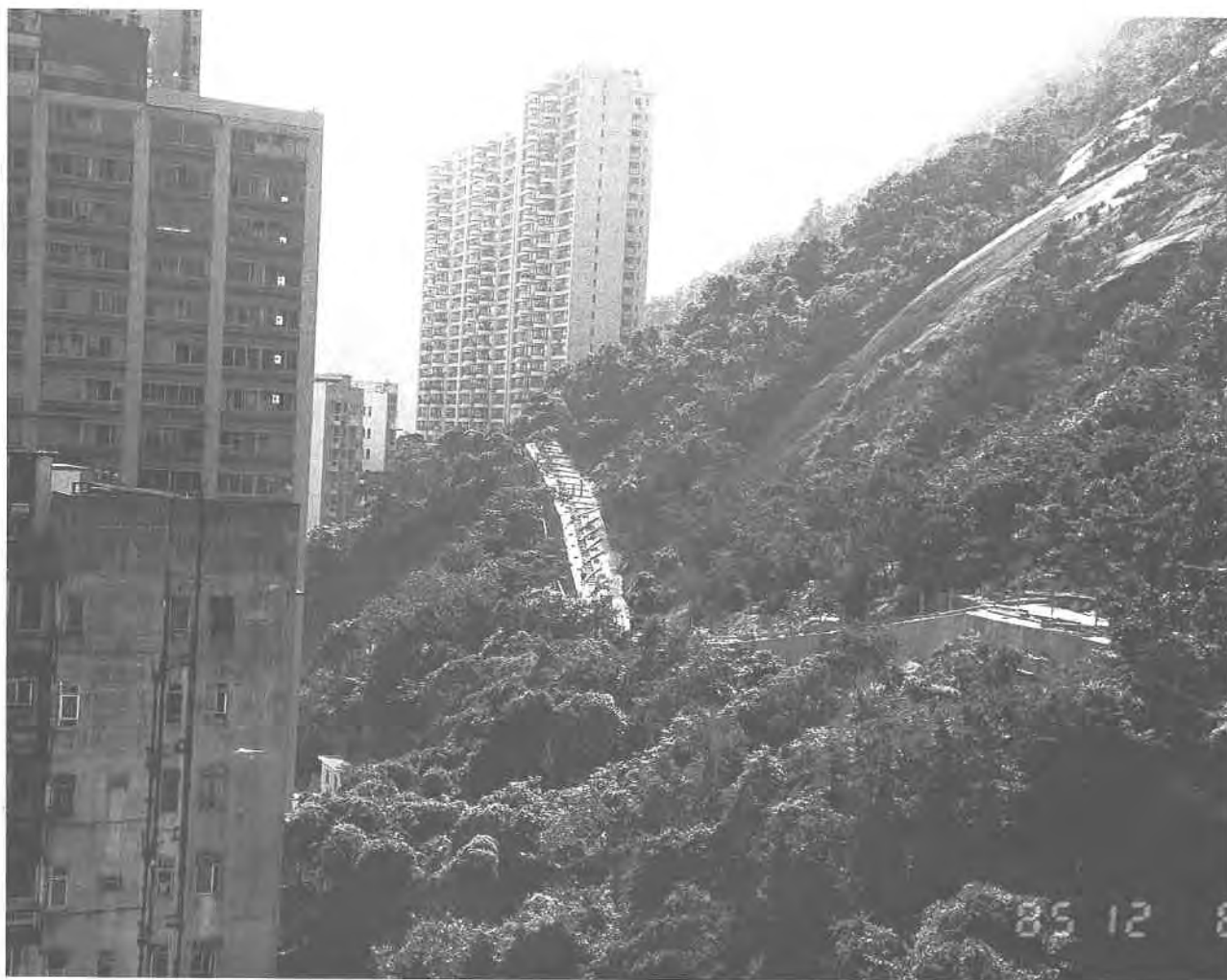
Plate 169. Boulder Fence below Victoria Peak in 1984. This photograph, taken from Buxey Lodge on 6.12.85, shows Segments 6 and 7 of the Fence under construction. These works were carried out within the Landslip Preventive Measures Programme. Construction of the Fence and associated boulder stabilization works cost in the order of $7.5m over a 2-year period. (Contract 1/GCO/93).
