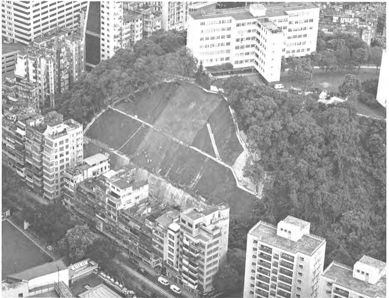
Plate 189. Oblique Aerial Photograph of Slope Stabilization at Leighton Hill in 1987. This slope has a history of failure and was reconstructed by the Geotechnical Control Office over an 18-month period between July 1986 and February 1988. Works in the order of $3.2 million were carried out within the Landslip Preventive Measures Programme. On this occasion, the design required that the finished slope be vegetated rather than chunamed. Geotextiles were used extensively during reinstatement. (GCO/OAP/1987/PS603-6).
