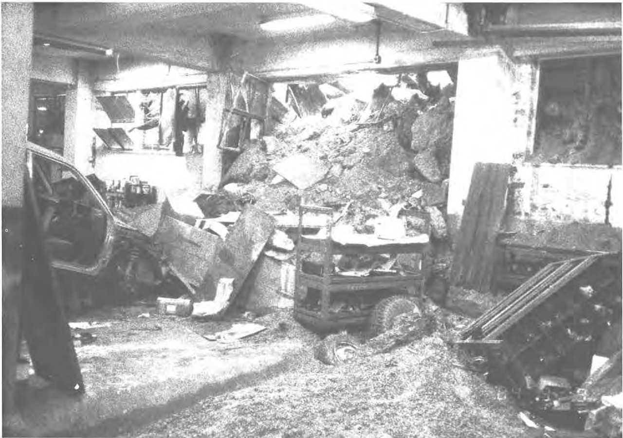
Plate 158. Damage to Workshop at Tsat Tsz Mui Road in 1984. Failure of the cut slope, shown in Plate 157, resulted in damage to a workshop on the ground floor. (GCO/IE/1984/IE111/84/6A).
