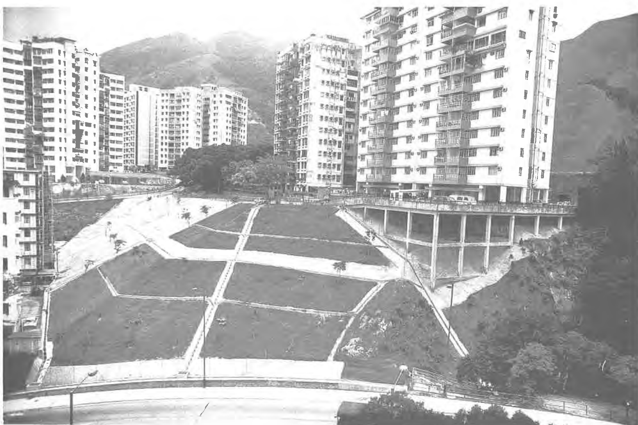
Plate 179. Stabilization Works on the Rhondda Road Slope in July 1985. This photograph, taken on 12.7.85, shows a general view following reinstatement of the slope at a cost of some $1.3m over a 12-month period. Compare this with Plates 177 and 178.
