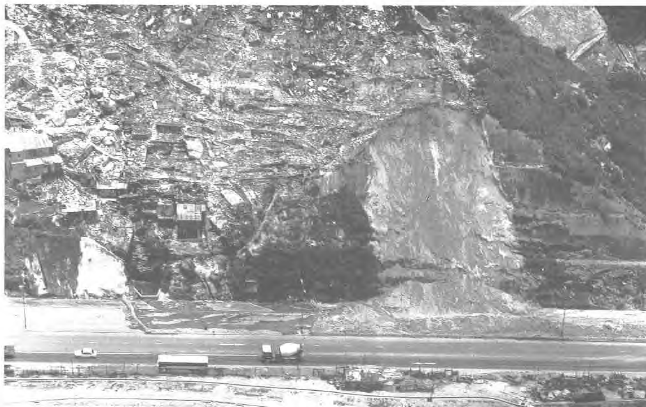
Plate 148. Oblique Aerial Photograph of Landslip near a Squatter Area at Lam Tin in 1982. A large cut slope failure occurred on Junk Bay Road near the location of the landslip in Plate 147. The general area had been cleared of squatters at the time due to a fire earlier in the year. Some details of the slope failure are presented in Plate 149. (GCO/OAP/1982/PS297-5A).
