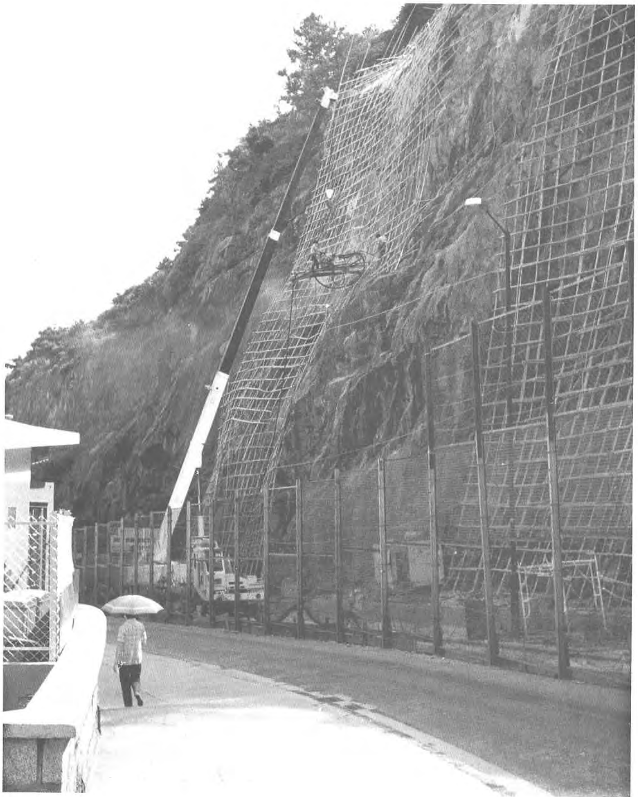
Plate 182. Remedial Works on Rock Slope at A Kung Ngam Road in July 1983. This photograph, taken on 25.7.83, shows the drilling of a raking drain. This slope was treated within the Landslip Preventive Measures at an approximate cost of $1.7m over an 18-month period. (3/GCO/82 & 5/GCO/83 Slope 11SE-B/C87).
