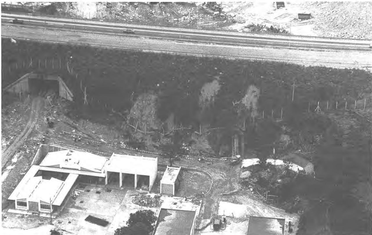
Plate 143. Oblique Aerial Photograph of Landslips on a Road Embankment near Cafeteria Beach in 1982. Although these are relatively small failures, this type of incident has considerable impact in terms of maintenance costs for reinstatement and clearance of blocked access and drainage systems. (GCO/OAP/1982/PS275-5A).
