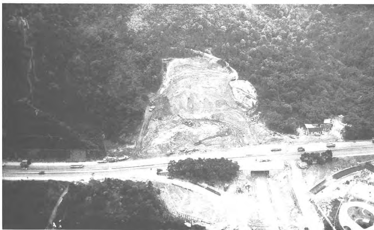
Plate 134. Oblique Aerial Photograph of Remedial Works to Landslip Site near World Wide Gardens in Sha Tin in 1979. This photograph, taken in 1979, shows remedial works on the site of a landslide which occurred during Severe Tropical Storm Agnes in July 1978. (GCO/OAP/1979/PS19-12).
