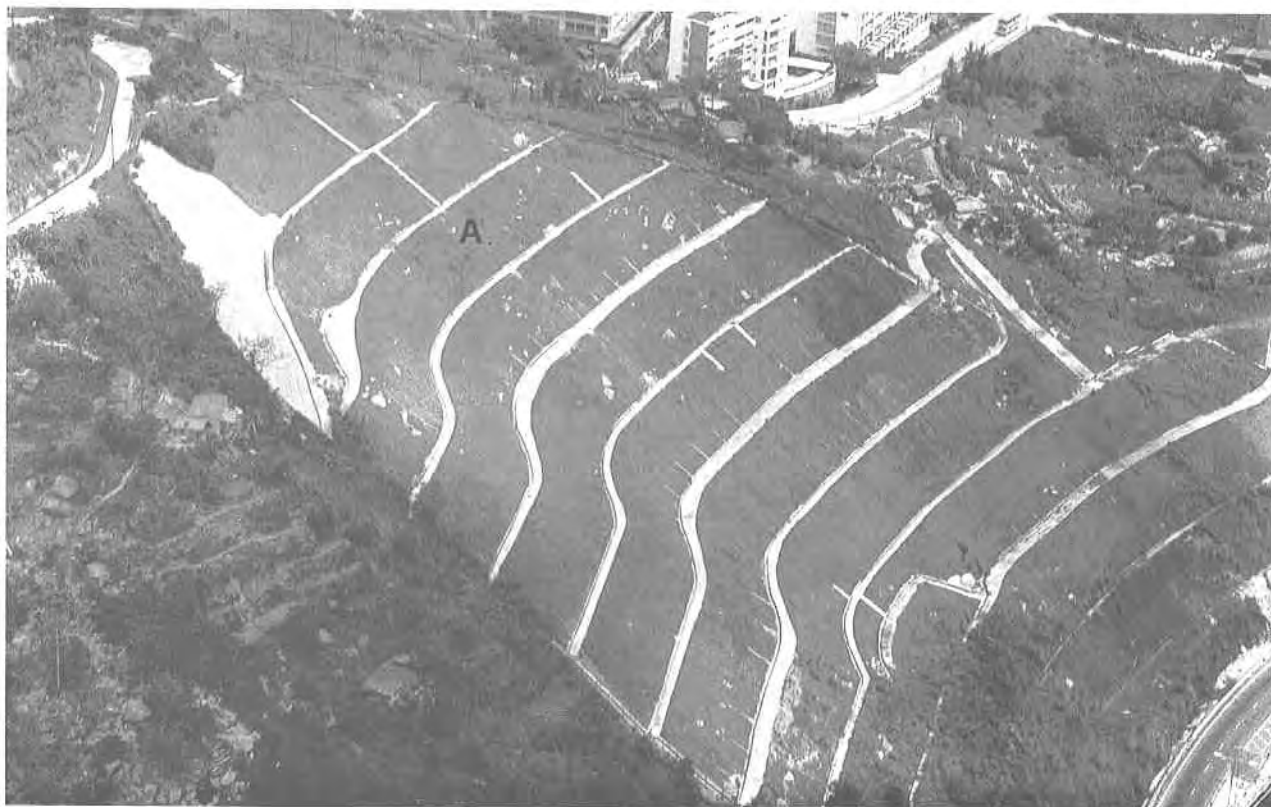
Plate 174. Oblique Aerial Photograph of Reinstated Cut Slope at Pun Shan Tsuen in September 1985. The slope has been regraded and has an extensive cover of vegetation. Soil piping, tunnel erosion and associated surface erosion are evident around A. (GCO/OAP/1985/PS523-10).
