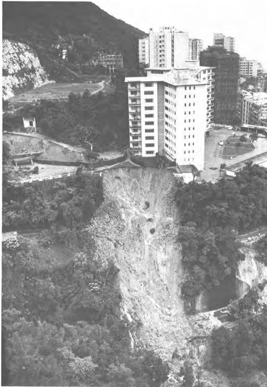
Plate 86. Landslip near Chater Hall in 1966. A section of May Road (Hornsey Road) was destroyed by this landslide, Plate 87 reveals the effects of the debris on the downslope terrain. A newspaper report at the time noted that the residents of Chater Hall were being accommodated at the Mandarin and Hilton Hotels 'at special rates'. (Reproduced from Chen (1969), ISD/3982/8).
