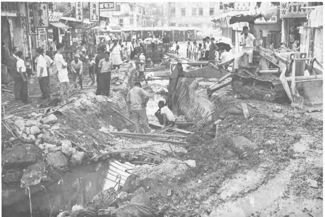
Plate 71. Damage to Drainage Culvert in Stone Nullah Lane in 1966. The concrete road slabs were washed away by floodwaters. (Reproduced from Chen (1969), ISD/3982/426).
