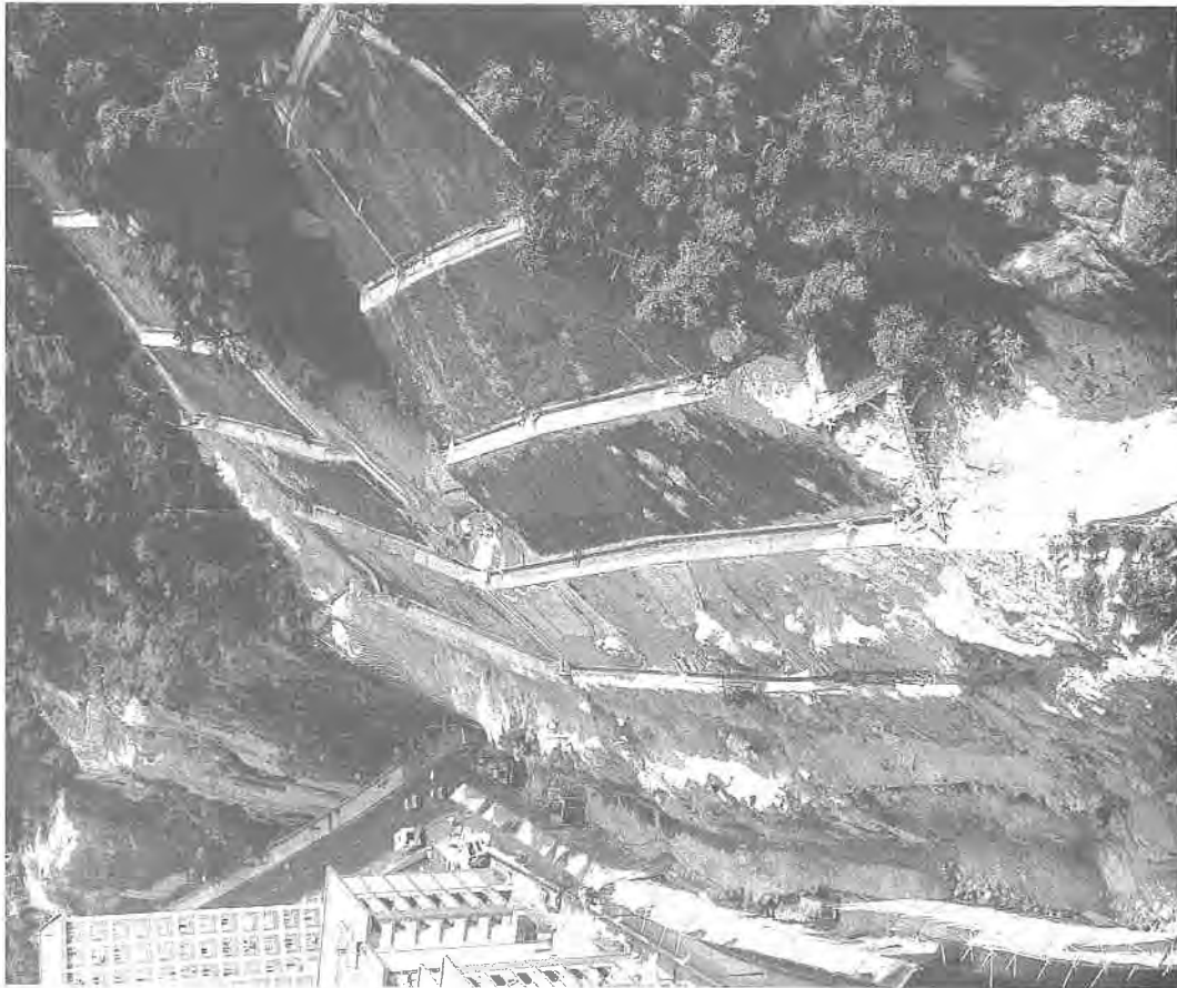
Plate 184. Slope Reconstruction at A Kung Ngam Road in December 1985. This photograph, taken on 2.12.85, shows the final stages of slope reconstruction. The approximate cost was $2.6 m over a 12-month period. Horizontal drains are in place on the upper portion of the slope. Compare this with Plate 183. (Contract No. GC/84/02; Slopes 11SE-B/C85 & 86).
