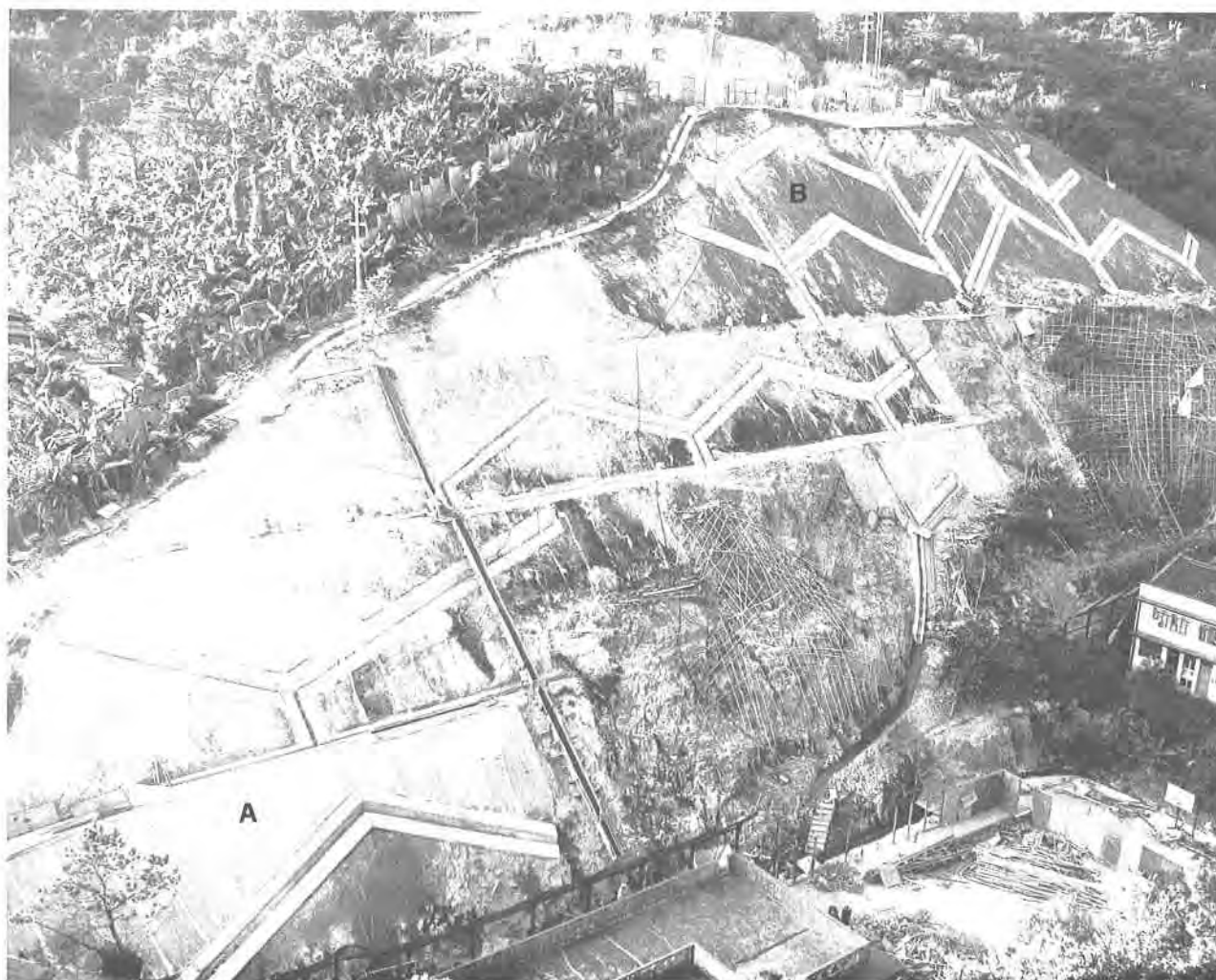
Plate 186. Slope Stabilization at Chung Kwai Chung in October 1986. This photograph, taken on 31.10.86, shows the slope in the final stages of reconstruction. Total expenditure on slope works was in the order of $1.3m over a period of 14 months. Surface drainage is in place and netting is evident on many of the lower berms (A). Hydroseeding is applied to the netting, which becomes covered as the grass becomes established (B). Compare this with Plate 185. (Contract No. GC/84/02; Slope 7SW-C/C259/14).
