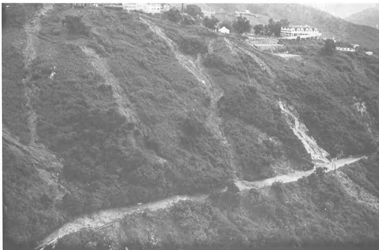
Plate 79. Oblique Aerial Photograph of Landslips above Victoria Road in Pok Fu Lam in 1966. It was reported that a total of 29 landslips and 18 washouts occurred along Victoria Road during the period of storm activity following 10.6.1966. (Reproduced from Chen (1969), ISD/3982/382).
