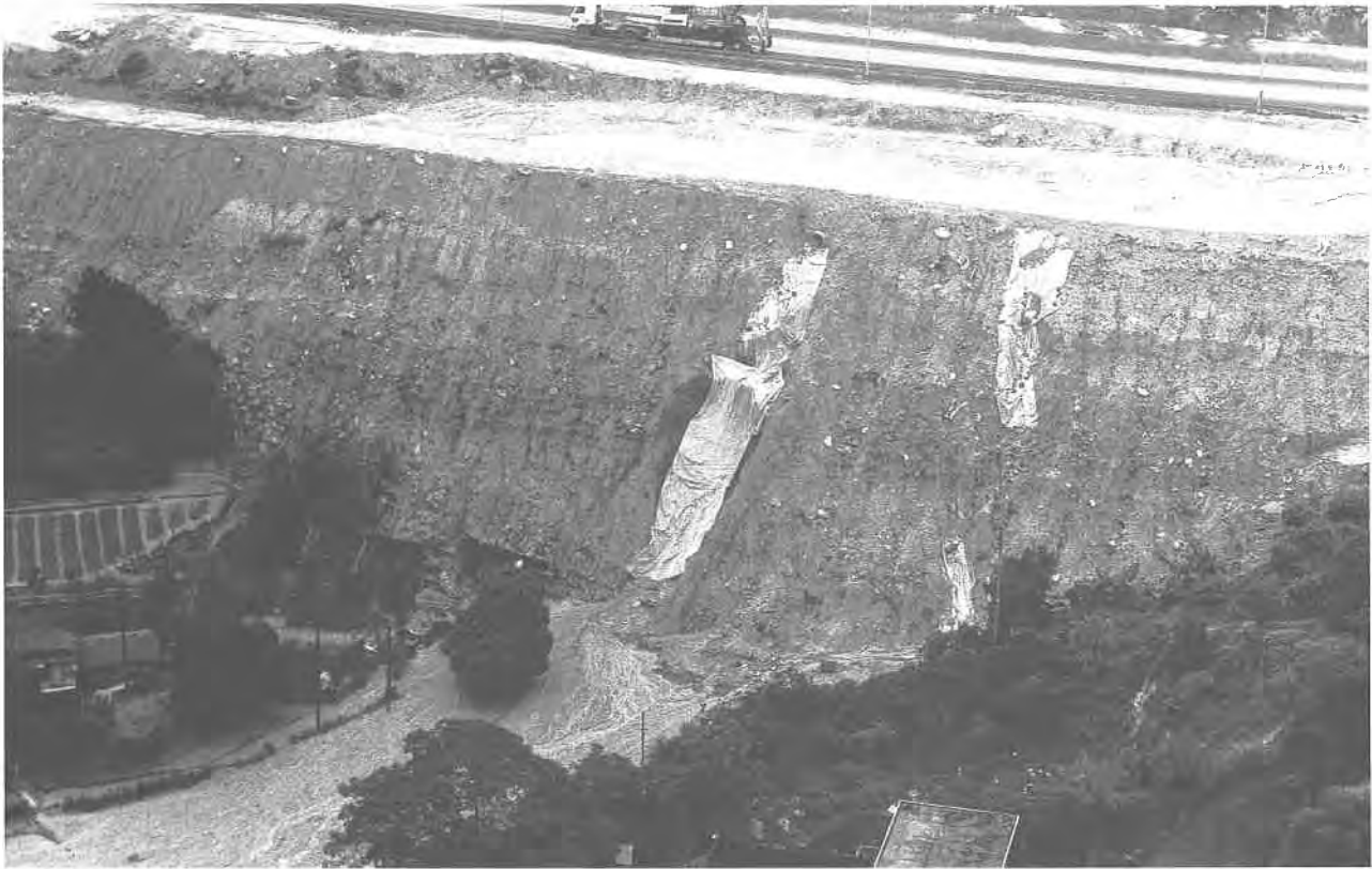
Plate 142. Oblique Aerial Photograph of Erosion on a Fill Slope near Siu Lam San Tsuen in 1982. Severe erosion is evident on the road embankment, and a large area of sediment is apparent. (GCO/OAP/1982/PS275-12A).
