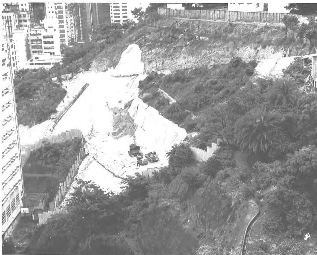
Plate 187. Slope Reconstruction at King's Park in August 1986. This photograph, taken on 24.8.86, shows the initial stages of reconstruction of the slope within the Landslip Preventive Measures Programme. Plate 188 shows the slope works nearing completion. (Contract No. GC/84/03; Slope 11SW-D/F97).
