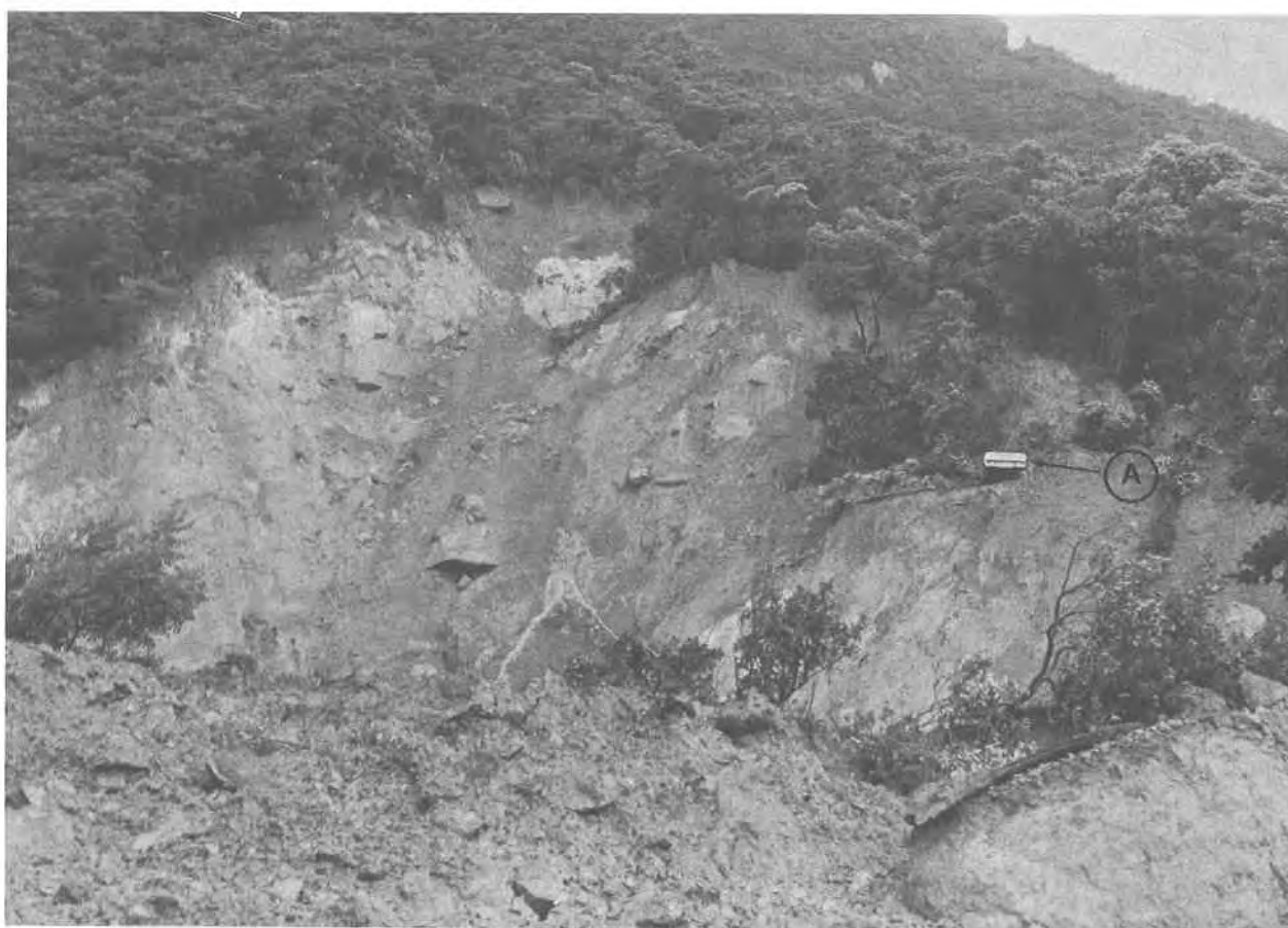
Plate 95. Backscar of the Po Shan Road Landslip in 1972. Part of a vehicle is evident (A). This vehicle was probably parked on Po Shan Road at the time of the landslip, but has come to rest some 5m below the level of the road. (19.6.1972/ISD/8257/1).
