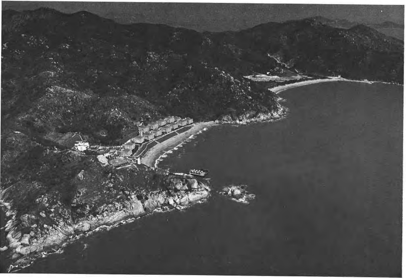
Plate 4. Oblique Aerial Photograph of the Southern Chi Ma Wan Peninsula. Note that many boulders on the sideslopes may pose a hazard to development downslope. (GCO/OAP 1984/11013).
