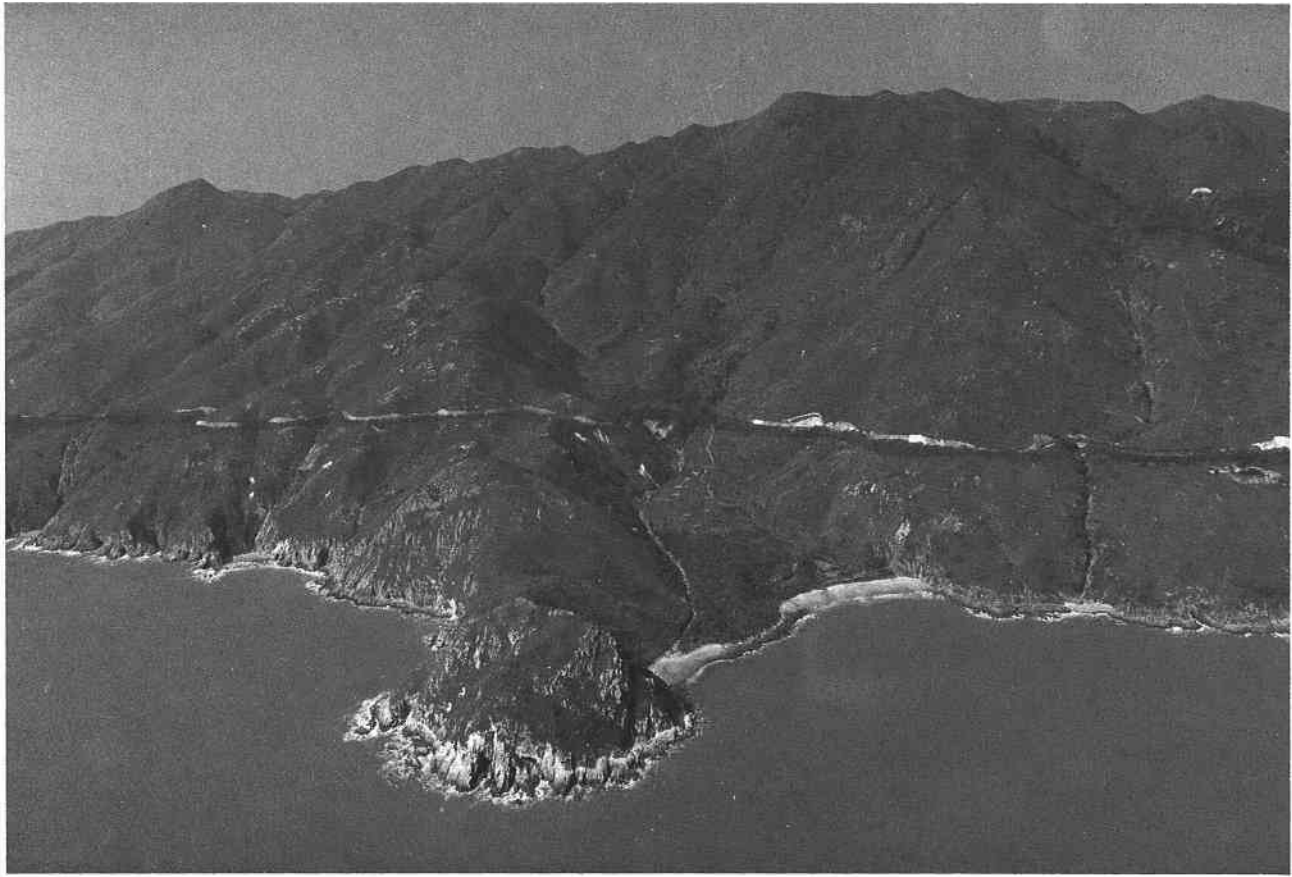
Plate 18. Oblique Aerial Photograph of the Southeastern Slopes of Ling Wui Shan. Landslips in the centre of this Plate are shown in greater detail in Plate 32. (GCO/OAP 1984/11031).
