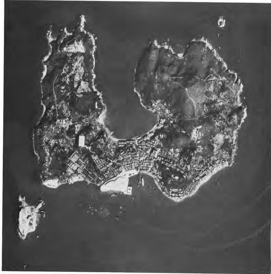
1983: Reclamation is evident on the western side of the island to the north of the ferry pier. A fixed crossing to Tai Lei is under construction. (1983/51348)
