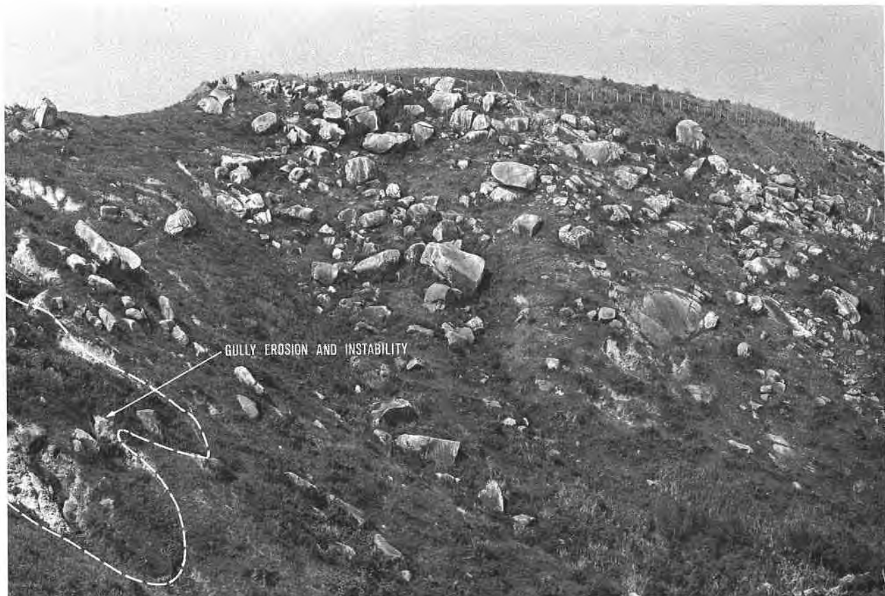
Plate 19. Boulder-strewn Slope on Cheung Chau Granite. Corestones, exposed by erosion of deeply weathered granite, litter this slope on northern Cheung Chau. The top of the slope, which has been cut to form a platform, formerly housed a radar station. Instability resulting from gully erosion in the weathered profile is evident in the left foreground. (GCO/TP 1984/52-84).
